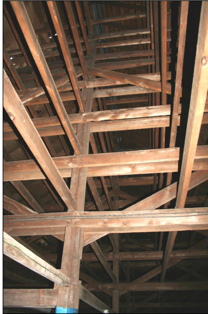
Photograph 72: Barn G (103), interior framing, looking upward toward ridge vent.
