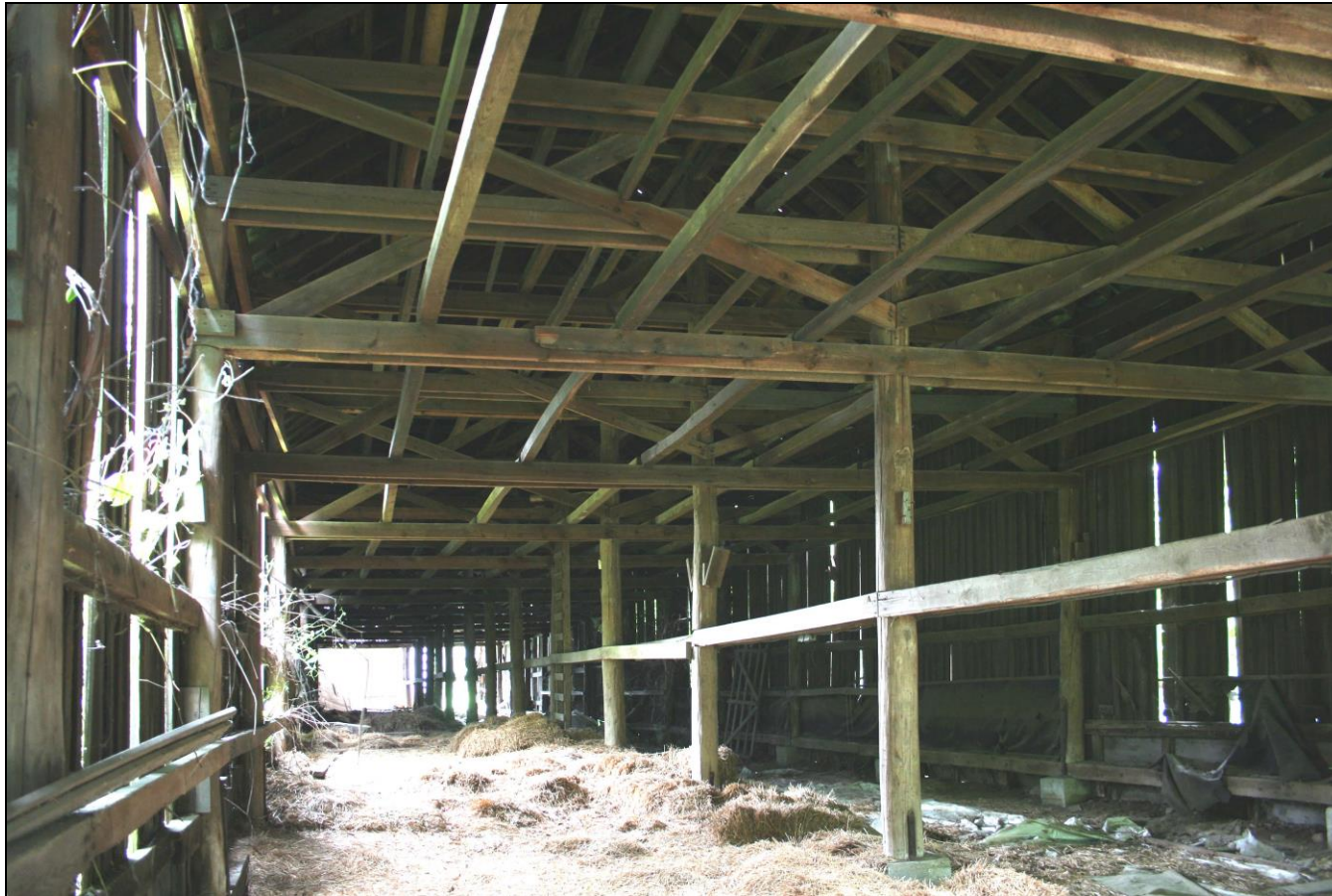
Photograph 14: Overview of the interior of Barn A (2-18/18), from the north end.
