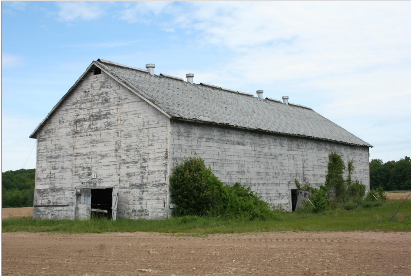
Photograph 59: Barn F (9), south and east elevations, camera facing northwest.
