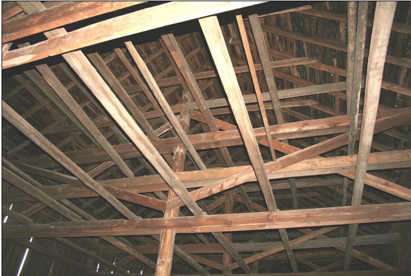
Photograph 17: Detail of transverse cross-bracing, Barn A (2-18/18).
