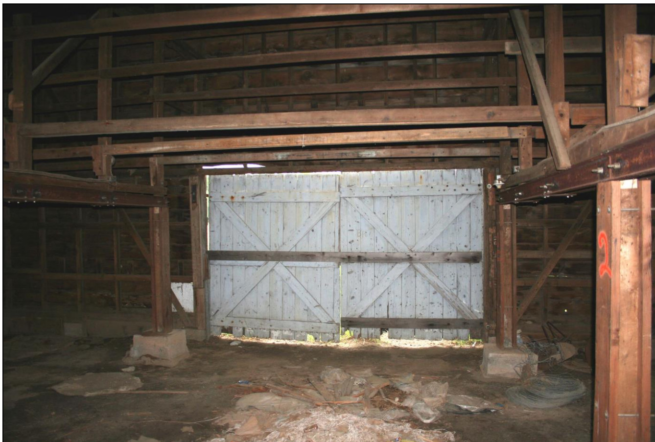
Photograph 135: Barn N (2-16), interior, detail of inside of south end doors.
