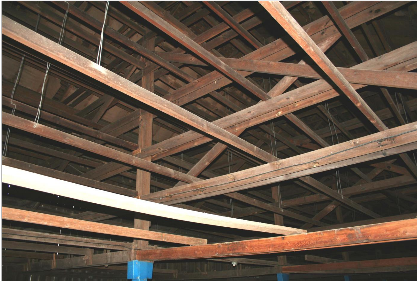
Photograph 81: Barn H (104), interior, detail of cross-bracing.
