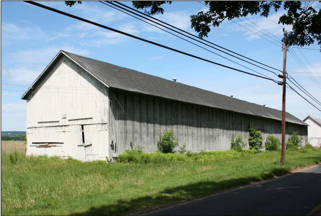
Photograph 20: Barn B (19), south and east elevations, camera facing northwest.
