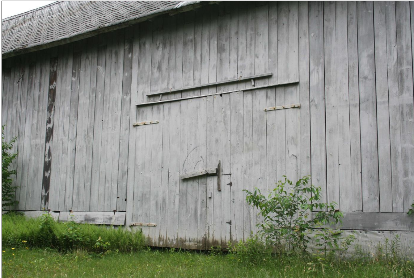
Photograph 33: Barn C (20), detail of door, east side, camera facing southwest.
