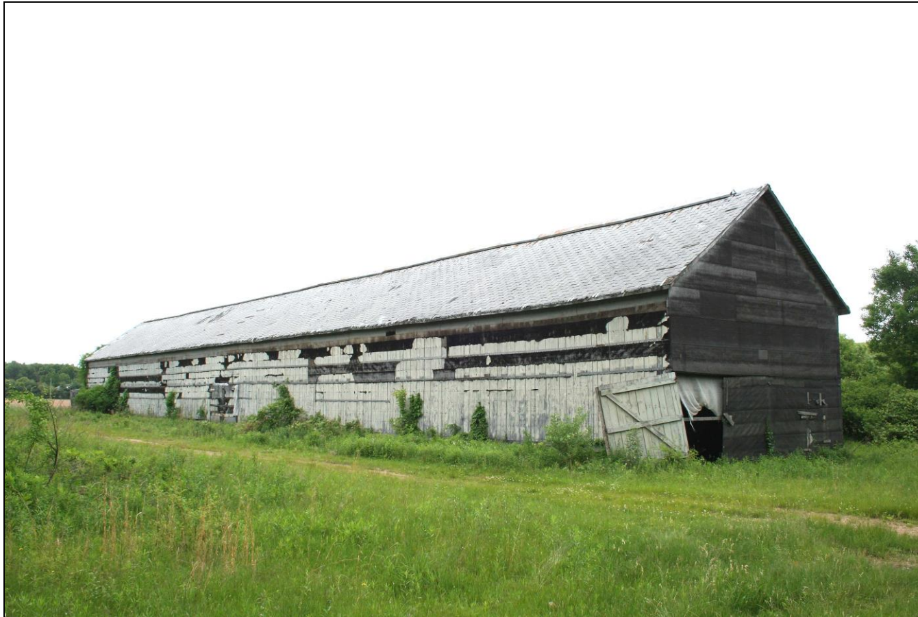
Photograph 77: Barn H (104), east and north elevations, camera facing southwest.
