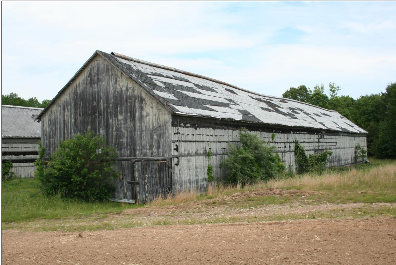
Photograph 68: Barn G (103), south and east elevations, camera facing northwest.
