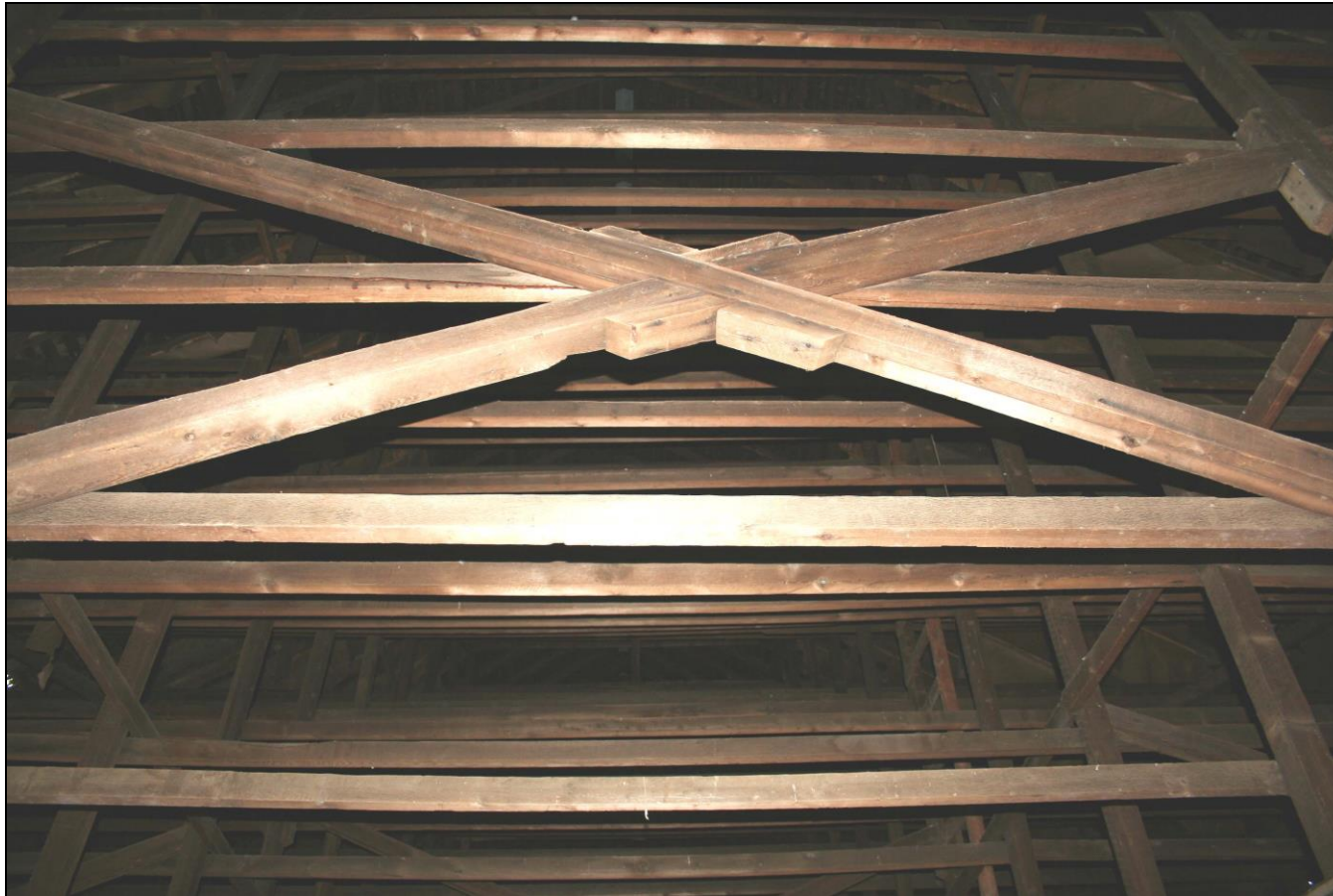
Photograph 65: Barn F (9), interior, detail of center cross-bracing.
