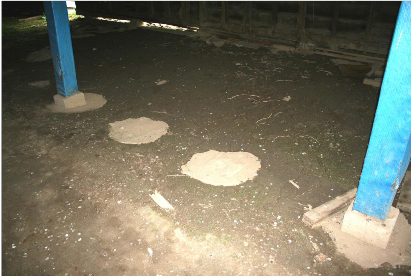
Photograph 64: Barn F (9), interior, showing remnants of footings for intermediate posts.
