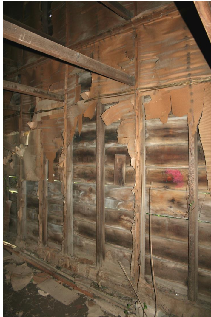
Photograph 62: Barn F (9), interior, detail of balloon-framed wall.
