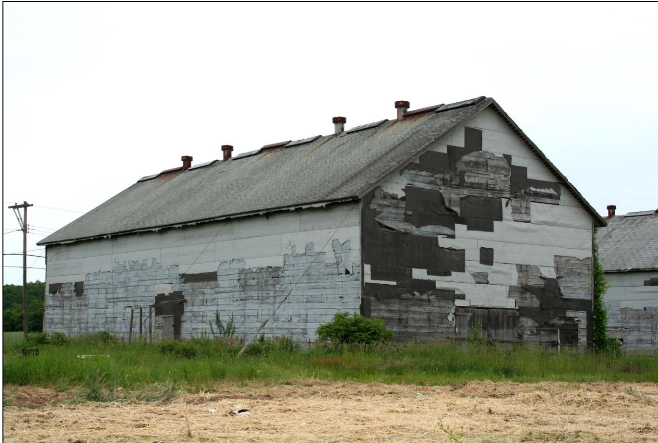
Photograph 106: Barn K (2-13), west and south elevations, camera facing northeast.
