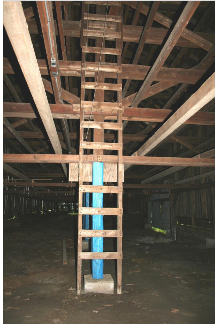
Photograph 29: Barn B (19), interior, detail of ladder leading into tiers.
