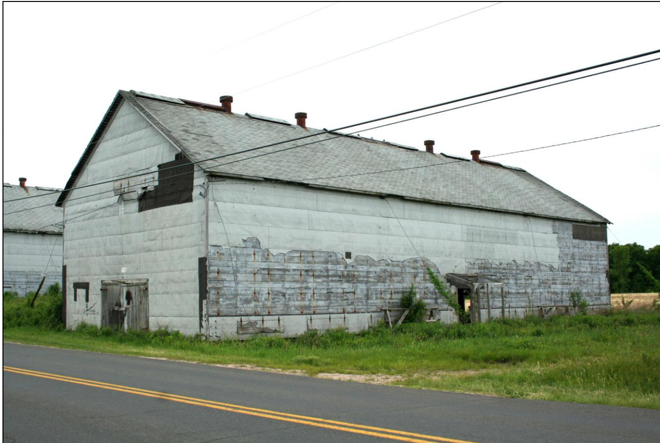
Photograph 120: Barn M (2-15), north and west elevations, camera facing southeast.
