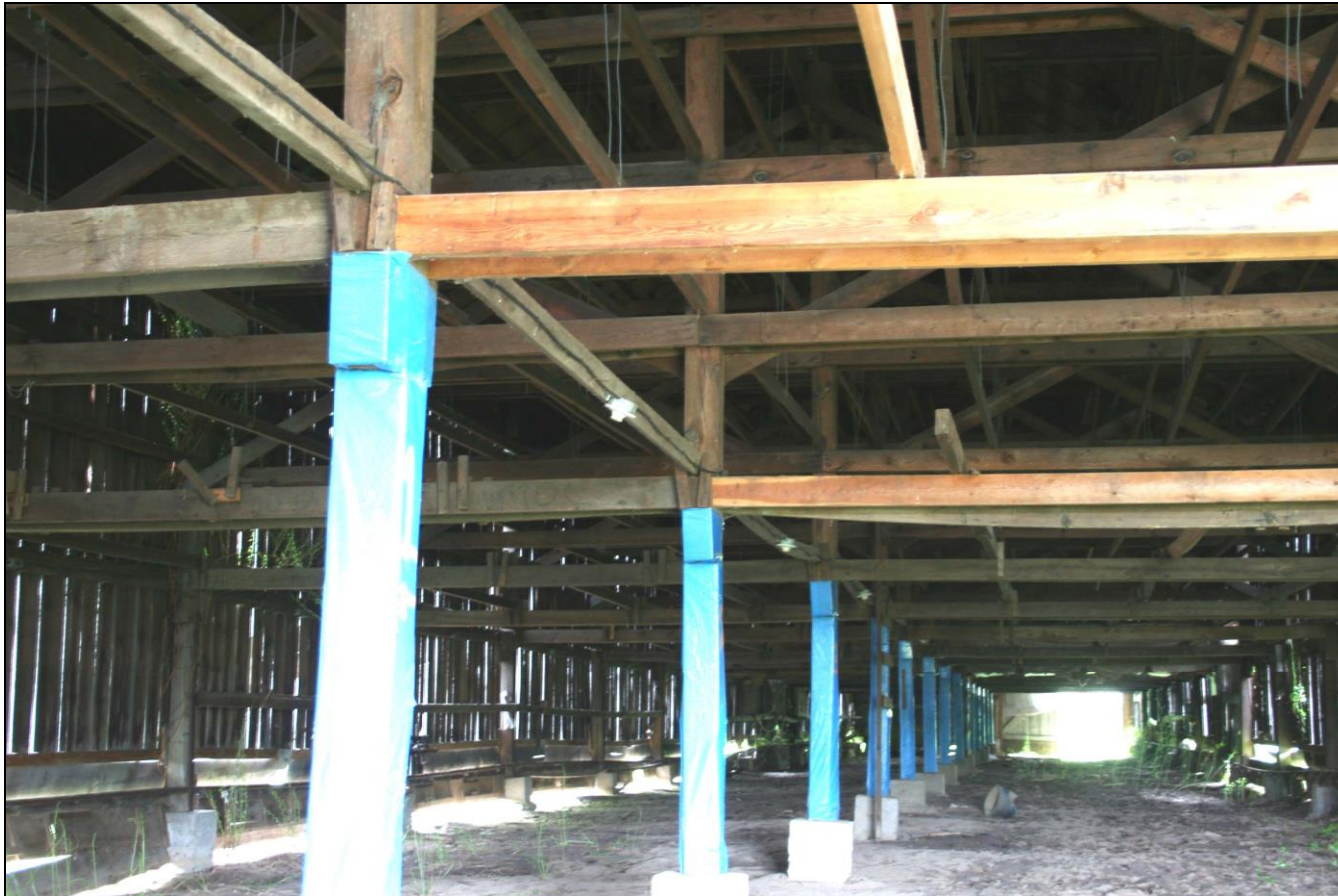
Photograph 79: Barn H (104), overview of interior from south end.
