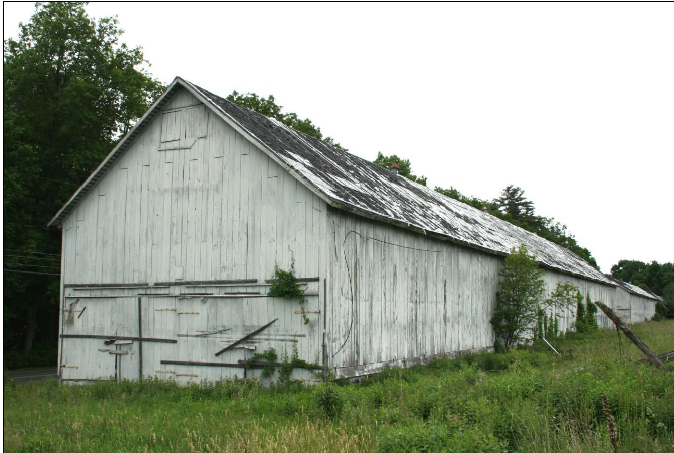
Photograph 32: Barn C (20), north and west elevations, camera facing southeast.
