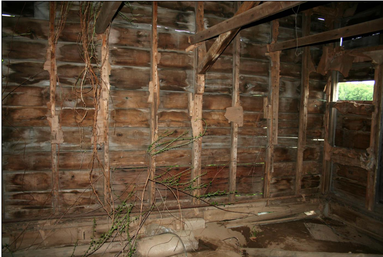
Photograph 101: Barn J, interior, detail of balloon-framed wall.
