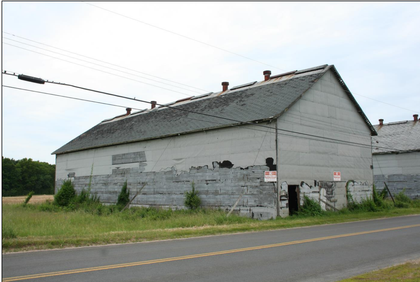
Photograph 97: Barn J (unnumbered), east and north elevations, camera facing southwest.
