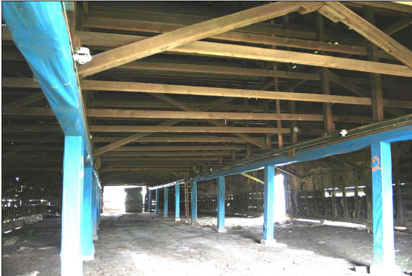
Photograph 61: Barn F (9), overview of interior from north end.
