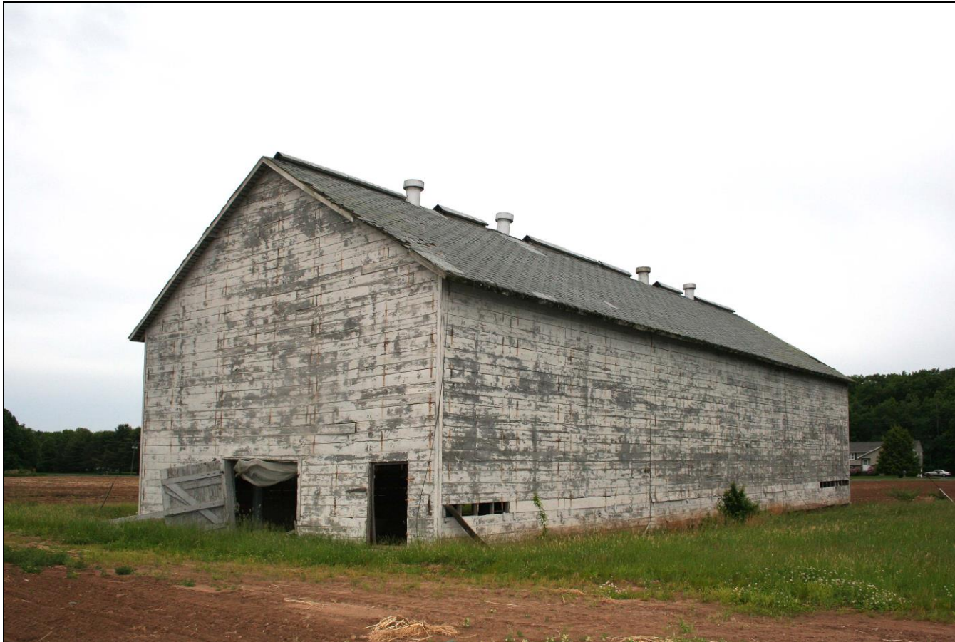
Photograph 45: Barn D (7), north and west elevations, camera facing southeast.
