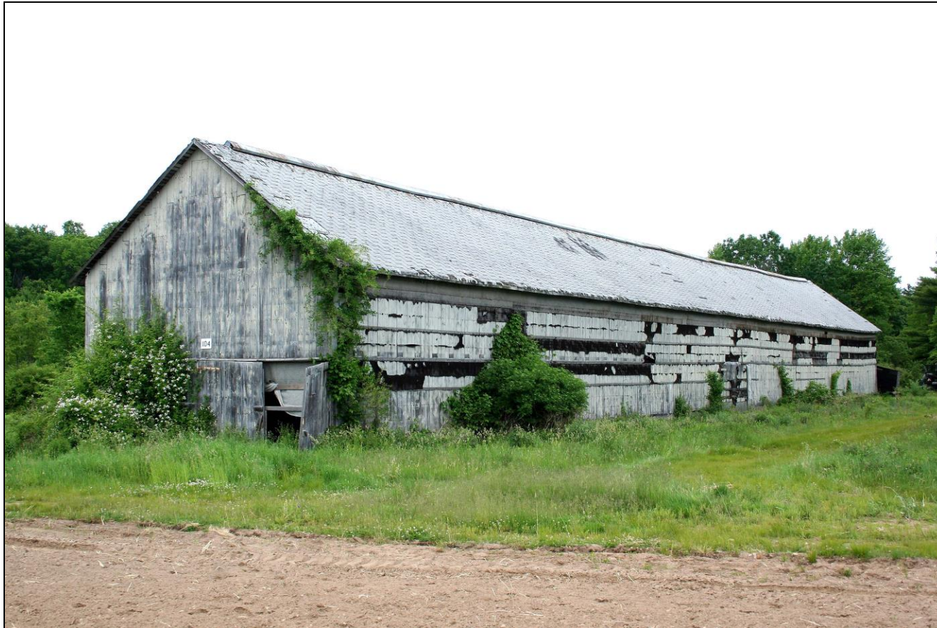
Photograph 76: Barn H (104), south and east elevations, camera facing northeast.
