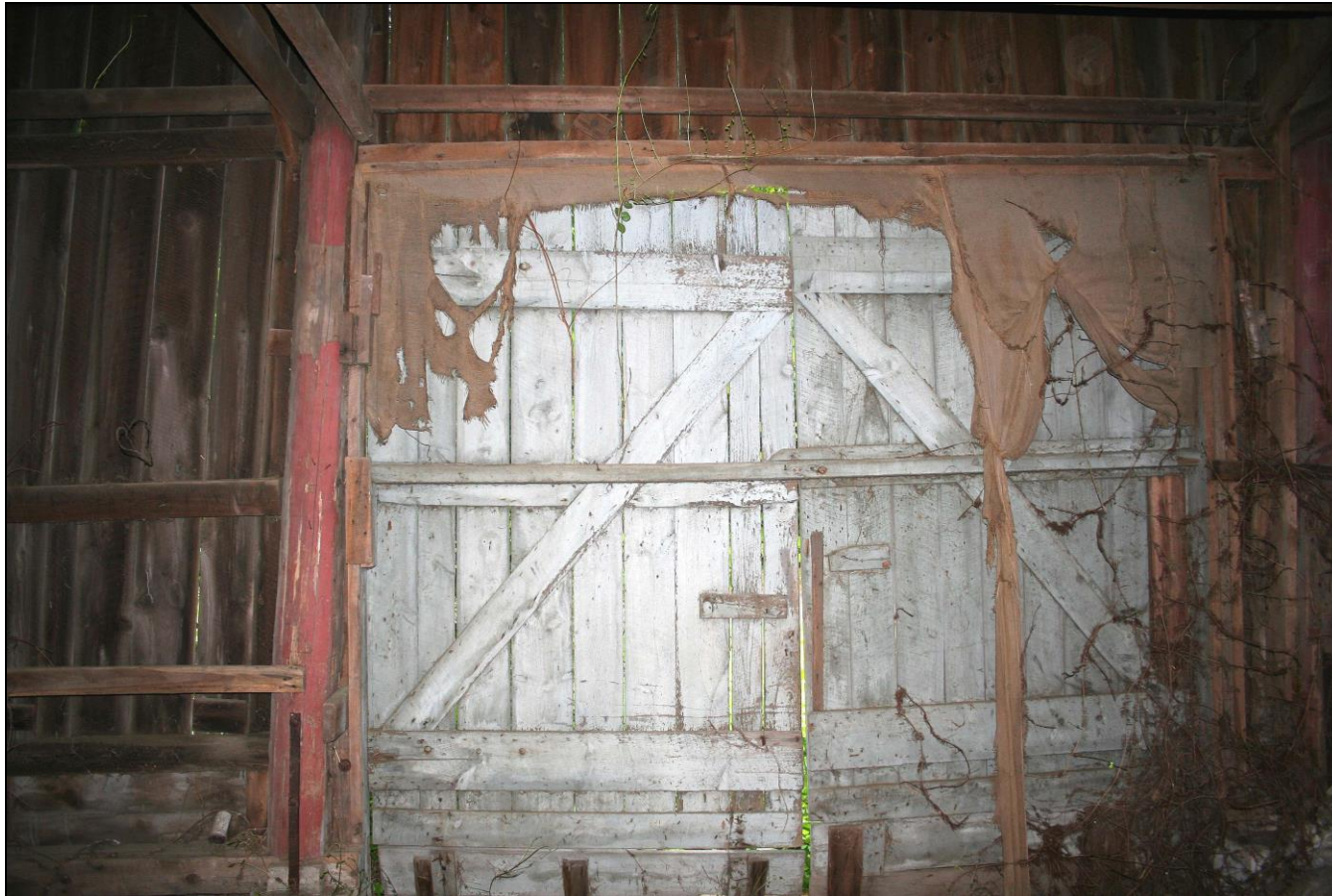
Photograph 18: Detail of interior of east side door, Barn A (2-18/18).
