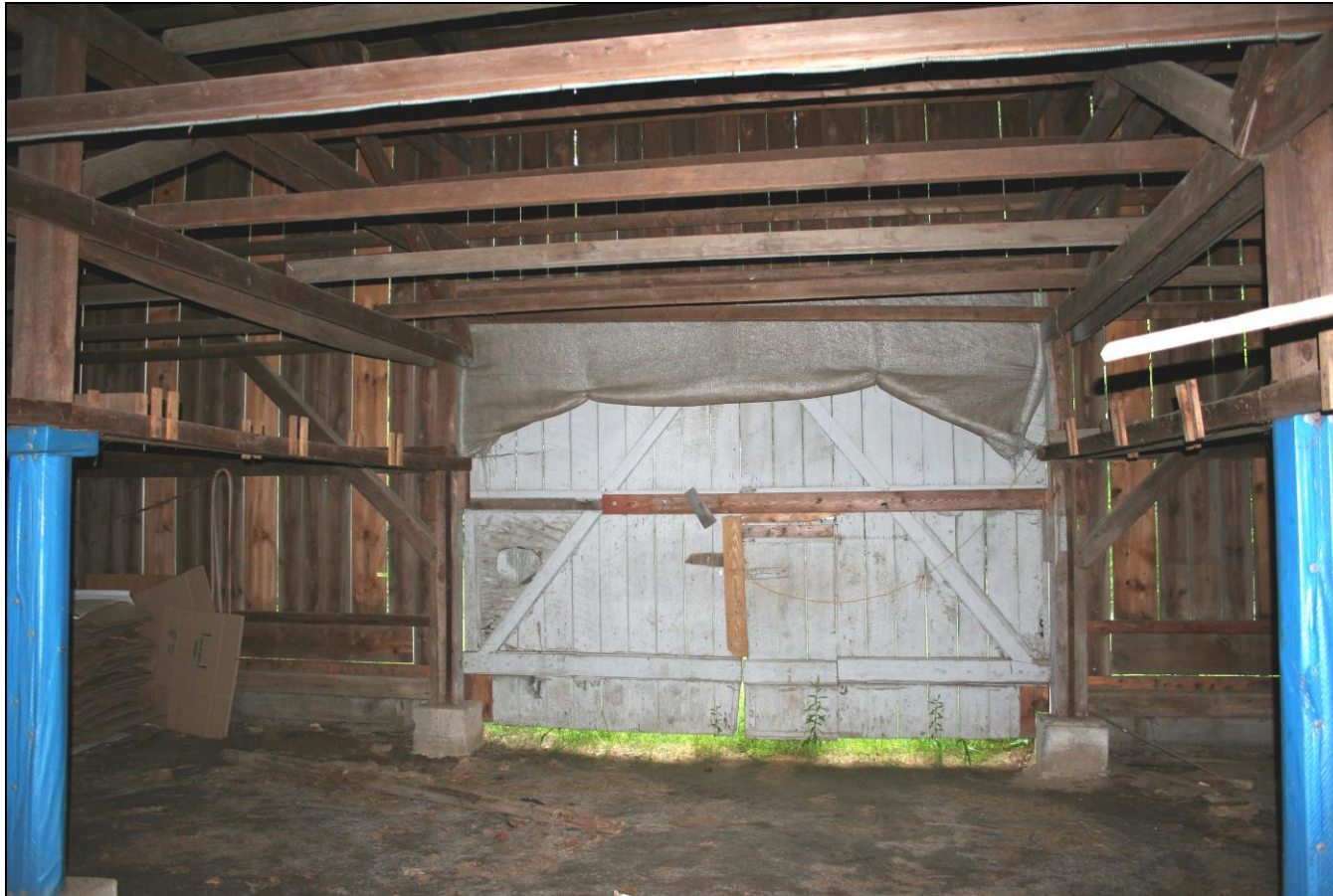
Photograph 28: Barn B (19), interior, detail of inside of east-side door.
