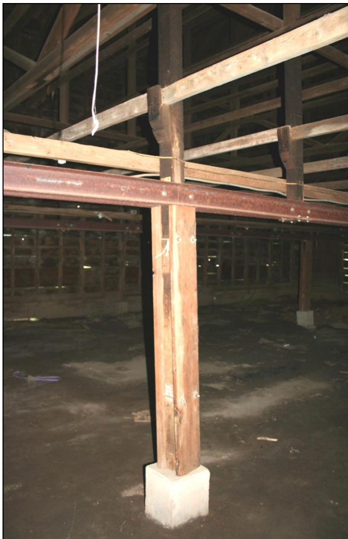
Photograph 109: Barn K (2-13), interior, detail of post, footing, and steel channel.
