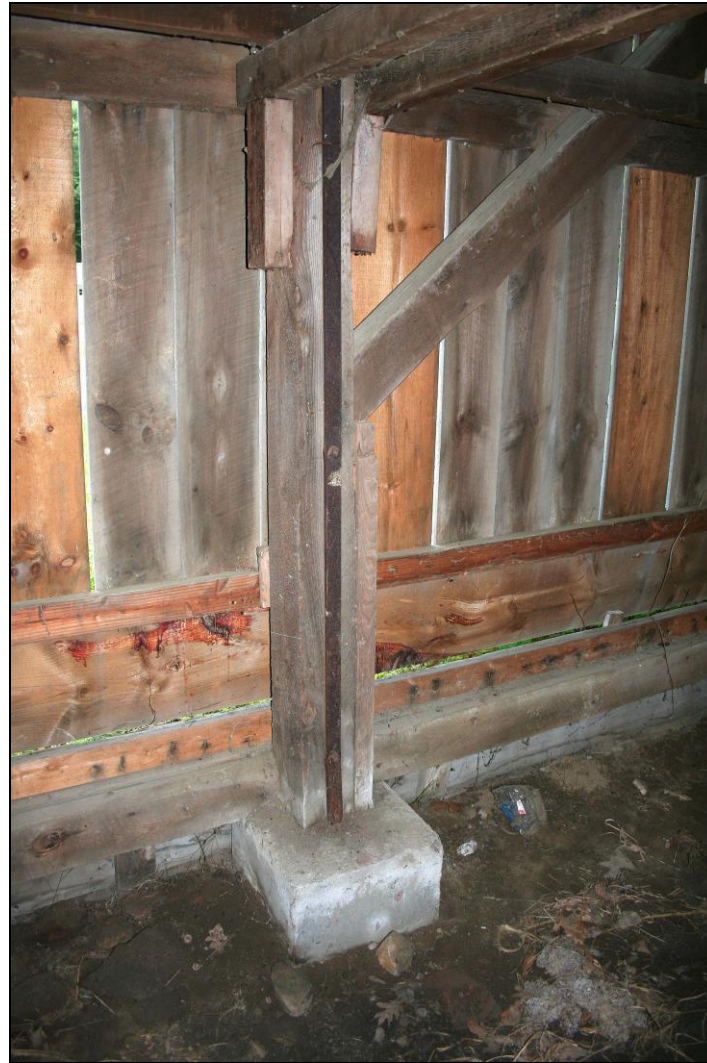
Photograph 26: Barn B (19), interior, detail of pedestal and post anchor-strap.
