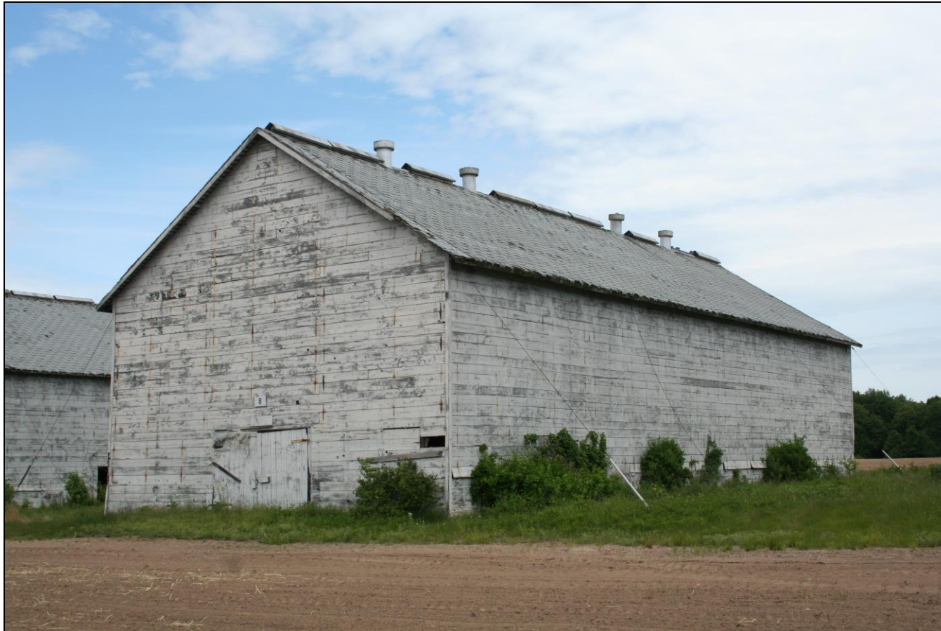
Photograph 51: Barn E (8), south and east elevations, camera facing northwest.
