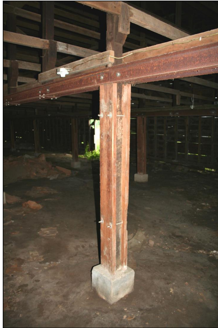
Photograph 102: Barn J, interior, detail of post, footing and steel channel.
