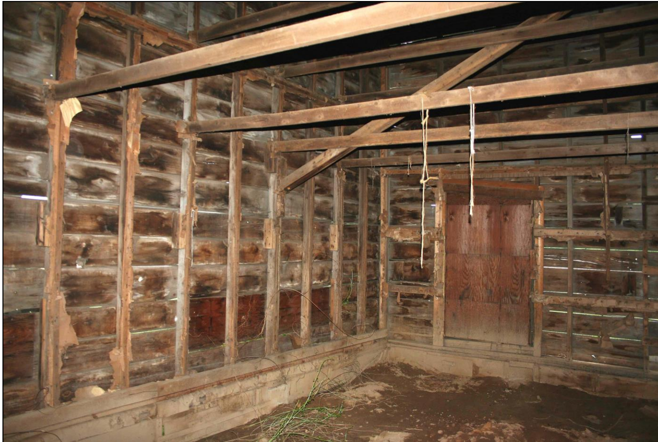
Photograph 108: Barn K (2-13), interior, detail of wall framing.
