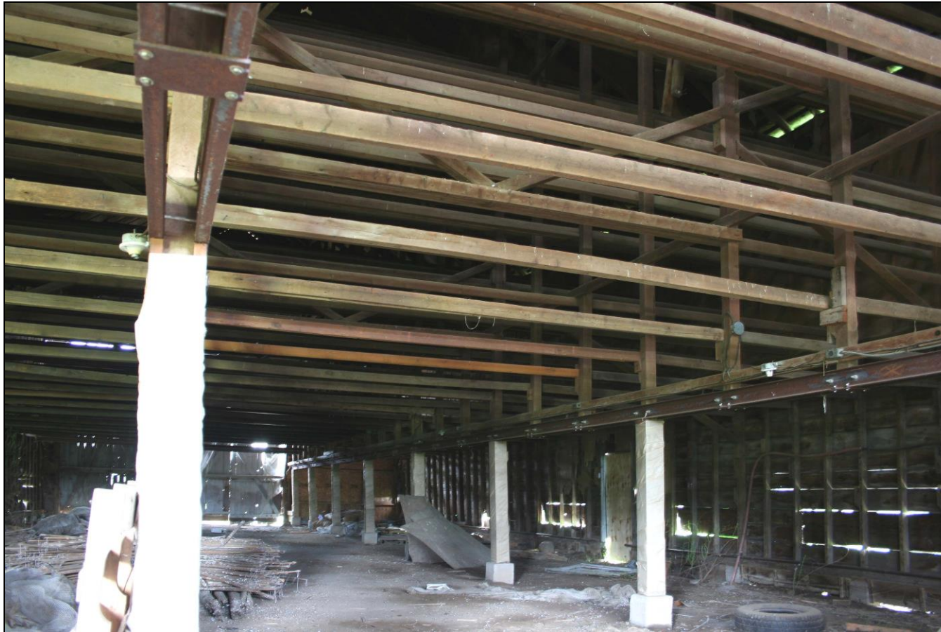
Photograph 91: Barn I, overview of interior from north end.
