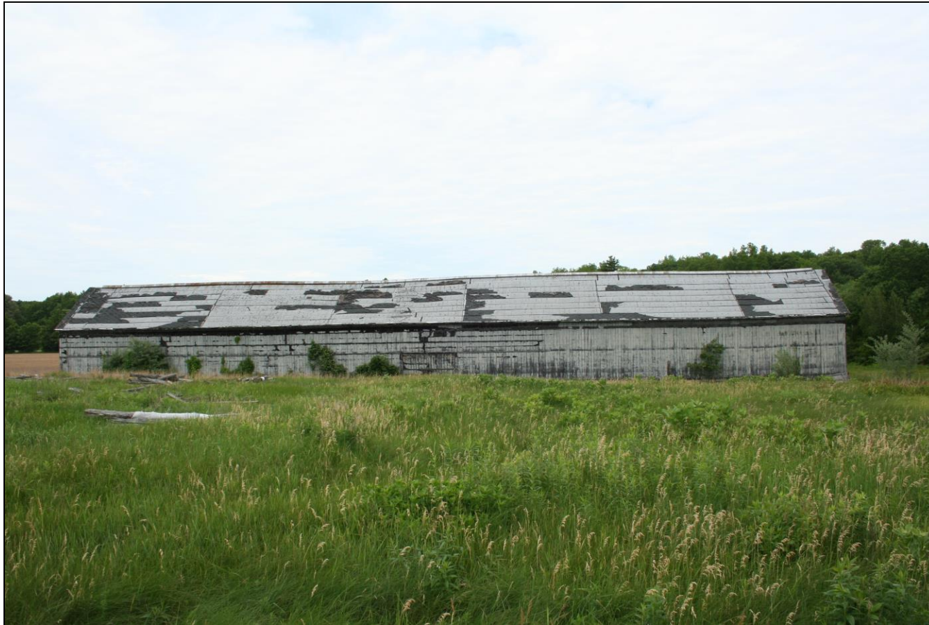
Photograph 69: Barn G (103), side view (east elevation), camera facing west.
