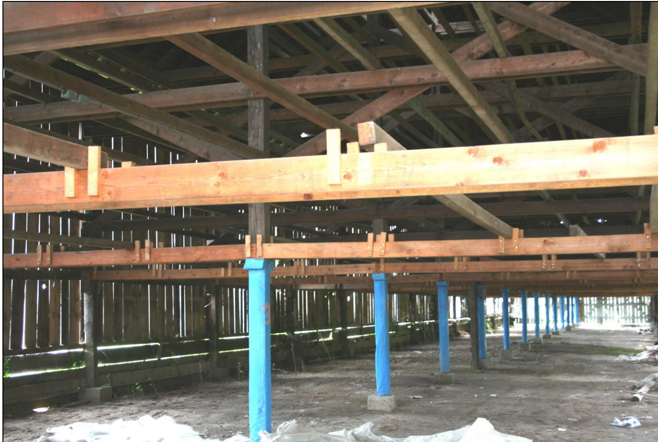
Photograph 35: Barn C (20), overview of interior from south end.
