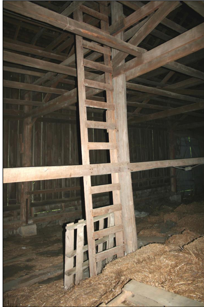
Photograph 19: Detail of ladder leading up into tiers, Barn A (2-18/18).
