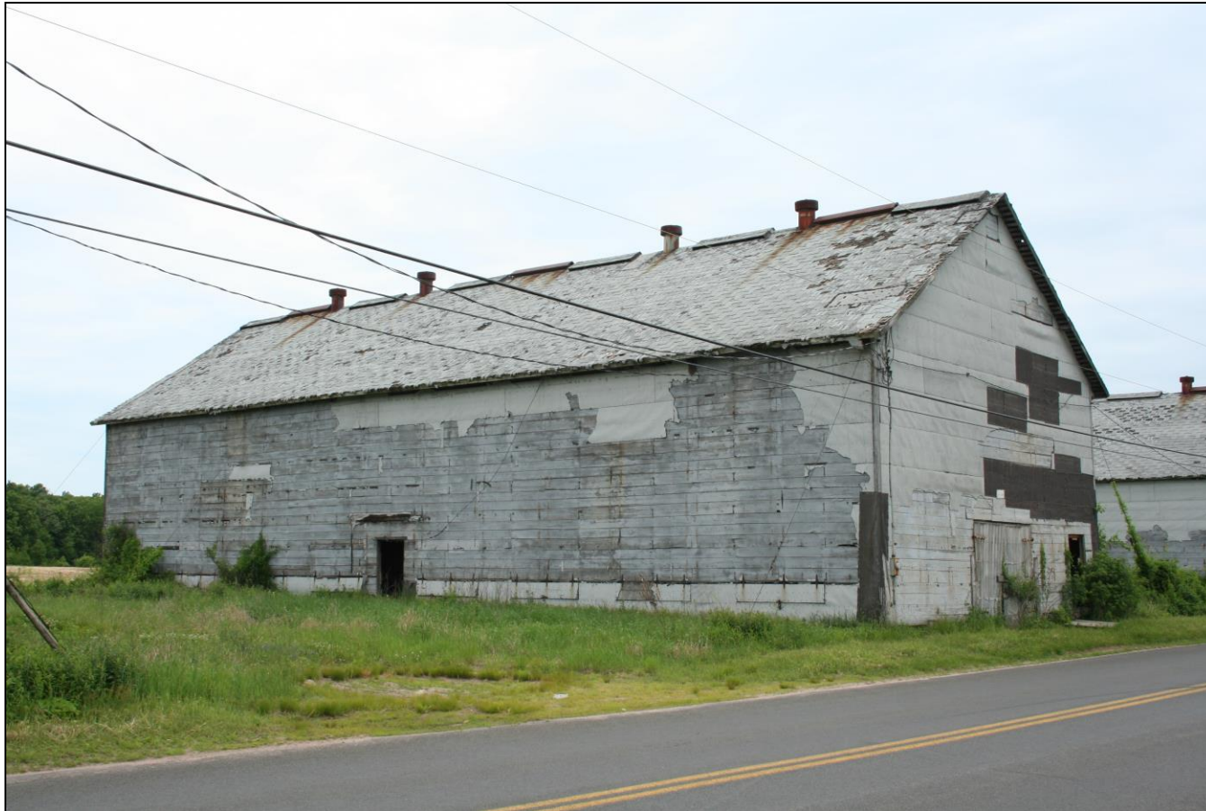
Photograph 113: Barn L (2-14), east and north elevations, camera facing southwest.
