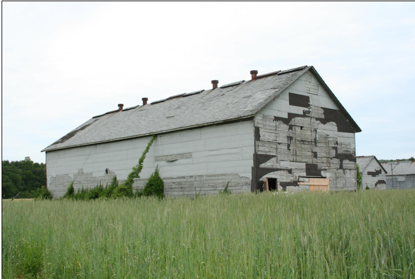
Photograph 90: Barn I, east and north elevations, camera facing southwest.
