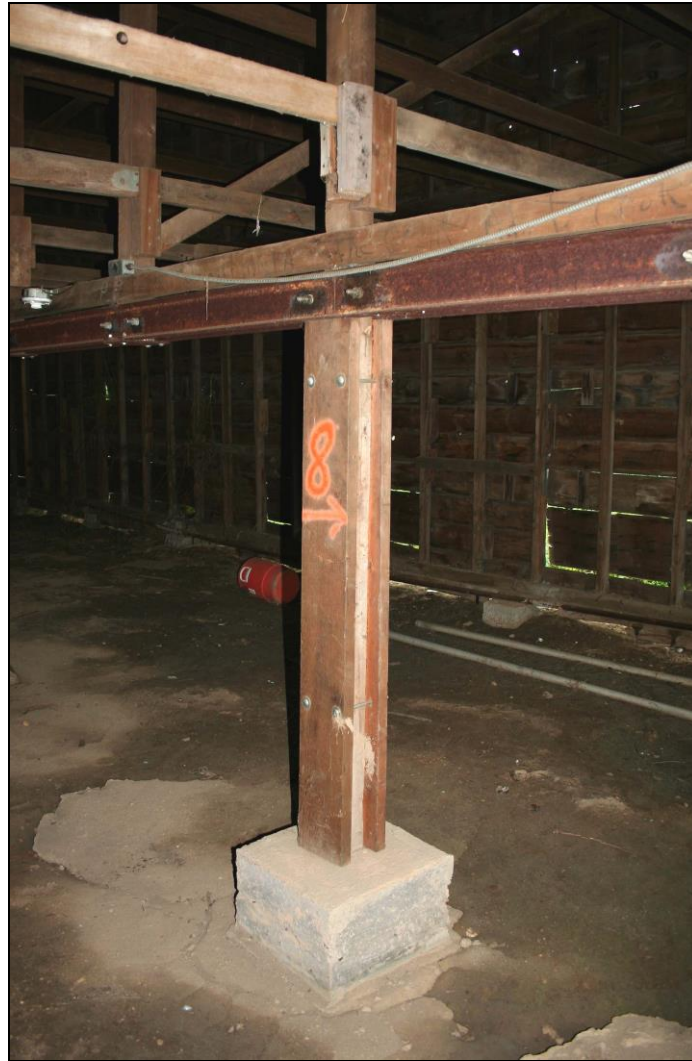
Photograph 132: Barn N (2-16), interior, detail of typical post and footing.
