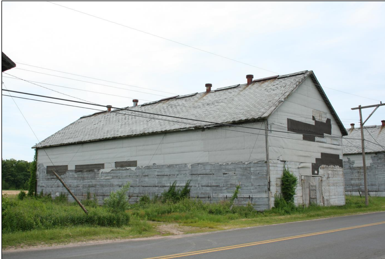
Photograph 105: Barn K (2-13), east and north elevations, camera facing west.
