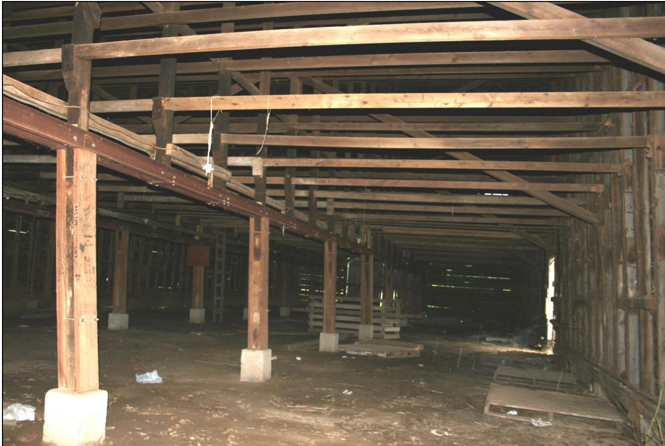
Photograph 107: Barn K (2-13), overview of interior from north end.
