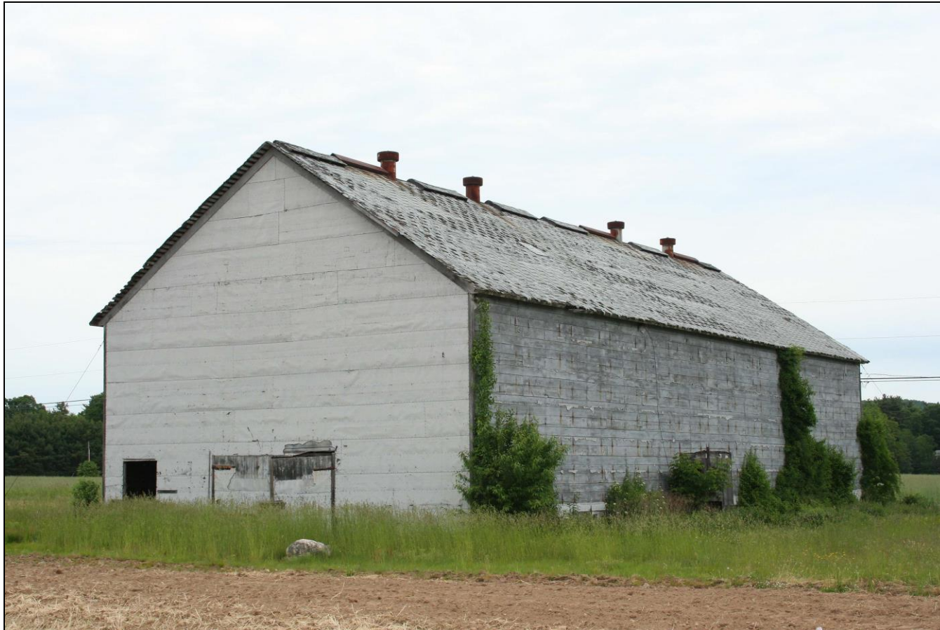
Photograph 128: Barn N (2-16), south and east elevations, camera facing north.
