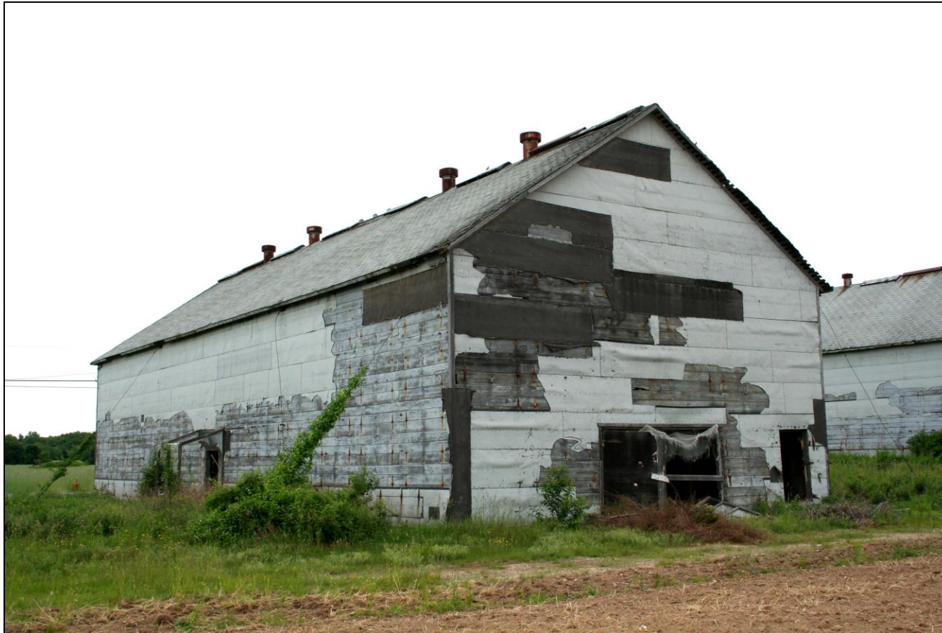
Photograph 121: Barn M (2-15), west and south elevations, camera facing northeast.
