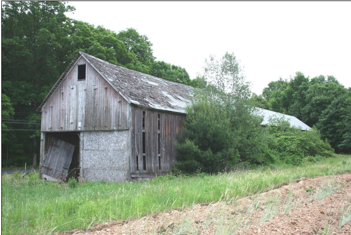
Photograph 7: Barn A (2-18/18), north and west elevations, camera facing southeast.
