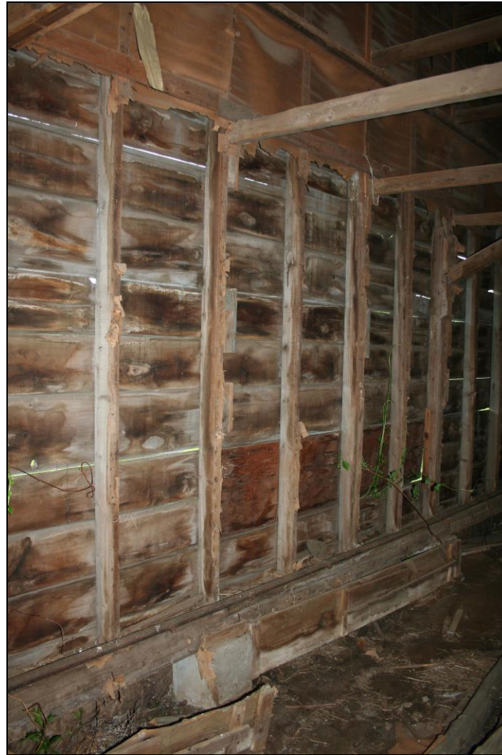
Photograph 92: Barn I, interior, detail of balloon-framed wall.
