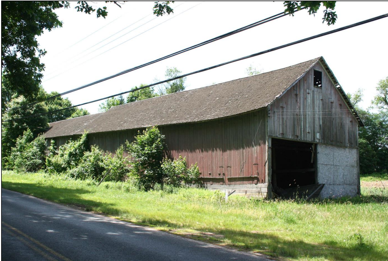
Photograph 6: Barn A (2-18/18), east and north elevations, camera facing south.
