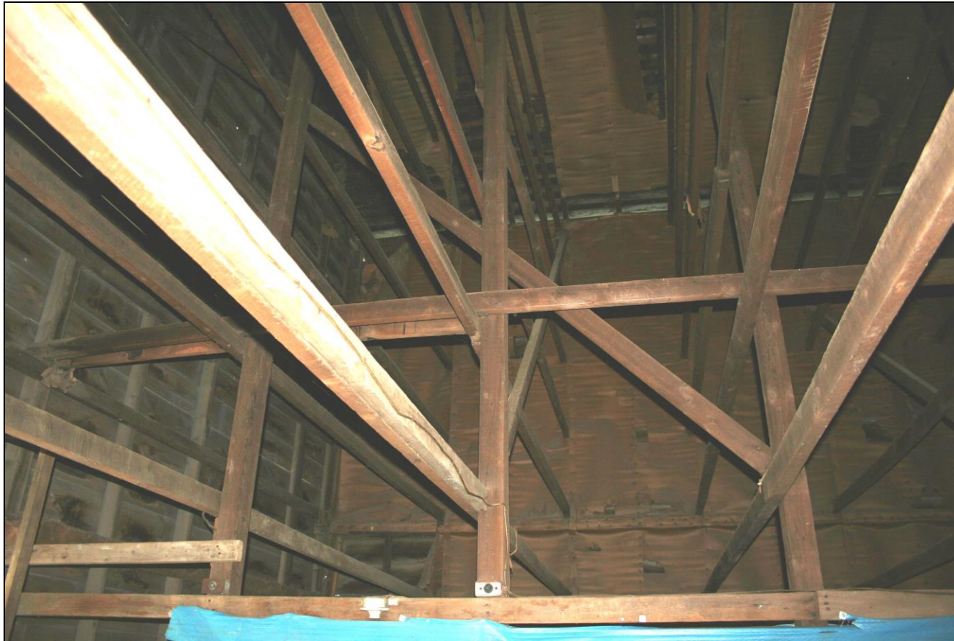
Photograph 58: Barn E (8), interior, detail of diagonal wind brace for end wall.
