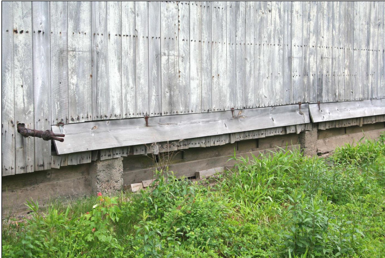
Photograph 71: Barn G (103), detail of exterior gas fittings and hinged boards.
