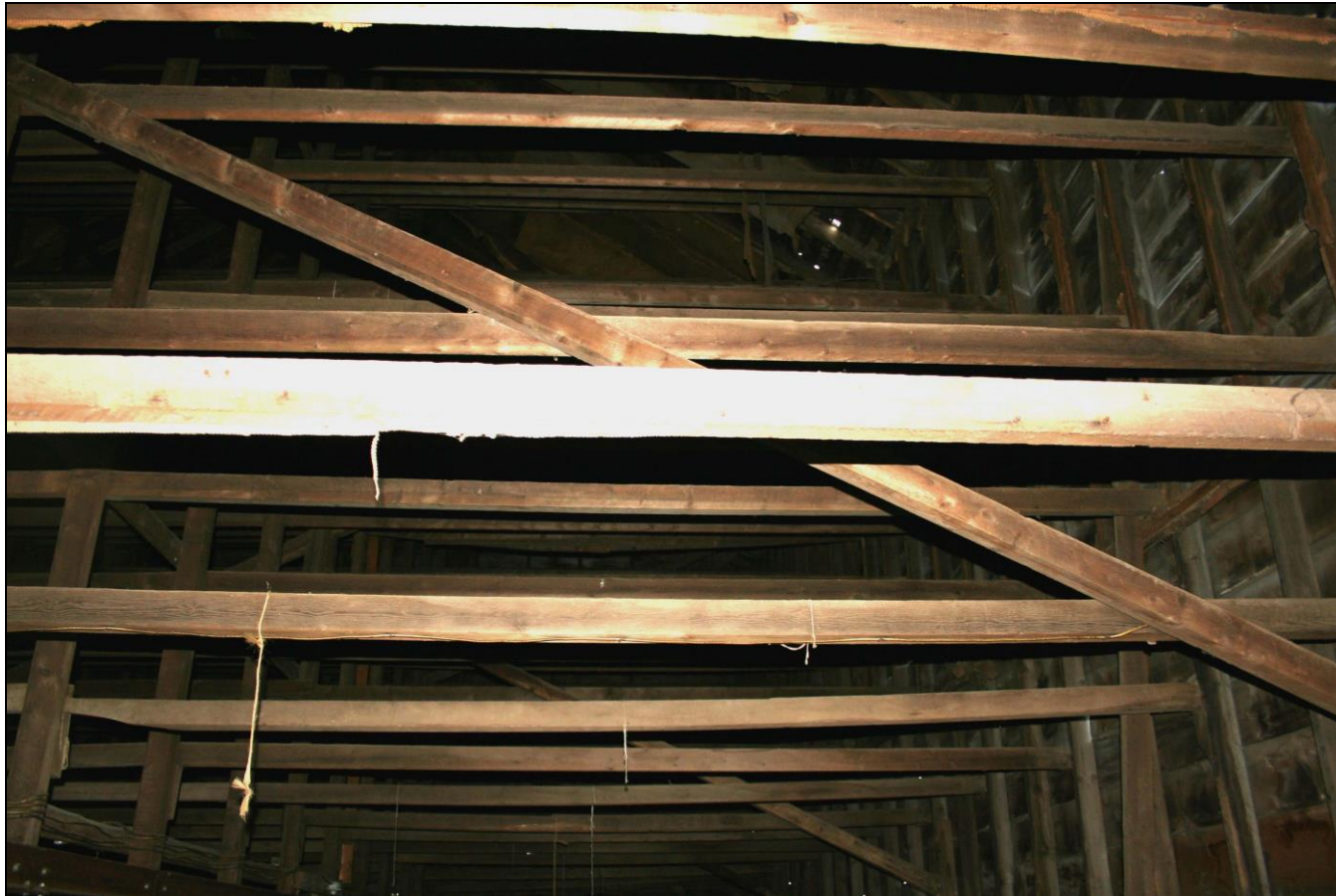
Photograph 117: Barn L (2-14), interior, detail of diagonal bracing.
