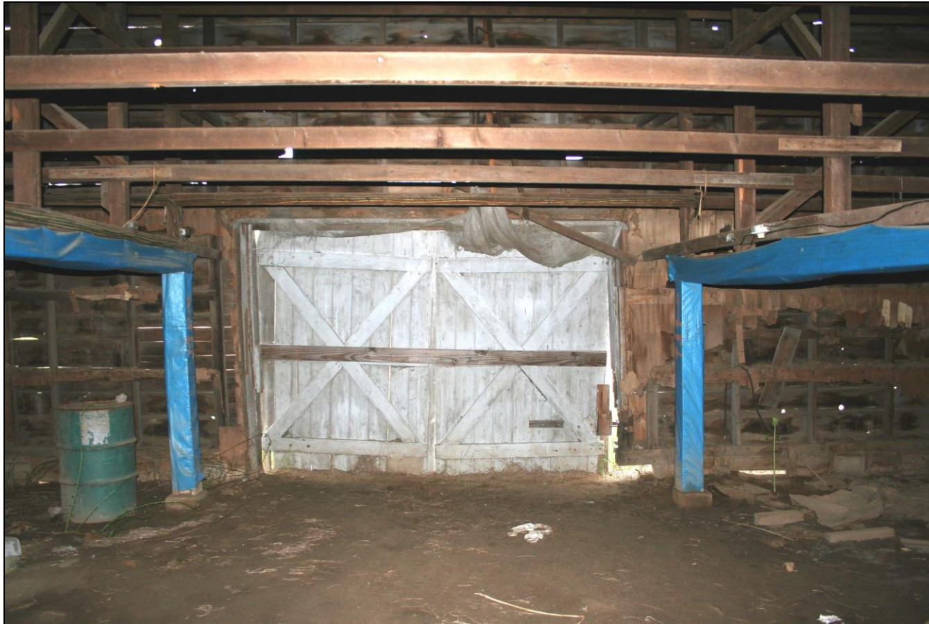
Photograph 57: Barn E (8), interior, detail of inside of south-end doors.
