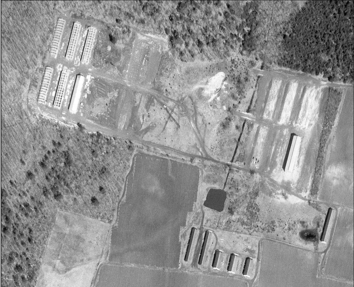
Figure 7: State of Connecticut aerial photograph of March 1965, showing tobacco barns under construction north of Barns G and H. The filled and leveled dirt floors for several barns not yet being built can be discerned, as well as one in which the footings have been completed. Three of the barns at the upper left have been completed to the point of having their side and end walls, needing only the roofs to finish them. The two at the far left are frames only. Eight barns in this area survive, but they were not included in this documentation because of their relatively late date of construction.
