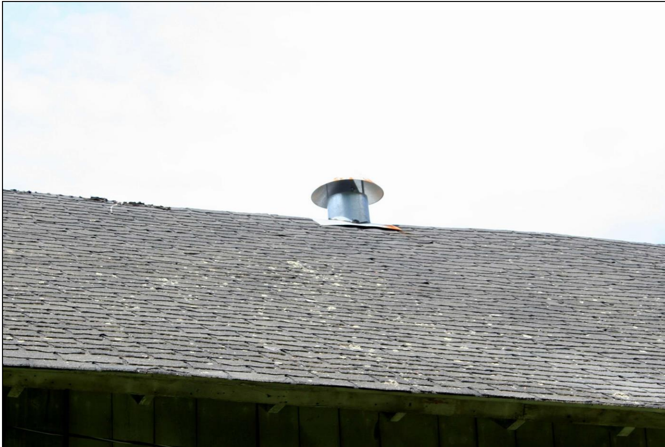
Photograph 24: Barn B (19), detail of rooftop ventilator.
