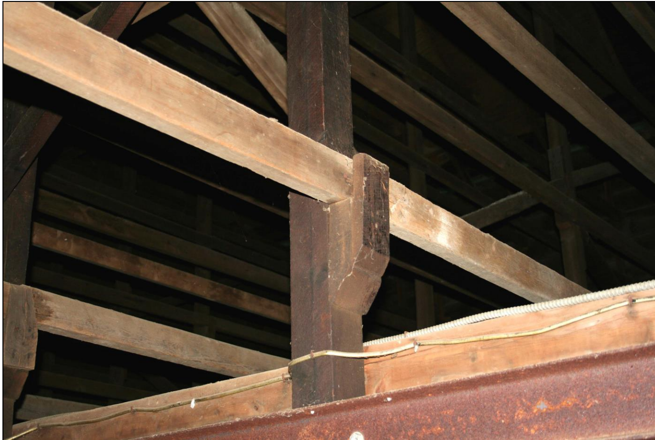
Photograph 103: Barn J, interior, detail of bracket for transverse tier timbers.
