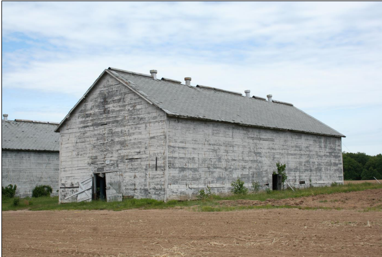
Photograph 44: Barn D (7), south and east elevations, camera facing northwest.
