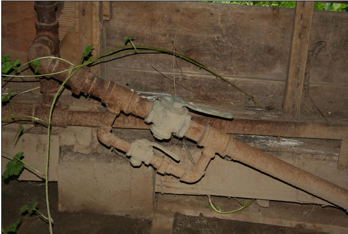
Photograph 118: Barn L (2-14), interior, detail of gas fittings.
