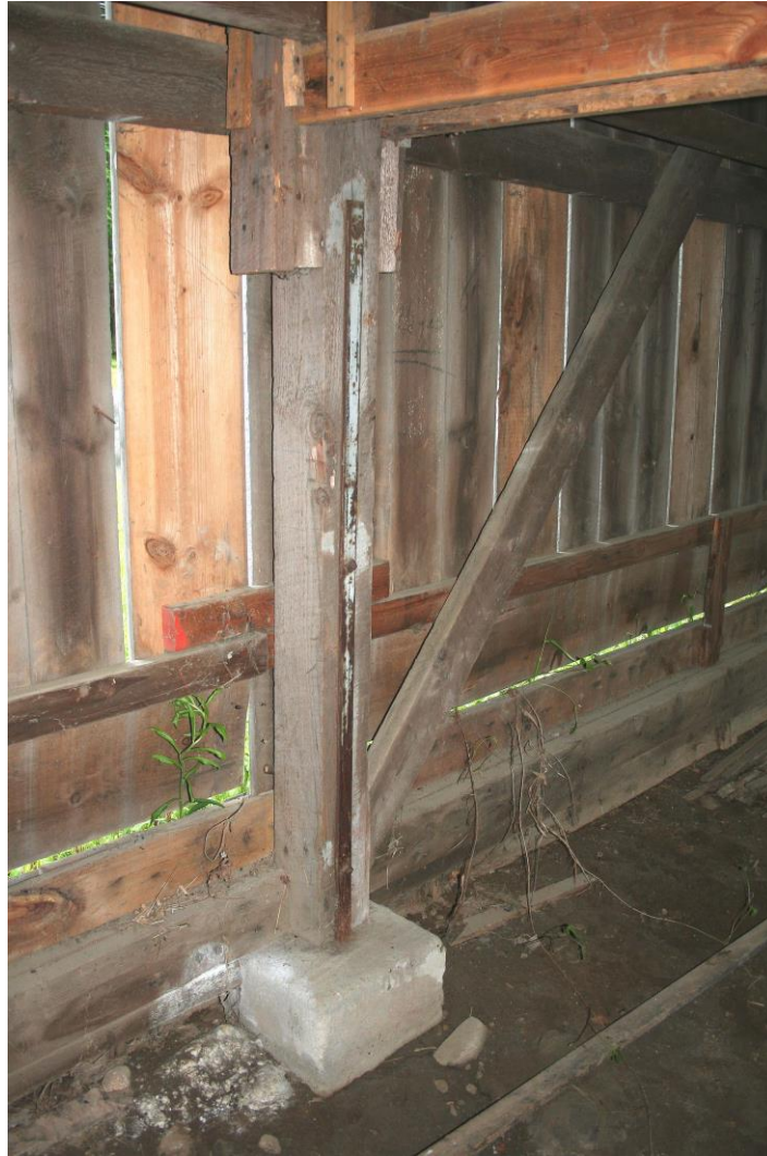
Photograph 36: Barn C (20), interior, detail of pedestal, post, sill and diagonal wind brace.
