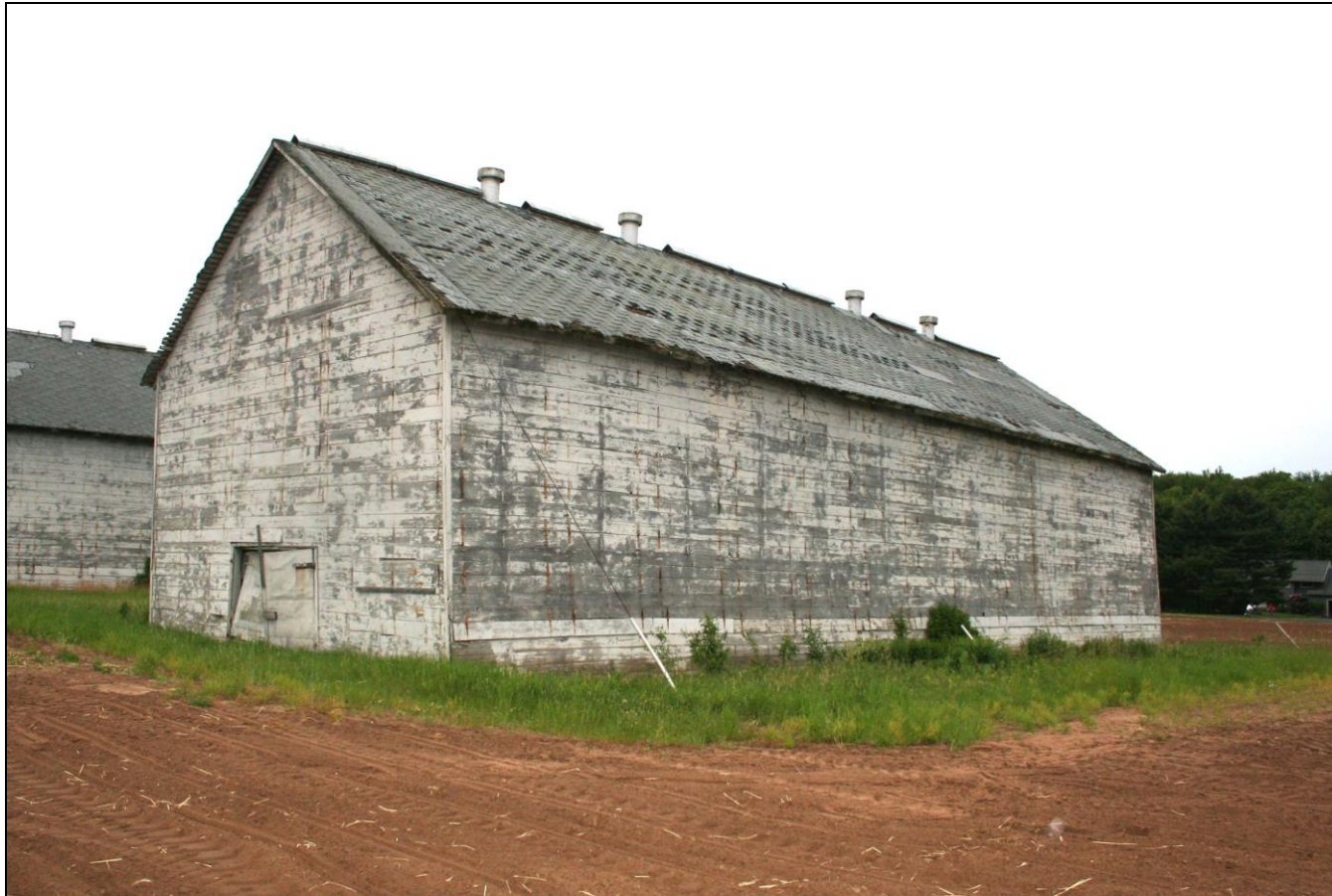
Photograph 60: Barn F (9), north and west elevations, camera facing southeast.
