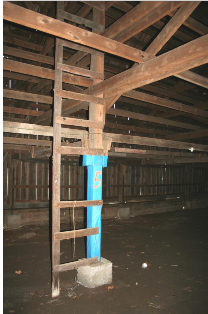
Photograph 82: Barn H (104), interior, detail of post, footing, and ladder to tiers.
