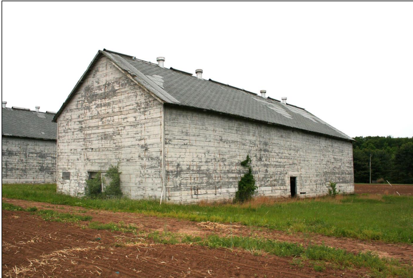
Photograph 52: Barn E (8), north and west elevations, camera facing southeast.
