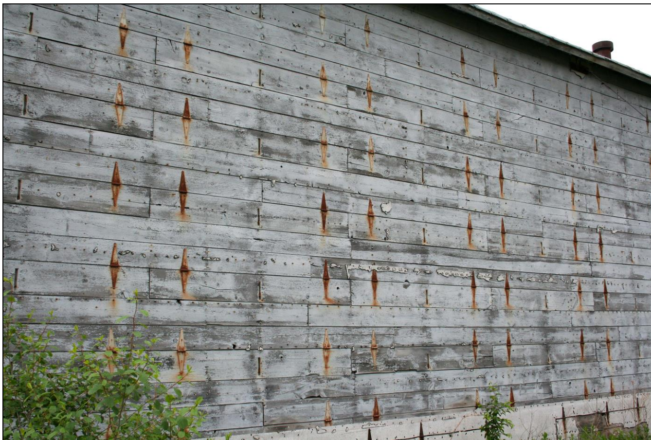
Photograph 130: Barn N (2-16), detail of hinged boards, west side.
