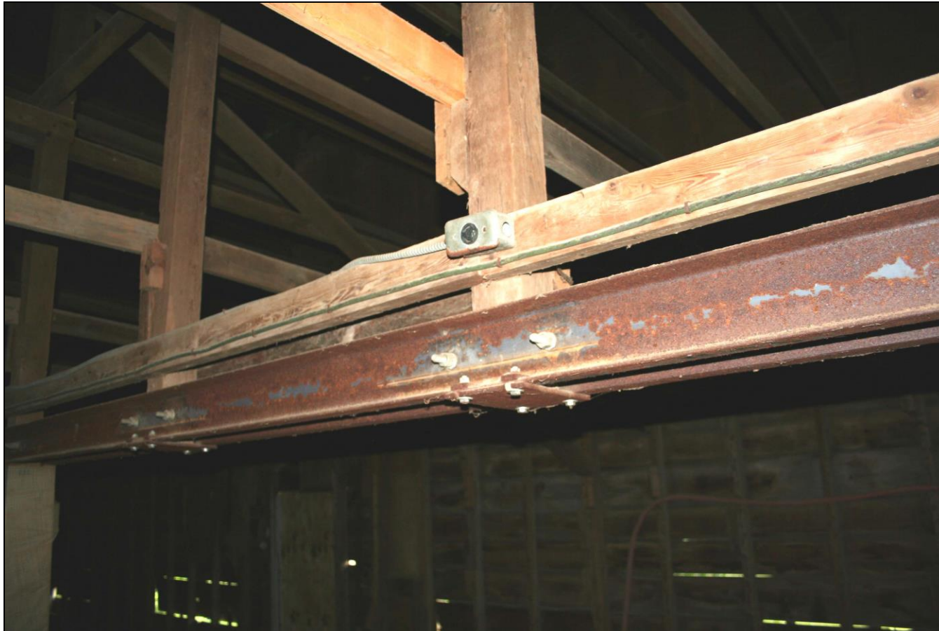
Photograph 93: Barn I, interior, detail of longitudinal steel channels.
