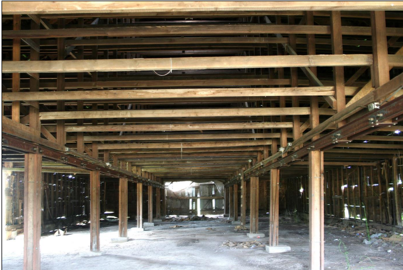
Photograph 123: Barn M (2-15), overview of interior from north end.
