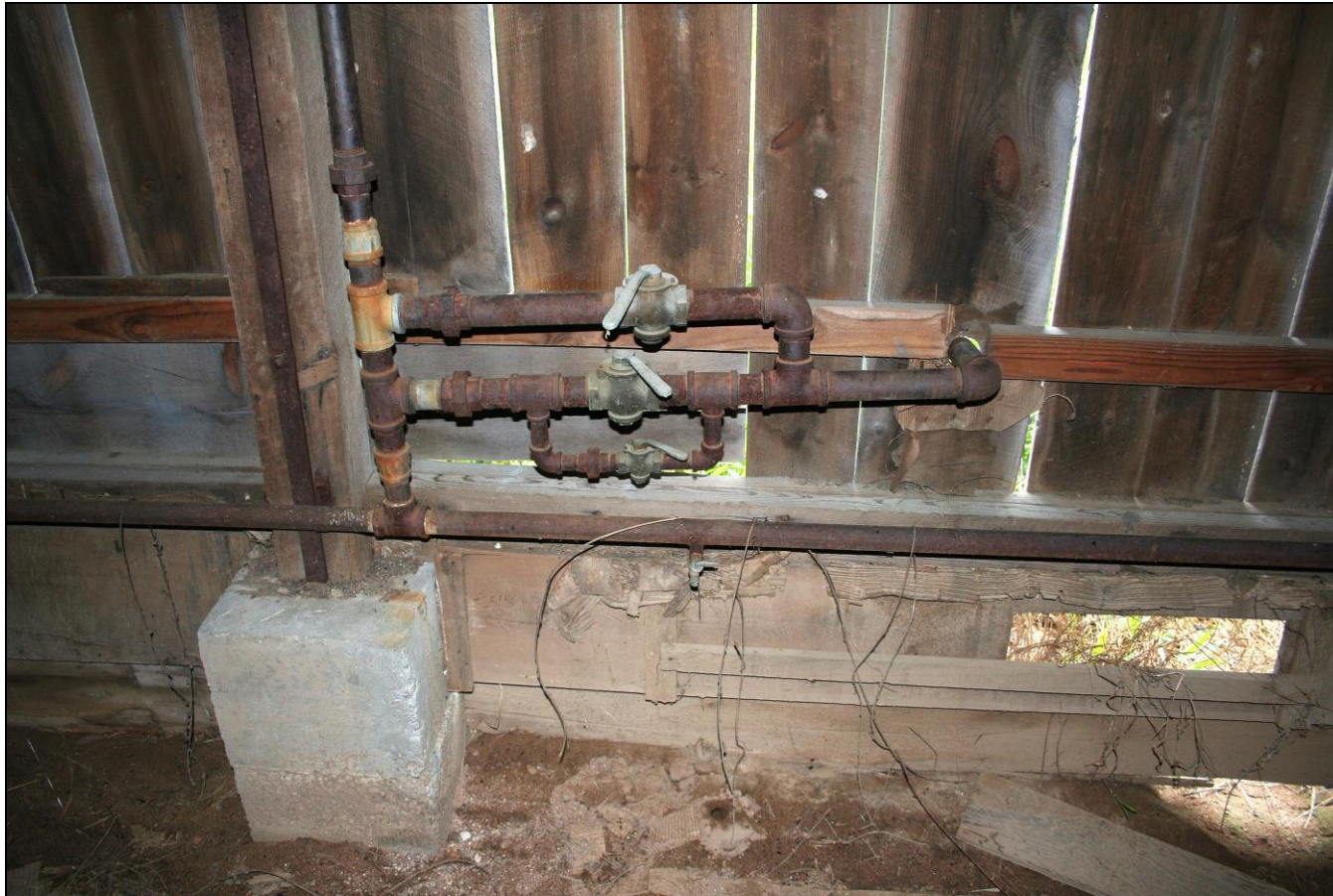
Photograph 73: Barn G (103), interior, detail of post, footing, sill, and gas piping.
