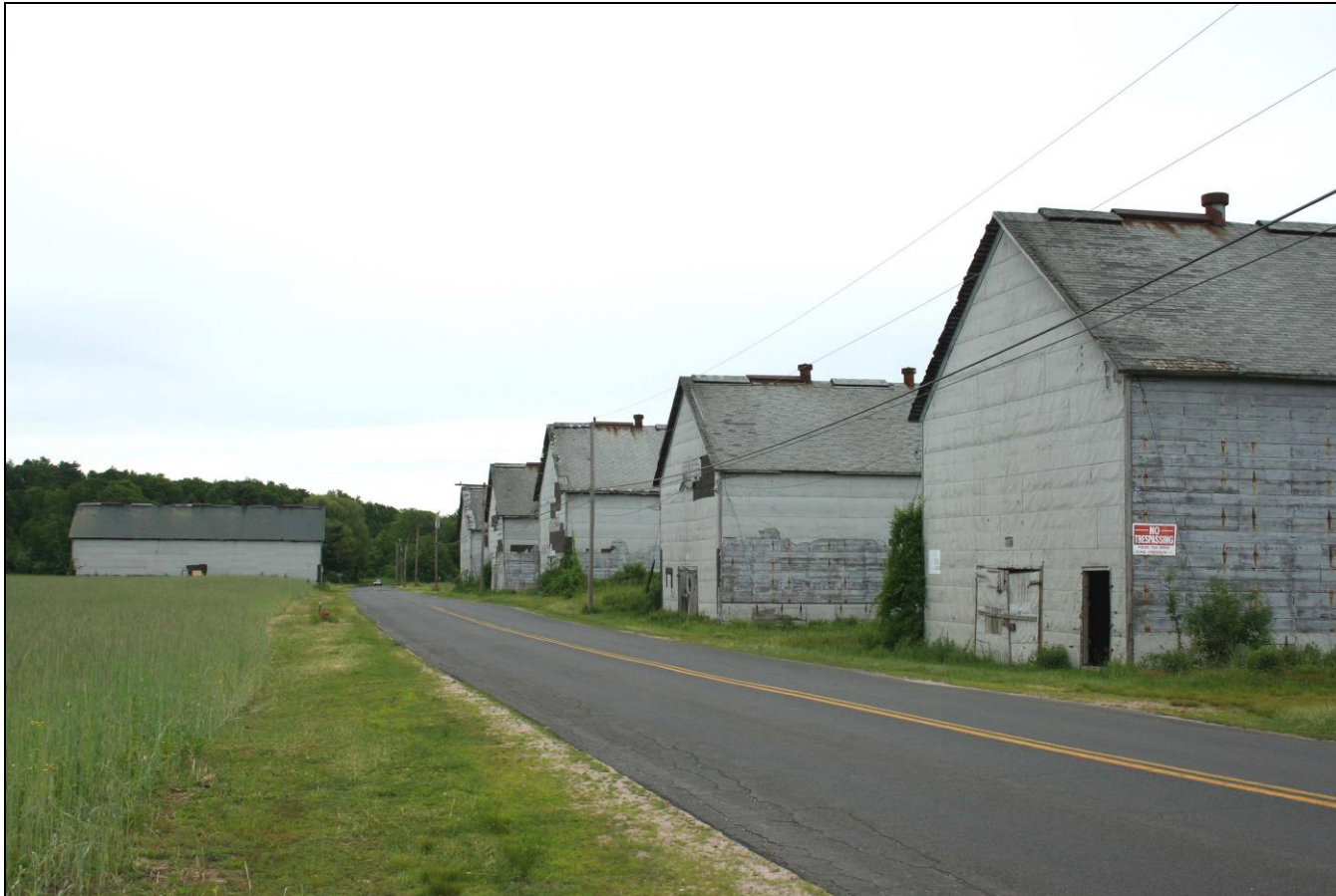
Photograph 85: Overview of barns on Firetown Road, camera facing southeast: Barn I on north side of road at left, with Barns J through N (left to right) on south side of the road at right.
