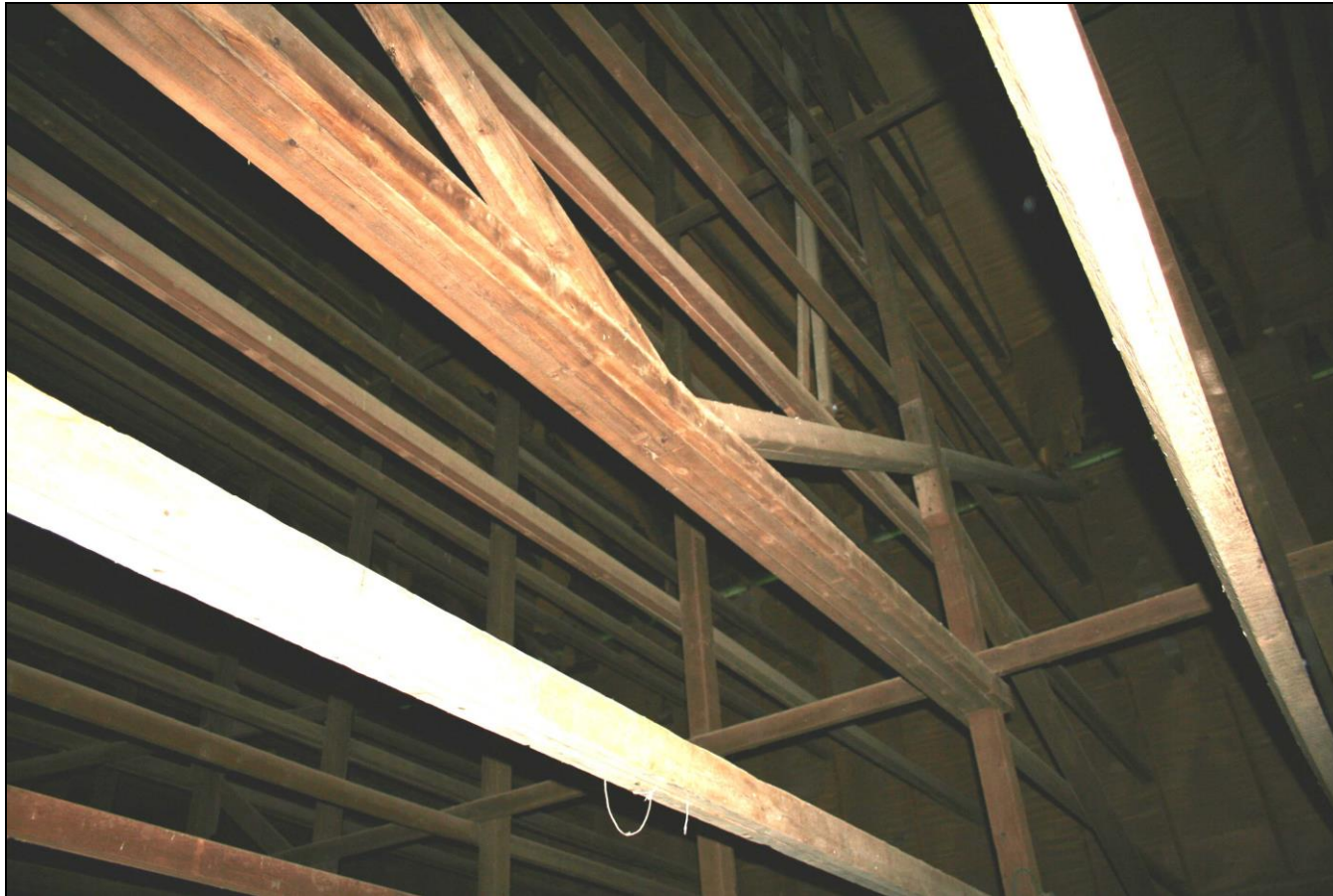
Photograph 95: Barn I, interior, detail of center transverse bracing.
