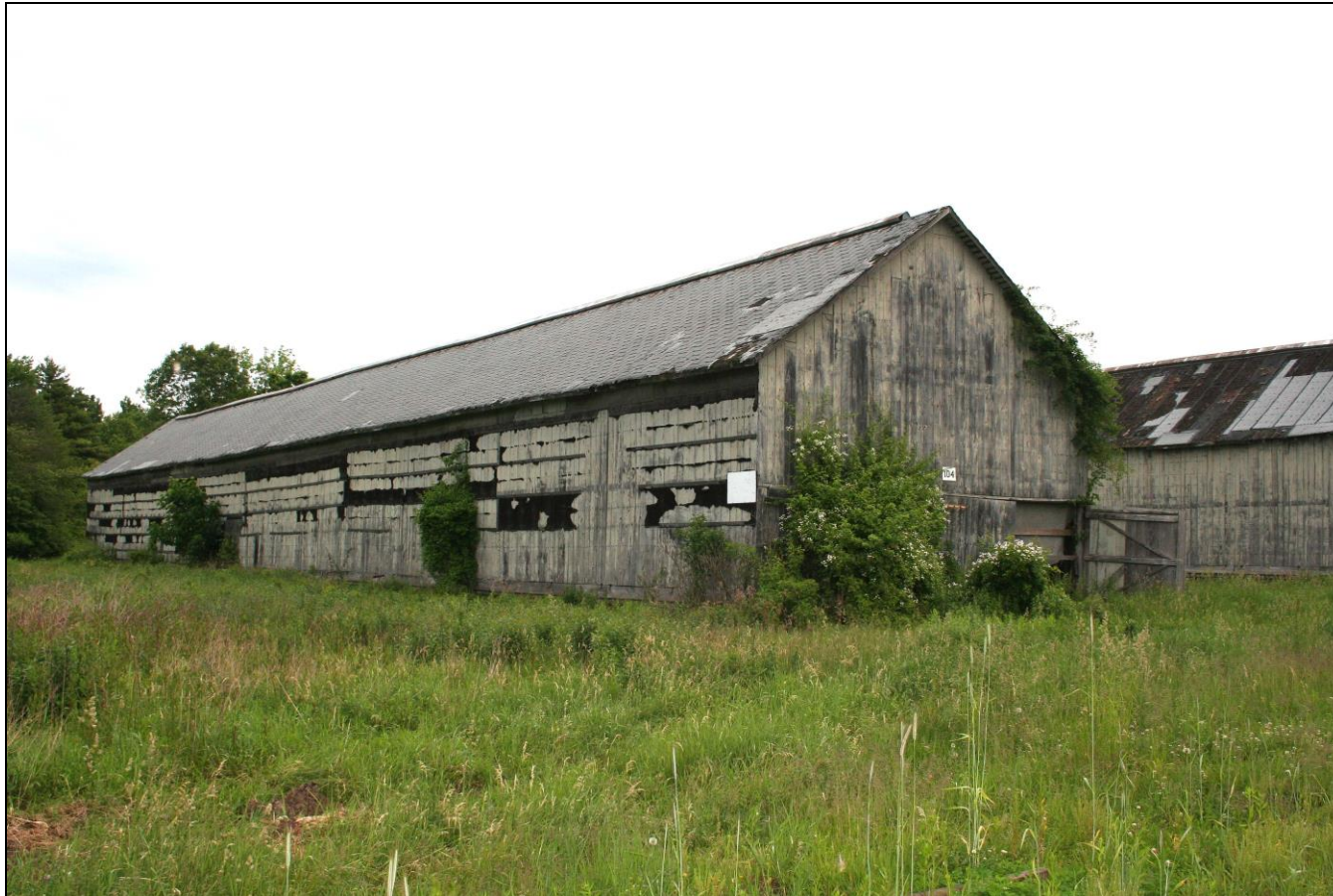
Photograph 78: Barn H (104), south and west elevations, camera facing northeast.
