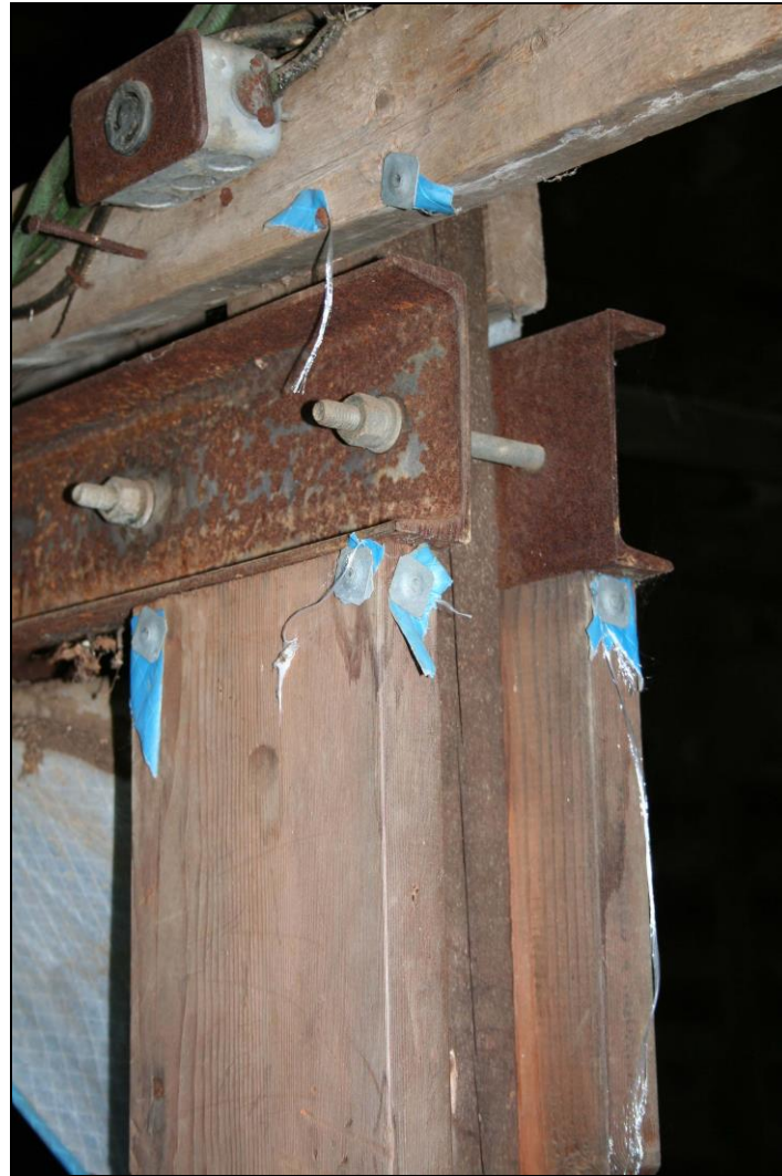
Photograph 63: Barn F (9), interior, detail of ends of steel channels.
