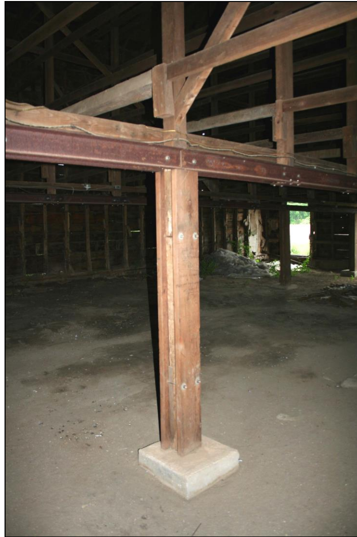
Photograph 124: Barn M (2-15), interior, detail of post, footing and steel channel.
