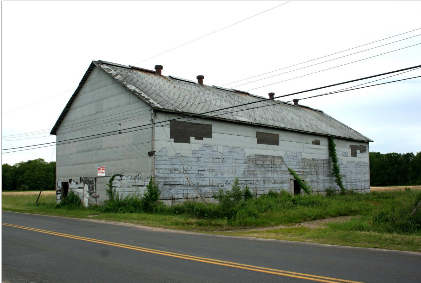
Photograph 98: Barn J, north and west elevations, camera facing southeast.
