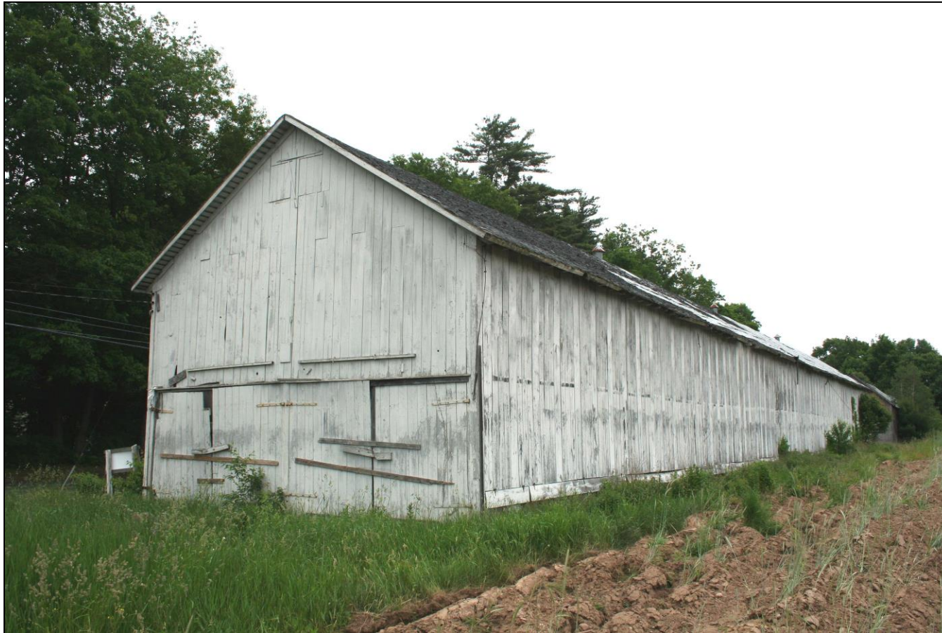
Photograph 21: Barn B (19), north and west elevations, camera facing southeast.
