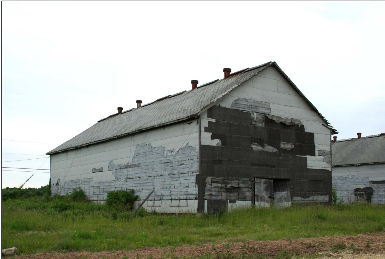
Photograph 115: Barn L (2-14), west and south elevations, camera facing northeast.
