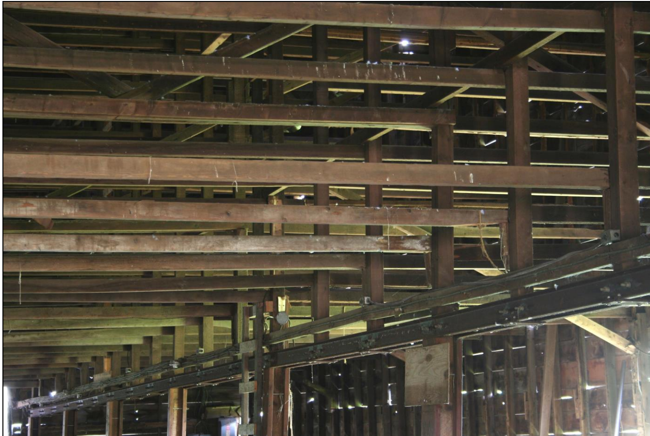
Photograph 116: Barn L (2-14), overview of interior from south end.
