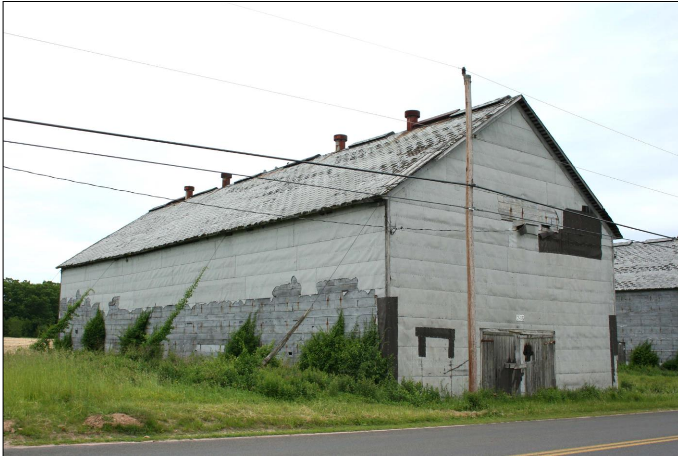
Photograph 119: Barn M (2-15), east and north elevations, camera facing southwest.
