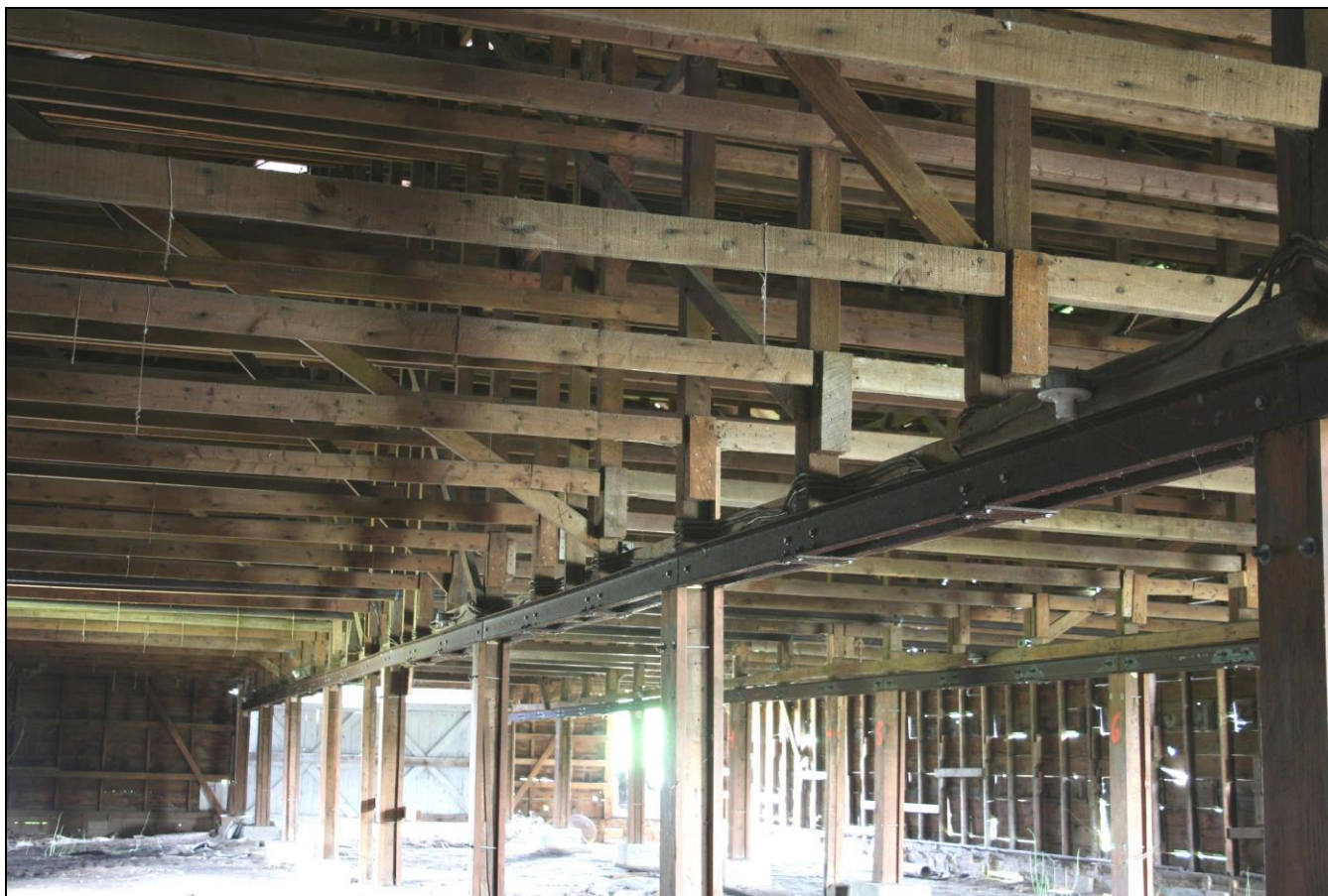
Photograph 131: Barn N (2-16), overview of interior from north end.
