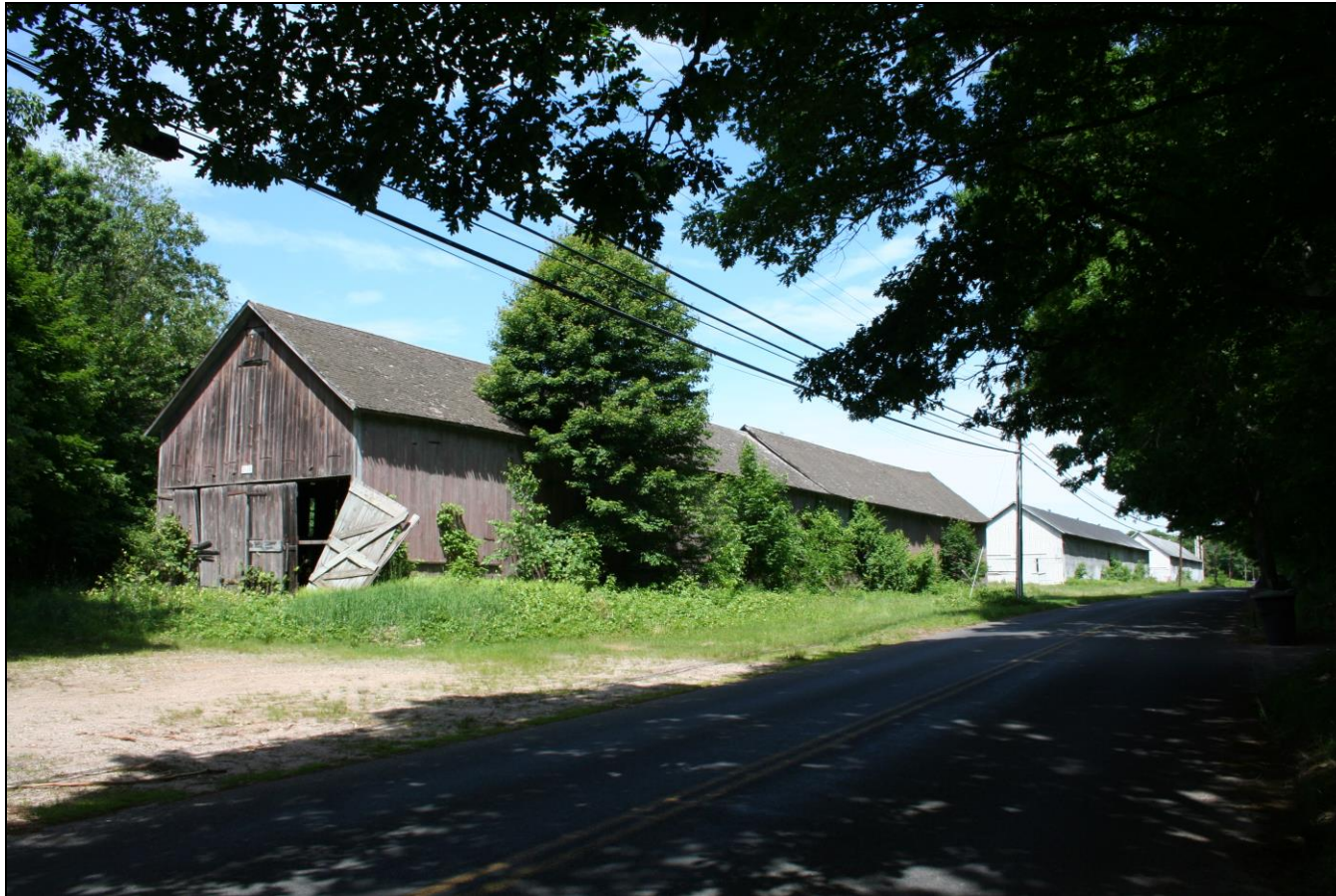
Photograph 1: Overview of barns on County Road: Barn A (2-18/18) at left, with B (19) and C (20) in background, camera facing northwest.
