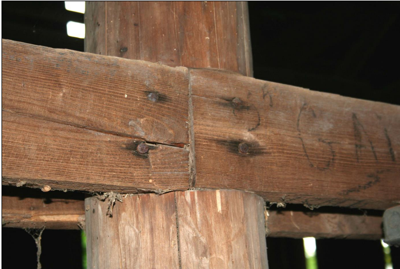
Photograph 16: Detail of post mortise for longitudinal bracing, Barn A (2-18/18).
