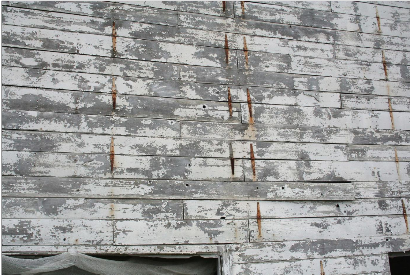
Photograph 46: Barn D (7), detail of horizontal boards and hinges.
