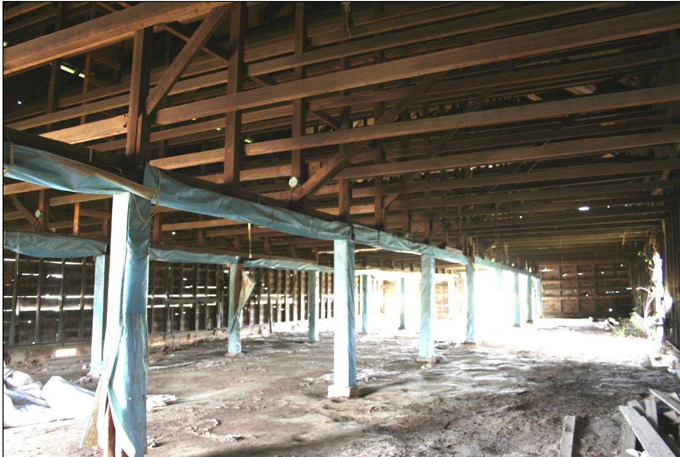
Photograph 48: Barn D (7), overview of interior from south end.
