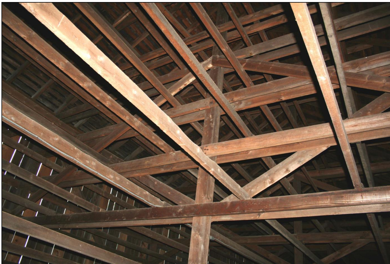
Photograph 27: Barn B (19), interior, detail of transverse cross-bracing.
