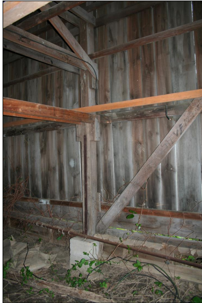
Photograph 80: Barn H (104), interior, detail of post, footing and diagonal wind brace.
