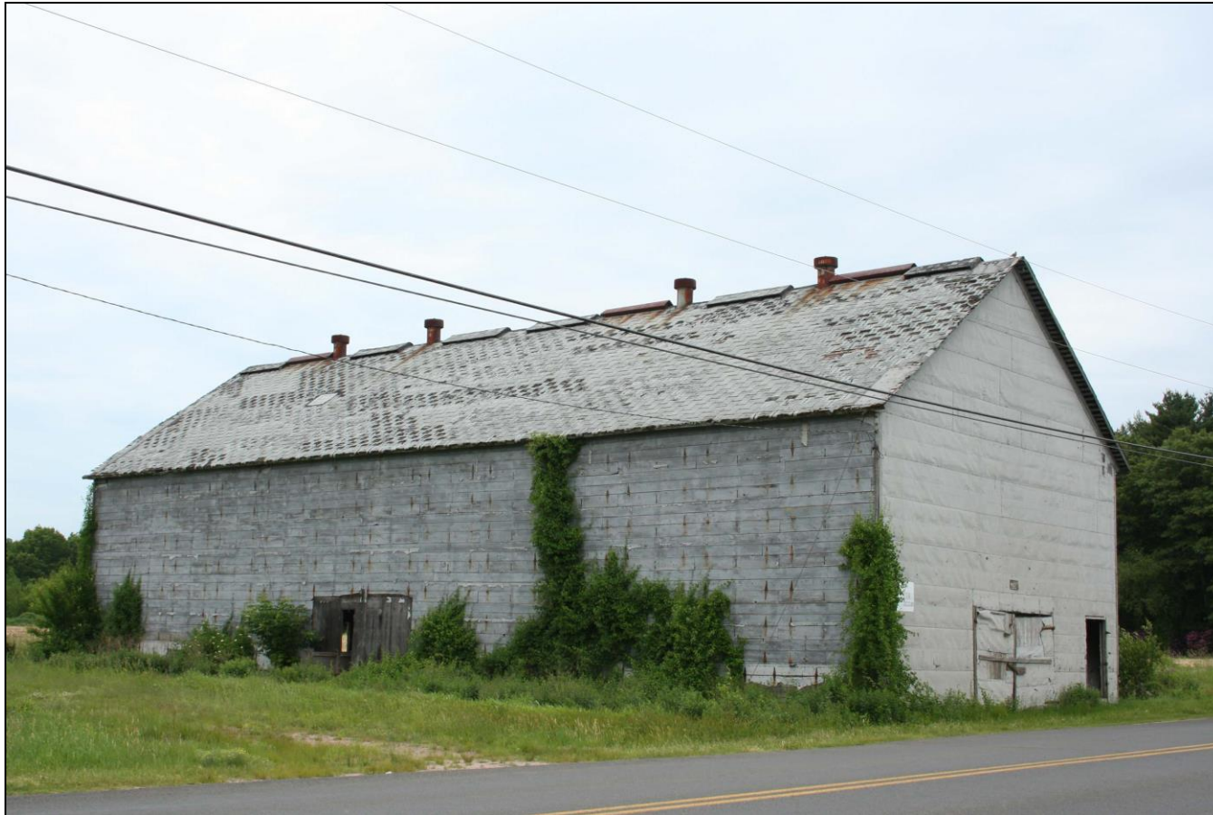
Photograph 126: Barn N (2-16), east and north elevations, camera facing southwest.
