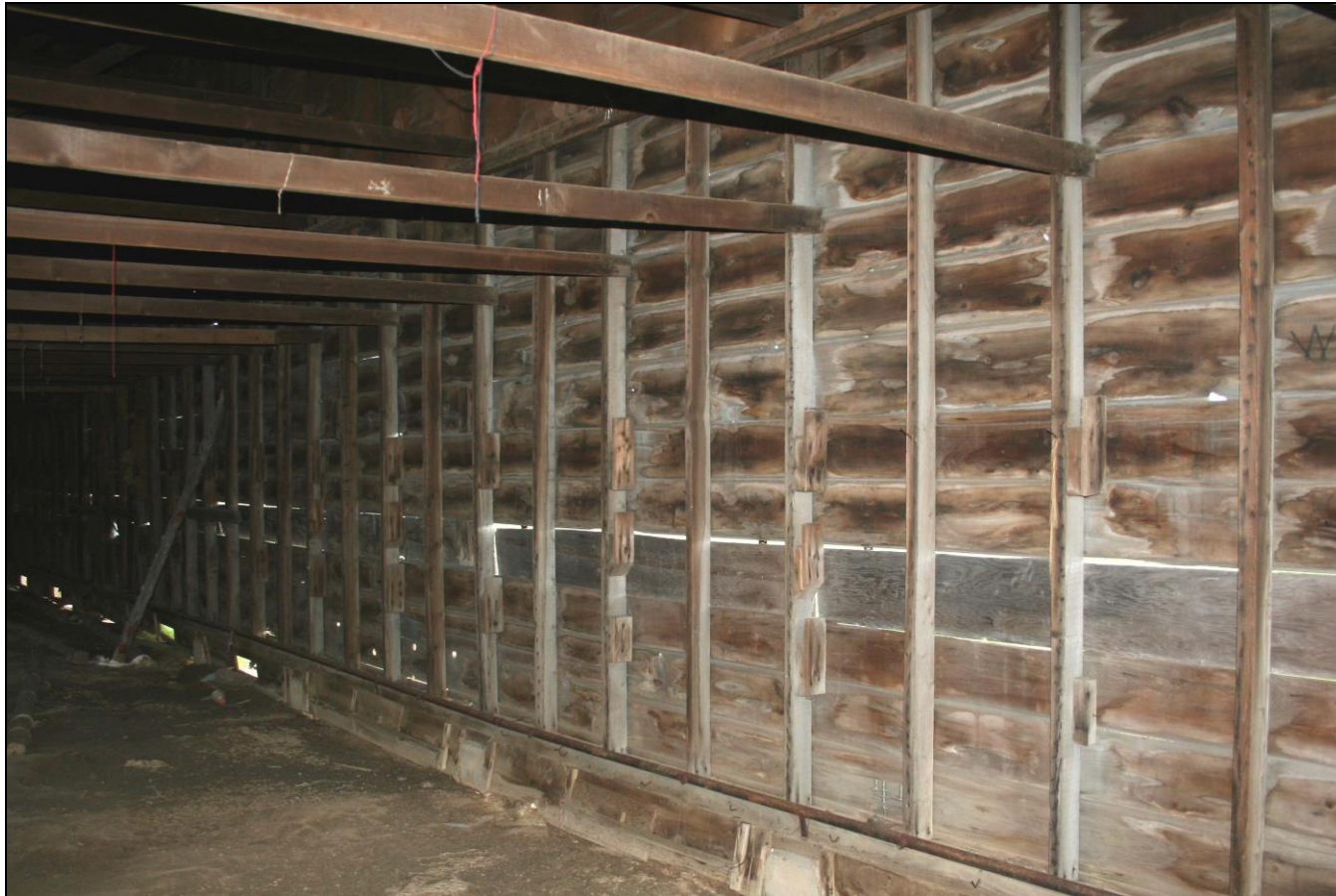
Photograph 49: Barn D (7), interior, detail of balloon-framed walls.
