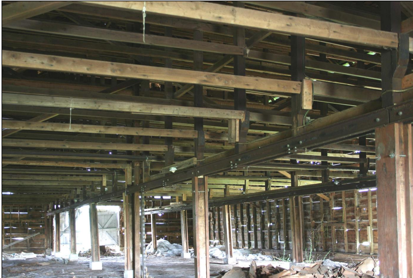
Photograph 100: Barn J, overview of interior from north end.
