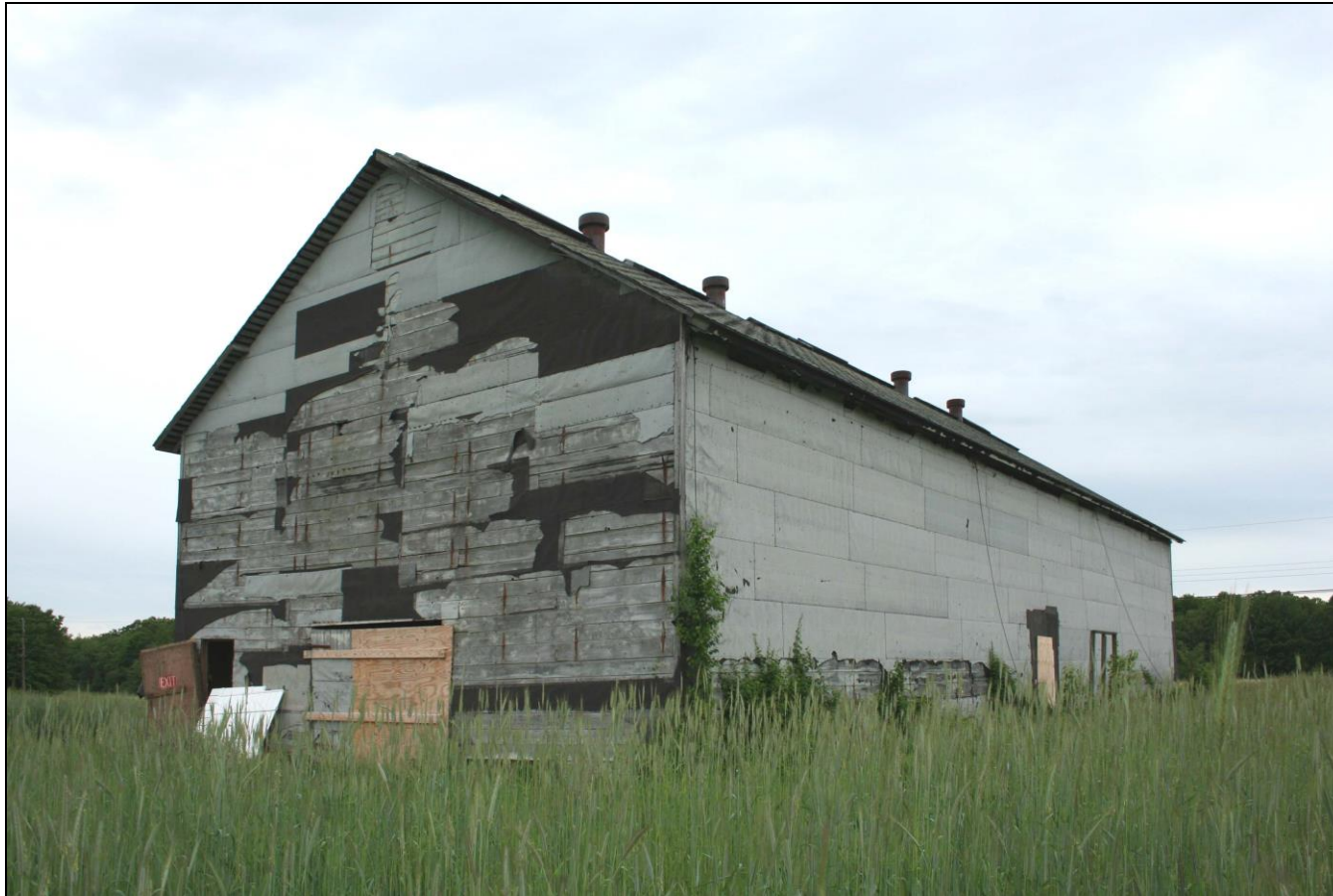
Photograph 89: Barn I, north and west elevations, camera facing south.
