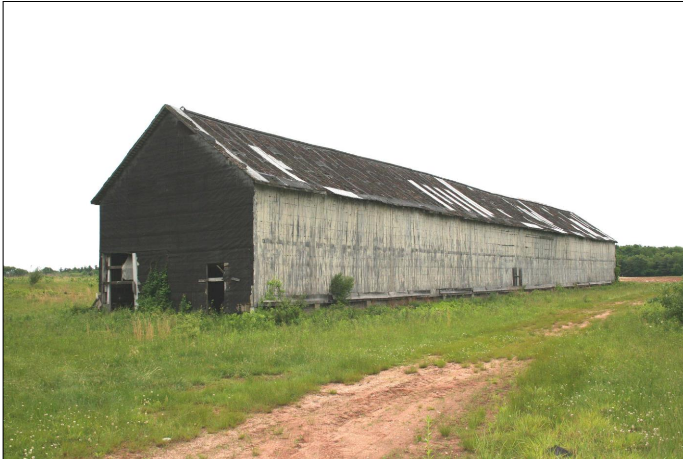
Photograph 70: Barn G (103), north and west elevations, camera facing southeast.
