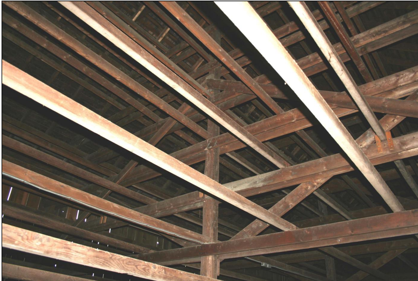
Photograph 37: Barn C (20), interior, detail of cross-bracing.
