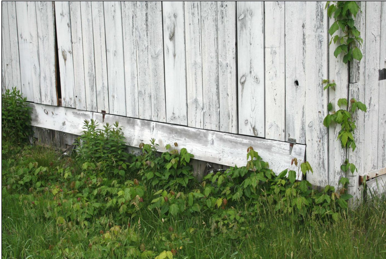
Photograph 23: Barn B (19), detail of hinged board at sill.
