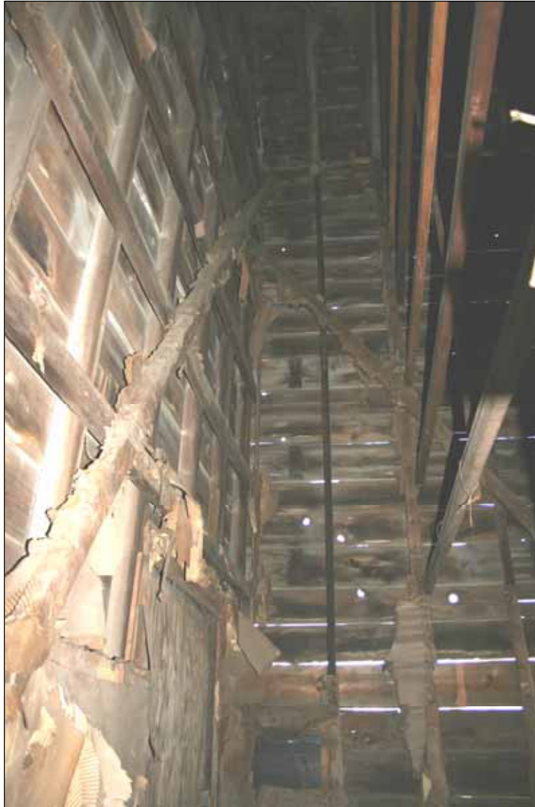
Photograph 38: Detail of typical end-wall and side-wall wind braces (No. 94, northeast corner, camera facing east).
