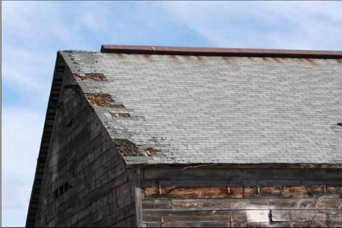
Photograph 32: Detail of sheet-metal ridge ventilator and roof damage, showing wood shingles under current asphalt-shingle roof (No. 92, west elevation, camera facing east).
