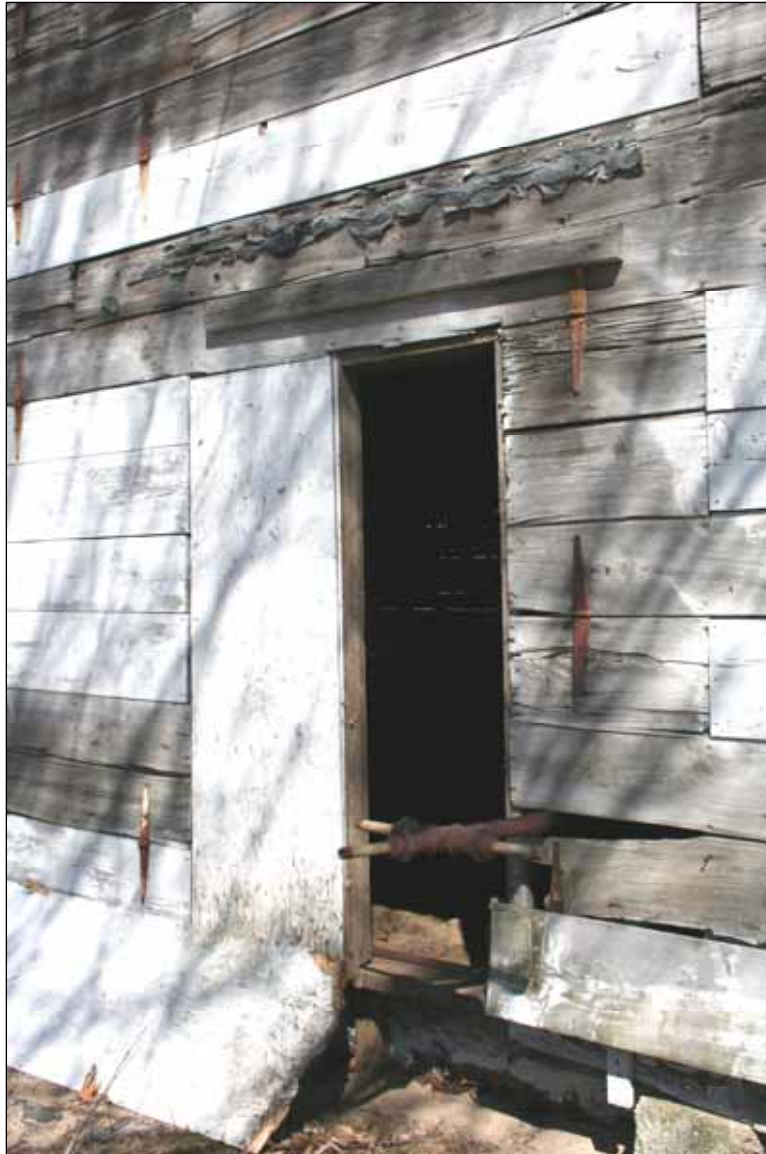
Photograph 29: Detail of side-elevation doorway, blocked off with particle board, with gas fittings exiting on right (No. 94, west elevation, camera facing northeast).
