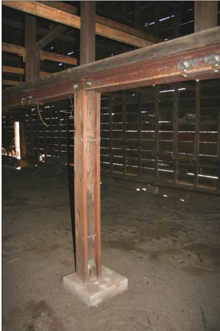
Photograph 36: Detail of typical interior post, showing concrete footing and steel-channel longitudinal member (No. 94, north end, camera facing east elevation, camera facing southwest).
