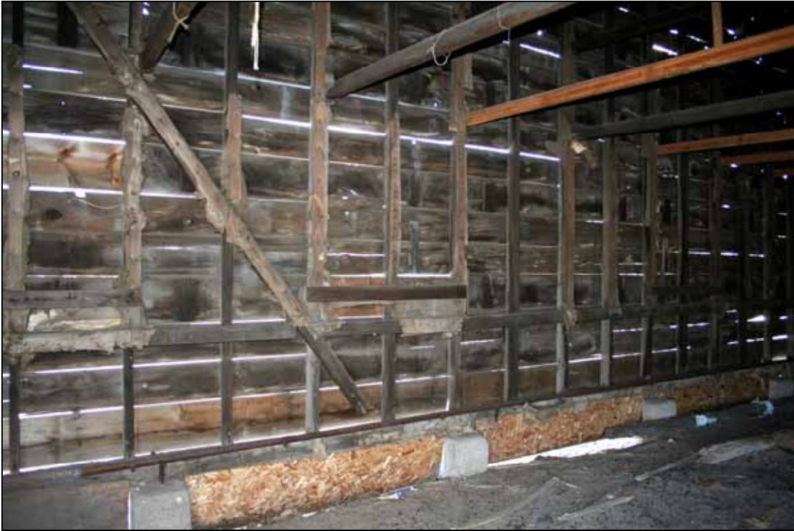
Photograph 37: Detail of typical side-wall construction, showing diagonal end wind brace (No. 94, east wall, north end, camera facing east).
