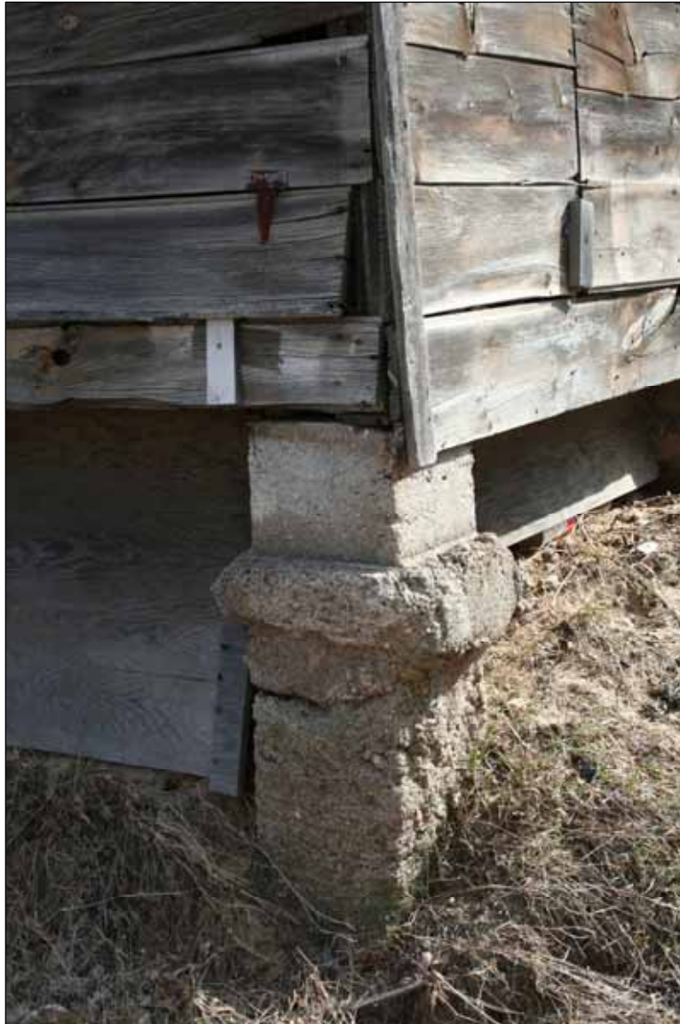
Photograph 34: Detail of eroded concrete foundation pier, showing lower portion, formerly embedded in the ground, exposed (No. 91, southwest corner, east elevation, camera facing northeast).
