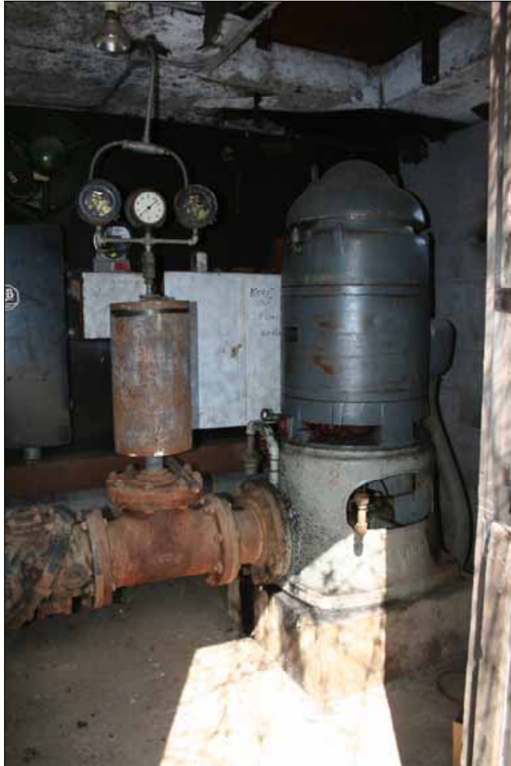
Photograph 53: Pump house, interior, U.S. Electric Motors motor and Deming pump on right, camera facing northwest.
