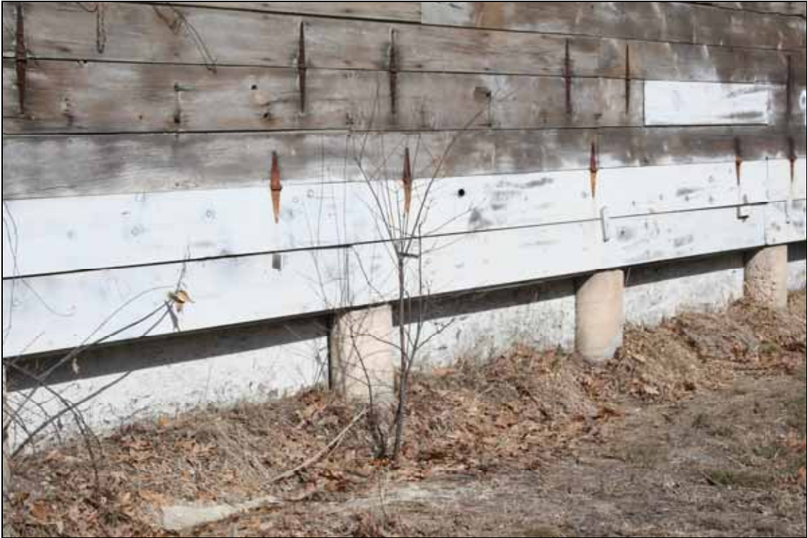
Photograph 35: Detail of replaced foundation piers, north end of No. 90, east elevation, camera facing northwest.
