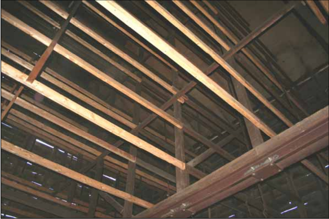
Photograph 39: Detail of typical cross-members forming tiers for hanging tobacco (No. 94, north end, camera facing southwest).
