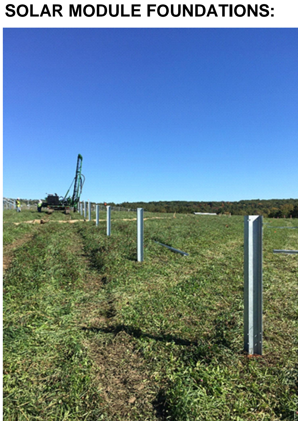
ABOVE IS A PHOTO REPRESENTING THE THE PROPOSED METHOD OF PILE DRIVING FOR THE SOLAR FACILITY. IMPACTS TO THE SUBSURFACE SOIL IS MINIMAL, AND NOT INCLUDED IN THE PROPOSED IMPERVIOUS AREAS FOR THE AREA WITHIN THE UPLAND HABITAT.
