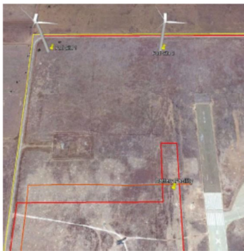
Large scale wind farm technology facility in Texas Tech University
