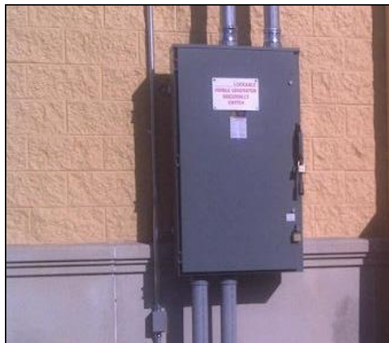
Figure 2: Electrical Disconnect
