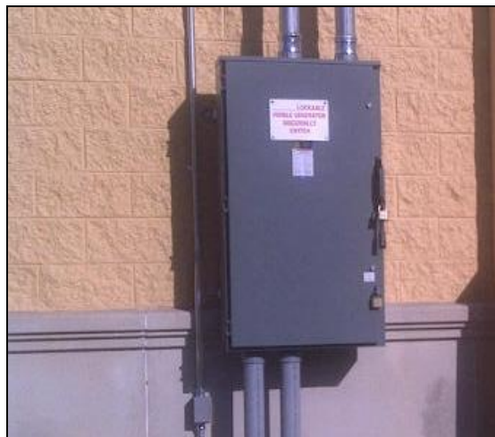
Figure 2: Electrical Disconnect
