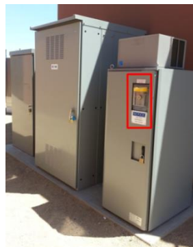
Figure 3 – Telemetry Cabinet & EPO Button
