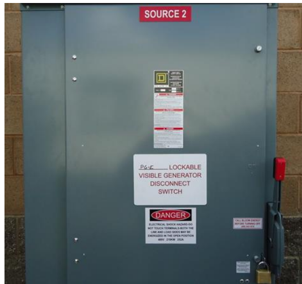
Figure 5 – Electrical Disconnect Switch
