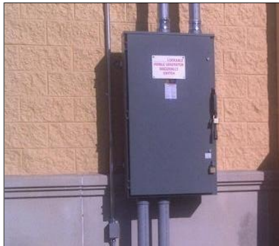
Figure 2: Electrical Disconnect
