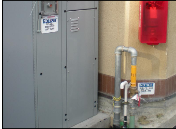
Figure 3: Manual Natural Gas Valve
