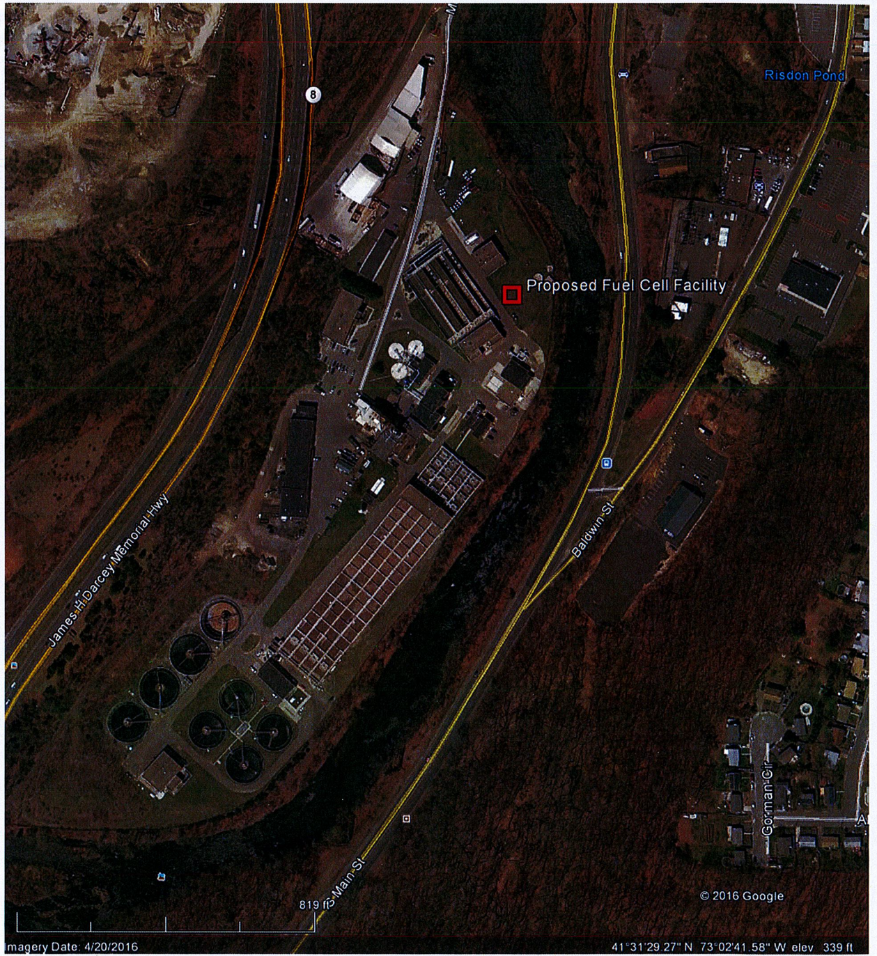
Location of proposed project - Waterbury Water Pollution Control Plant
