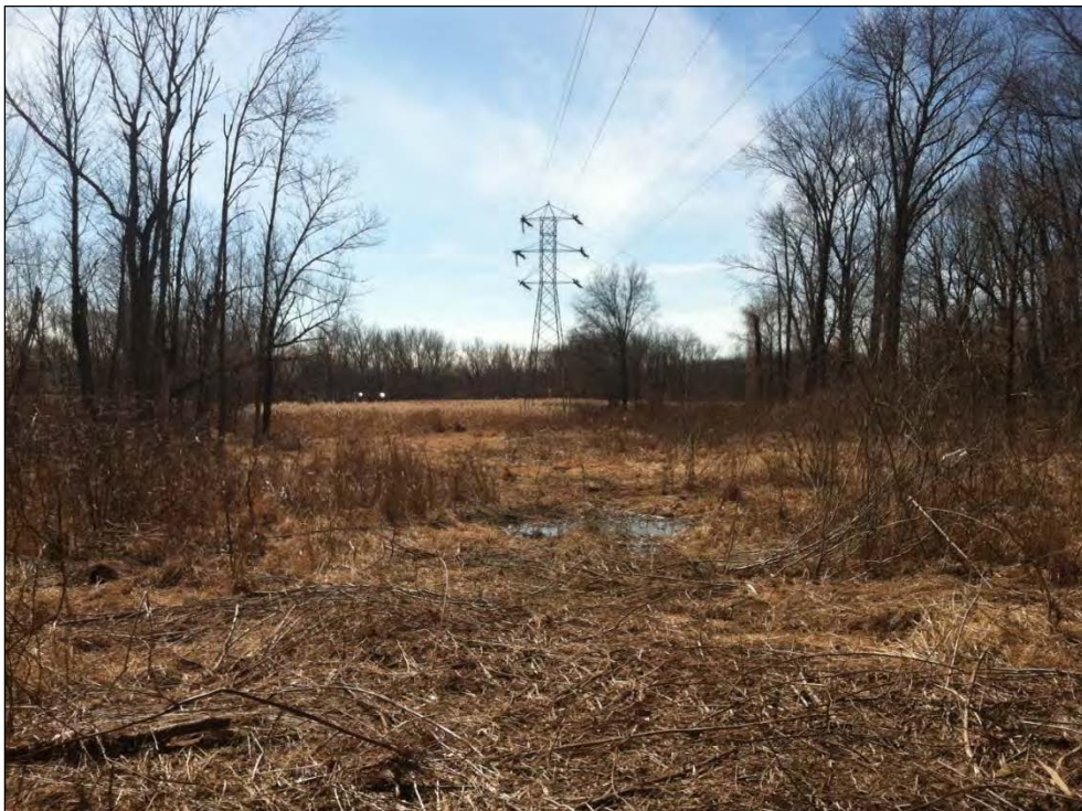
Photo 6 – 3/19/2016: View facing southwest of Wetland W-8 from existing access road. Existing structure 3018 is in the background.
