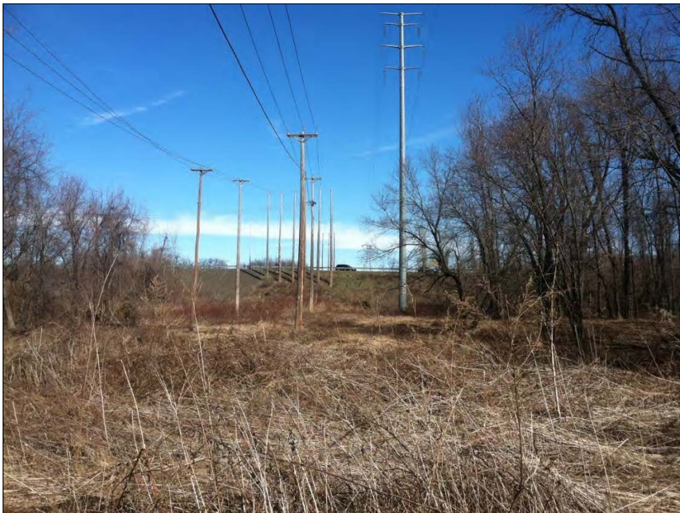
Photo 2 – 3/19/2016: View facing northeast of Wetland W-1. Existing structure 3002 is in background.
