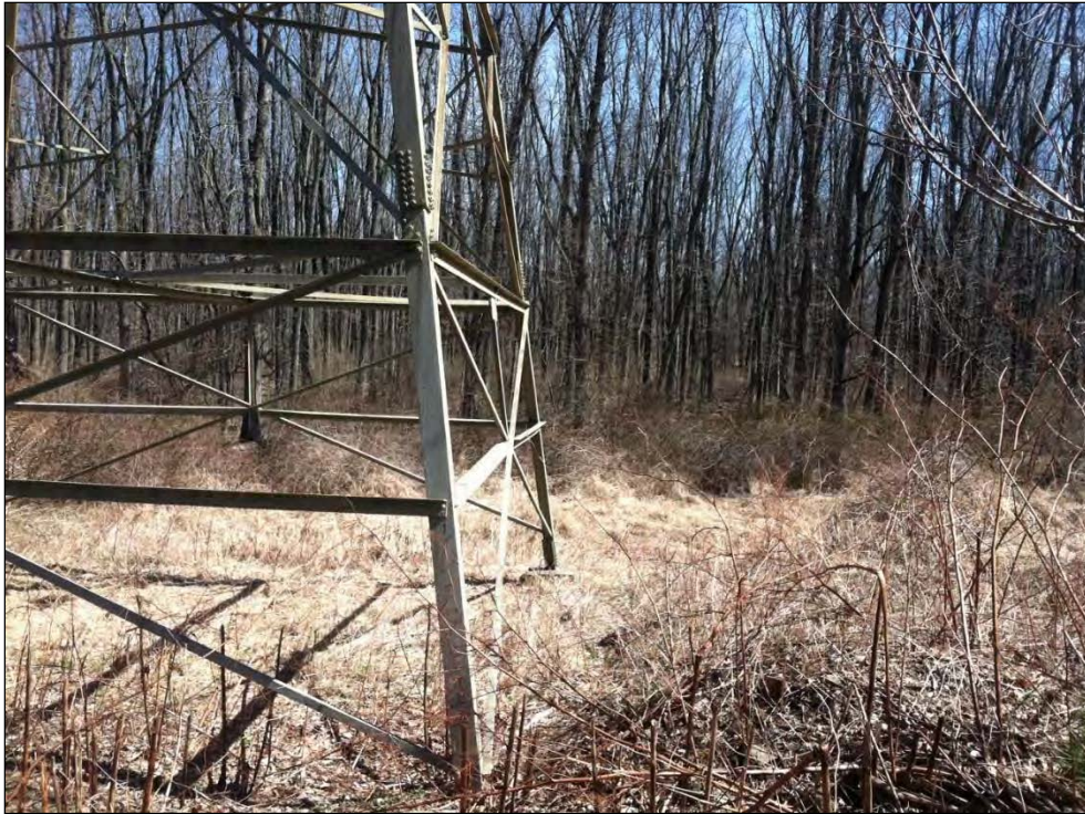
Photo 5 – 3/19/2016: View facing east of Wetland W-7 and existing structure 3013.
