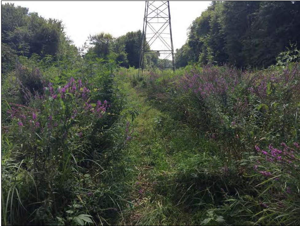
Photo 7 – 8/6/2015: View facing north of existing structure 3025 in Wetland W-9.
