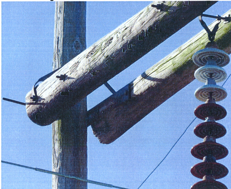
Figure H- 4 Pole and Cross Arm Hardware
