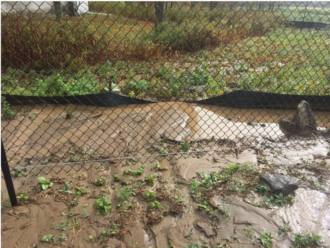
Photo 8: View of sediment build-up and discharge from channel erosion looking east (Maintenance Action Item #1).
