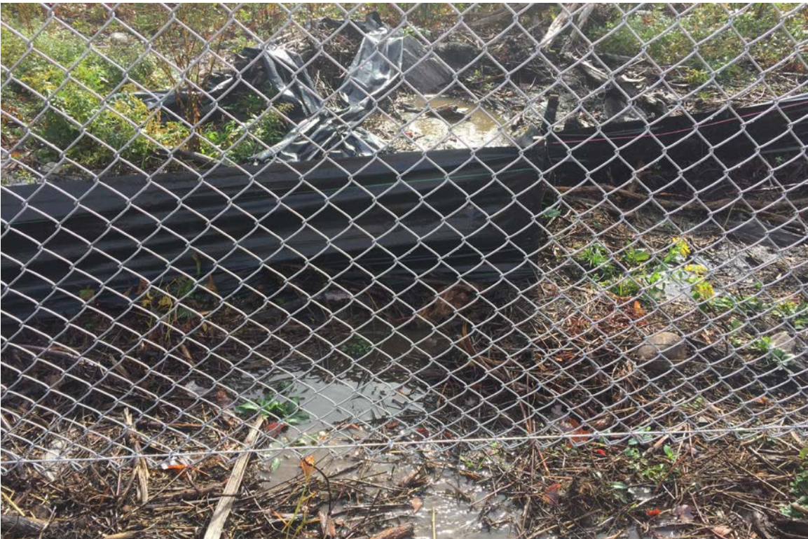
Photo 4: View of silt fence requiring repair (Maintenance Action Item #3).
