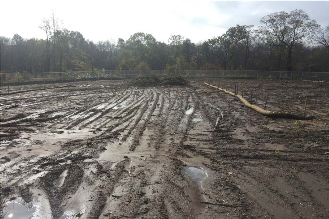
Photo 3: View of unprotected soil stockpile looking south (Maintenance Action Item #6).
