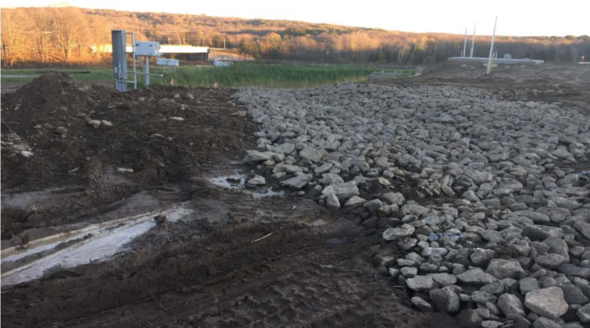
Photo 2: View of access road cross drainage from ponding water (Maintenance Action Item #2).
