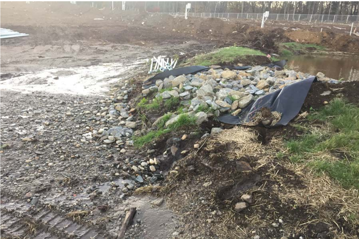
Photo 8: View of southwest temporary sediment trap outfall looking south (Maintenance Action Item #3).
