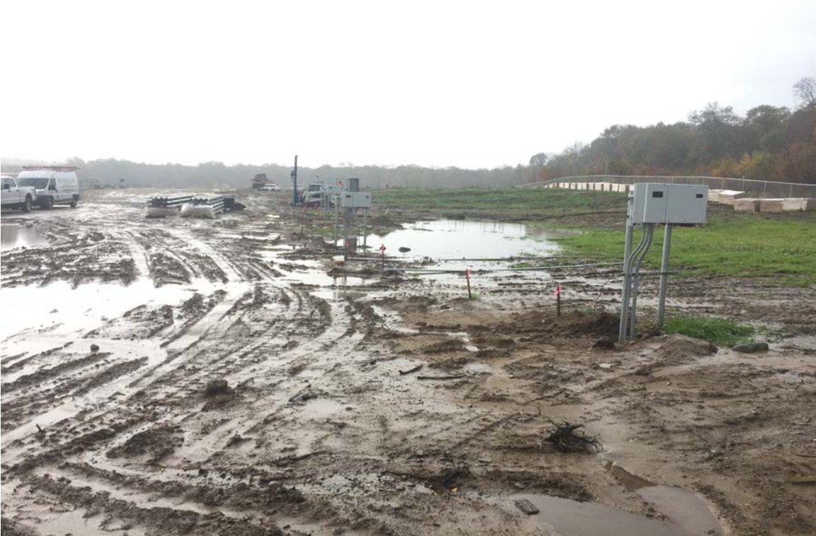
Photo 5: View of ponding water looking west across access (Maintenance Action Item #2).
