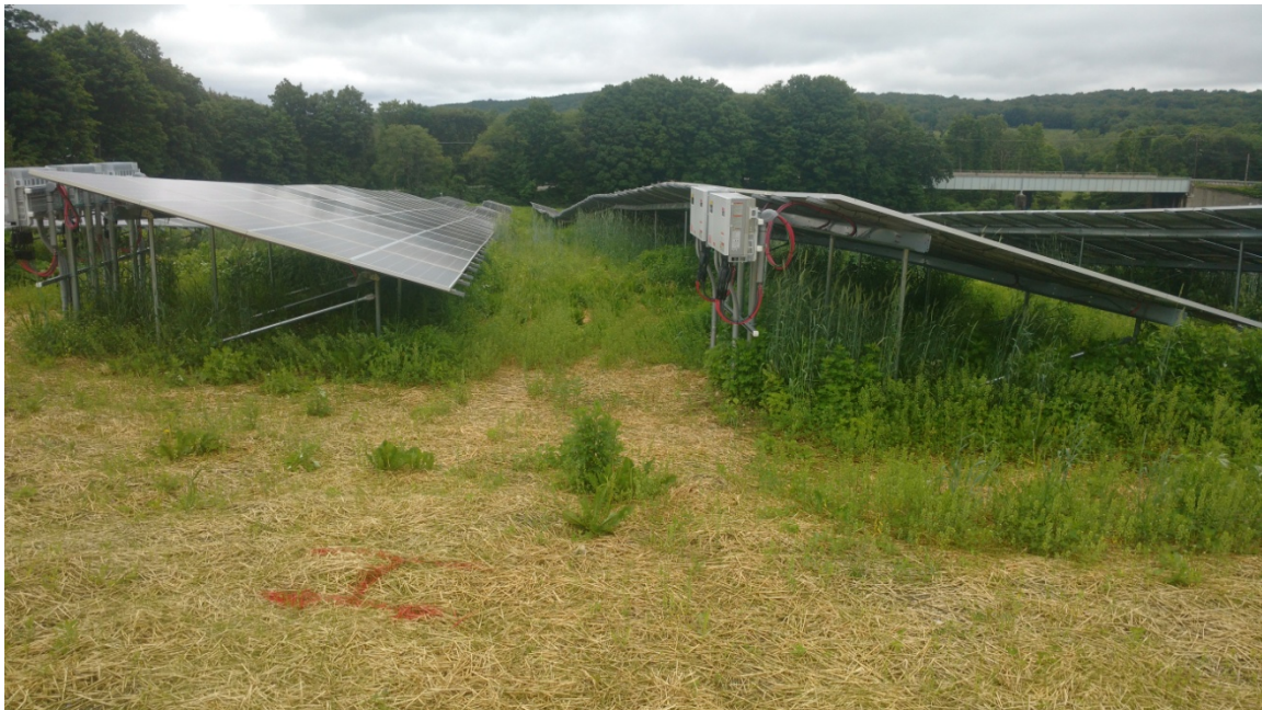
Photograph 4 – combination of straw mulch and volunteer vegetation between solar panels
