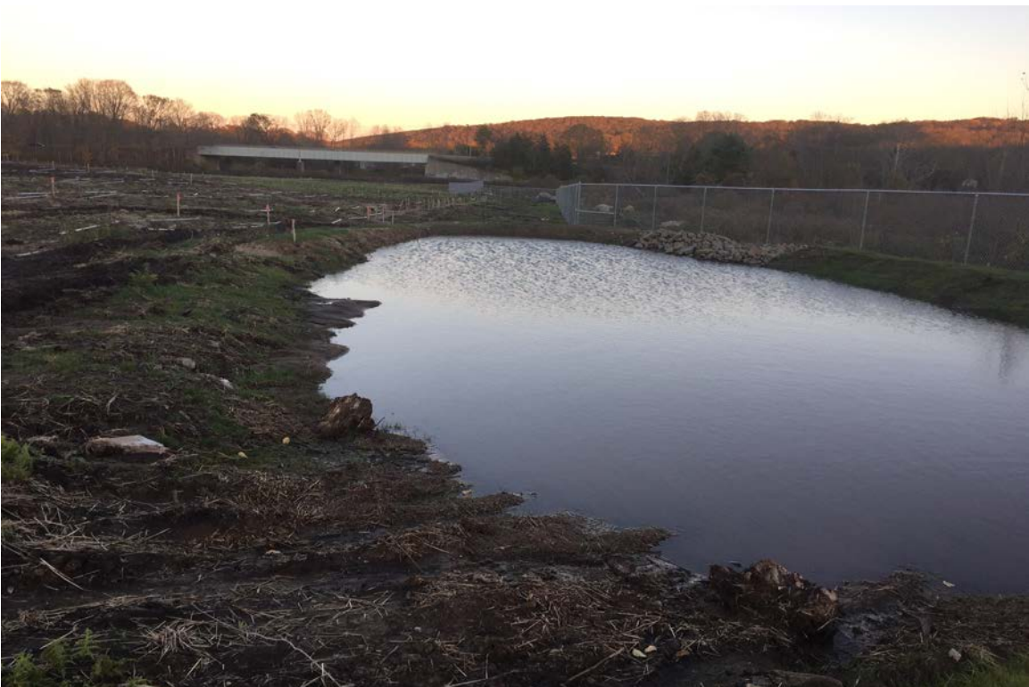
Photo 6: View of southwest temporary sediment trap looking northeast.
