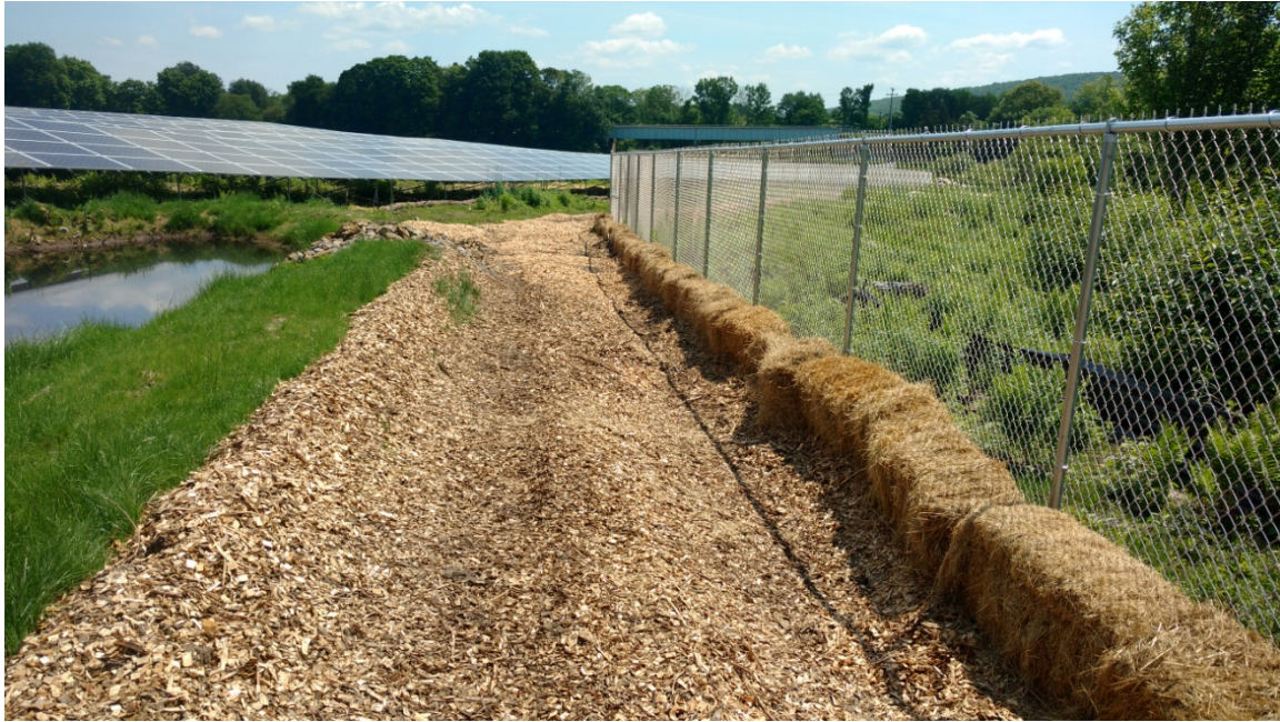
Photograph 2 – Hay bale/woodchip barrier along southern perimeter
