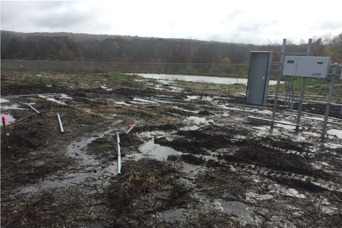
Photo 9: View of southeast temporary sediment trap and discharge into trap looking east (Maintenance Action Item #3).
