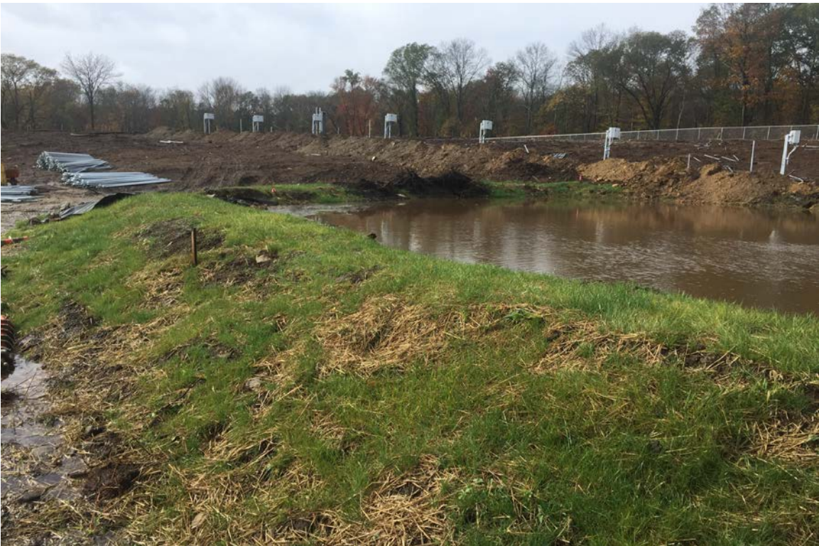
Photo 10: View of southwest temporary sediment trap looking south.
