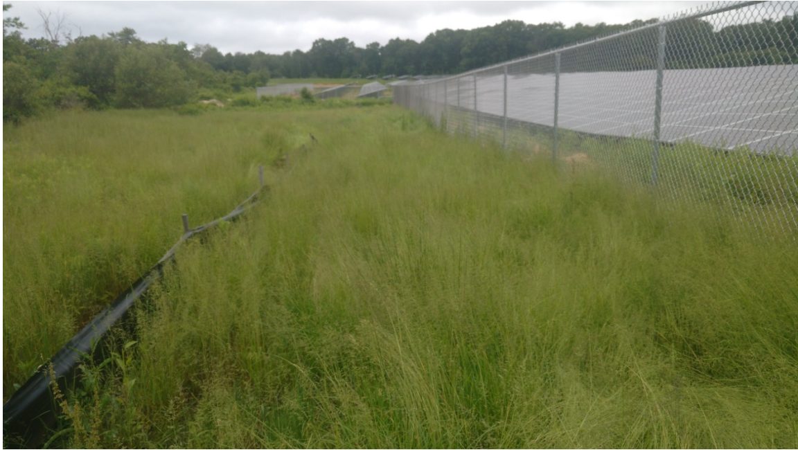
Photograph 3 – combination of hydro seed and volunteer vegetation at the down slope edge of the site
