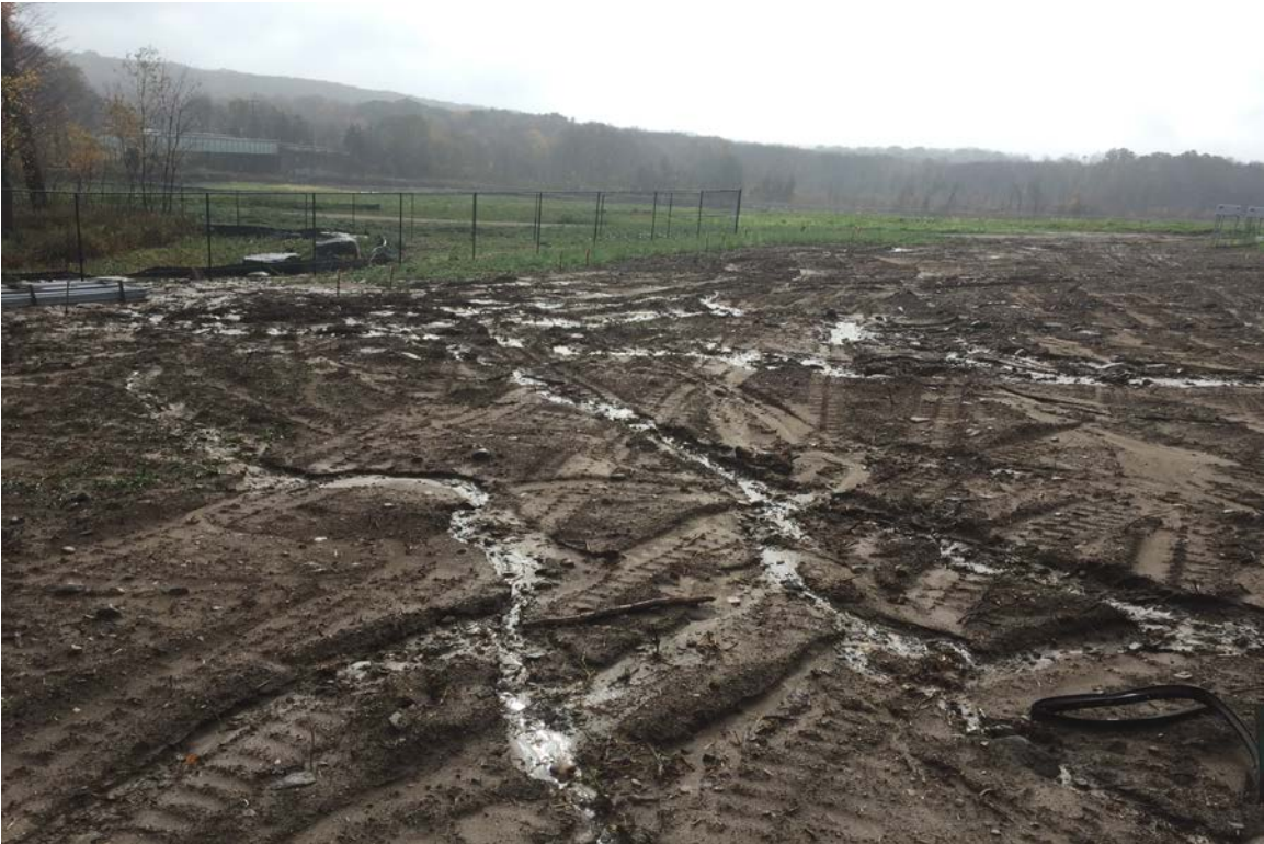
Photo 7: View of channel erosion looking east (Maintenance Action Item #1).
