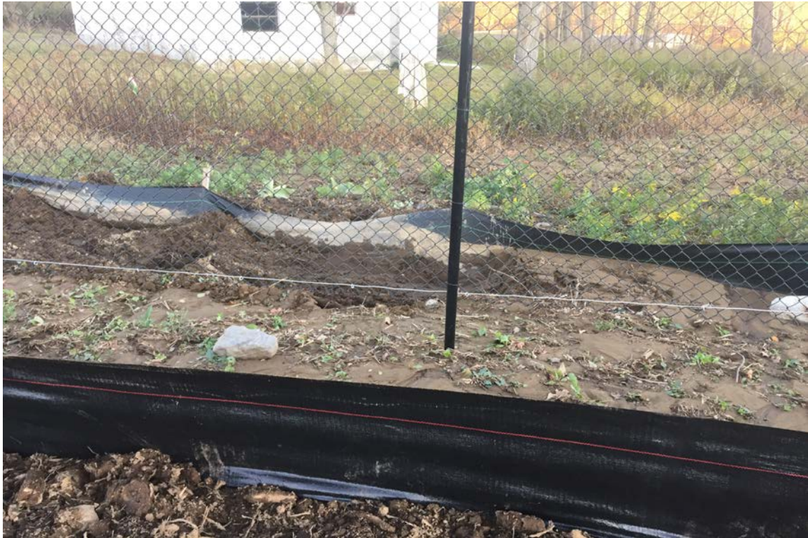
Photo 3: View of sediment accumulation at silt fence from channel erosion looking east (Maintenance Action Item #1).
