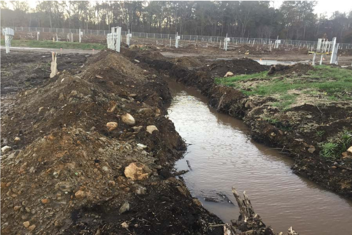
Photo 5: View of unprotected open trenches (Maintenance Action Item #5).
