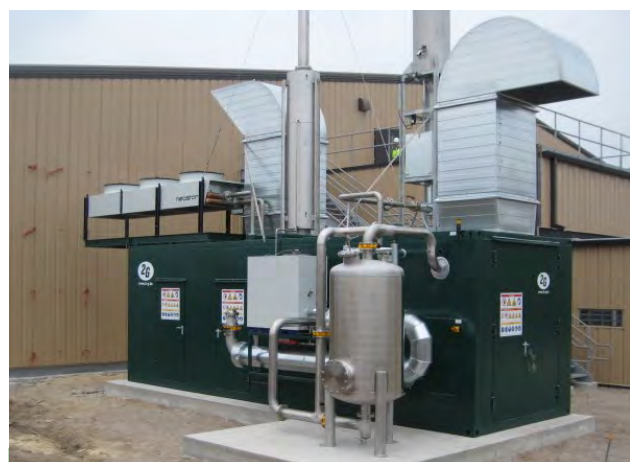
Municipal Dry Anaerobic Digester Biogas CHP Power Generation Plant with “Plug & Play” Container Module, including Gas Conditioning & Treatment System.
