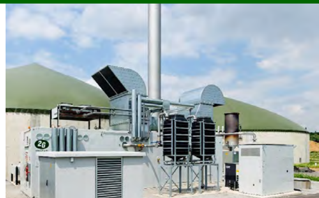
Anaerobic Farm Digester Biogas CHP Power Generation Plant with “Plug & Play” Container Module.
