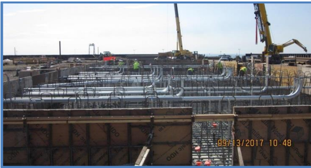
Installed Conduits in the CTG Foundation
