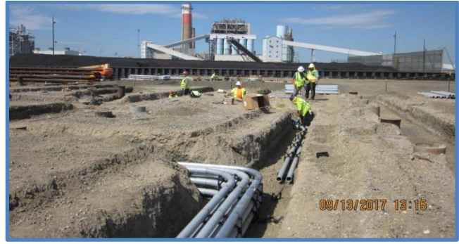
Admin Building Ductbank Conduits Being Installed
