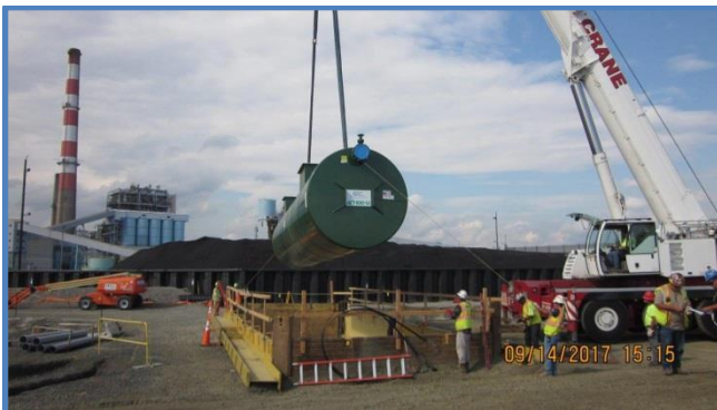
Installing Oily Water Separator
