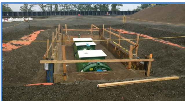
Oily Water Separator Installed
