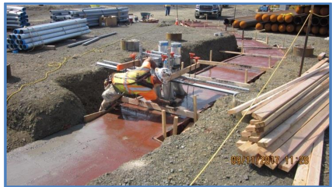
Finishing Aux transformer Ductbanks
