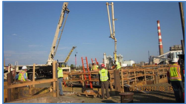
Pouring Walls at Spent Slurry Sump
