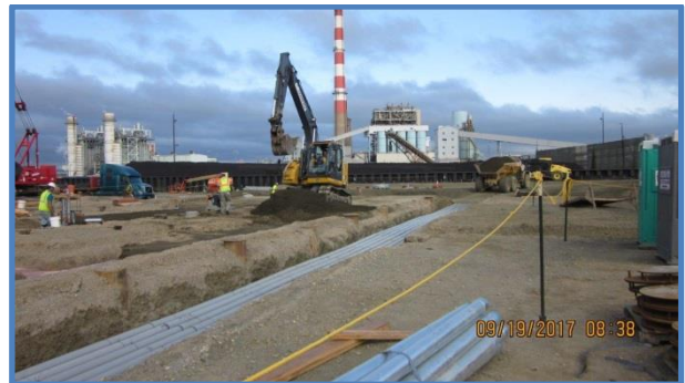
Admin Building Ductbank Conduits Being Installed
