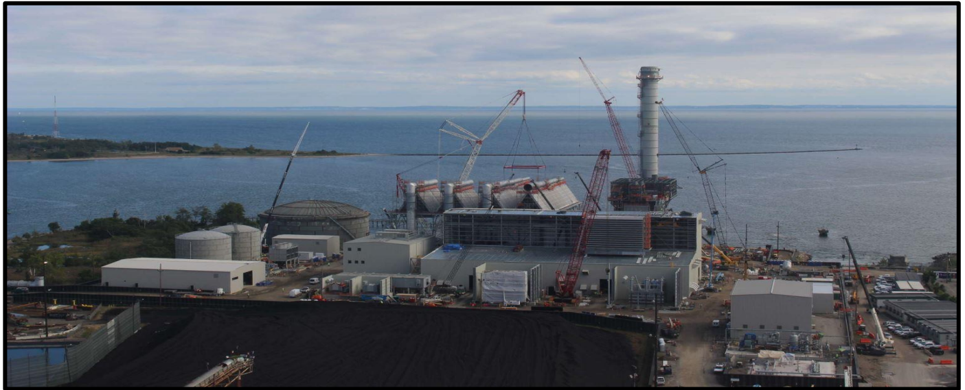
Site Progress Photo 9/27/2018
