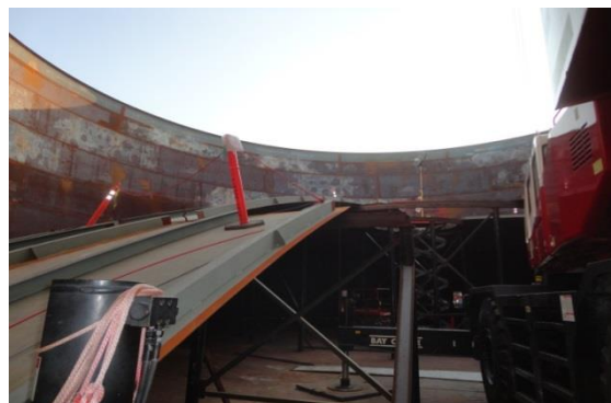
ULSD Tank Roof Erection
