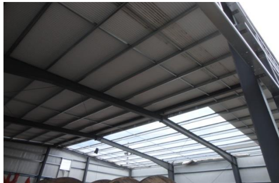
Warehouse Roof Installation
