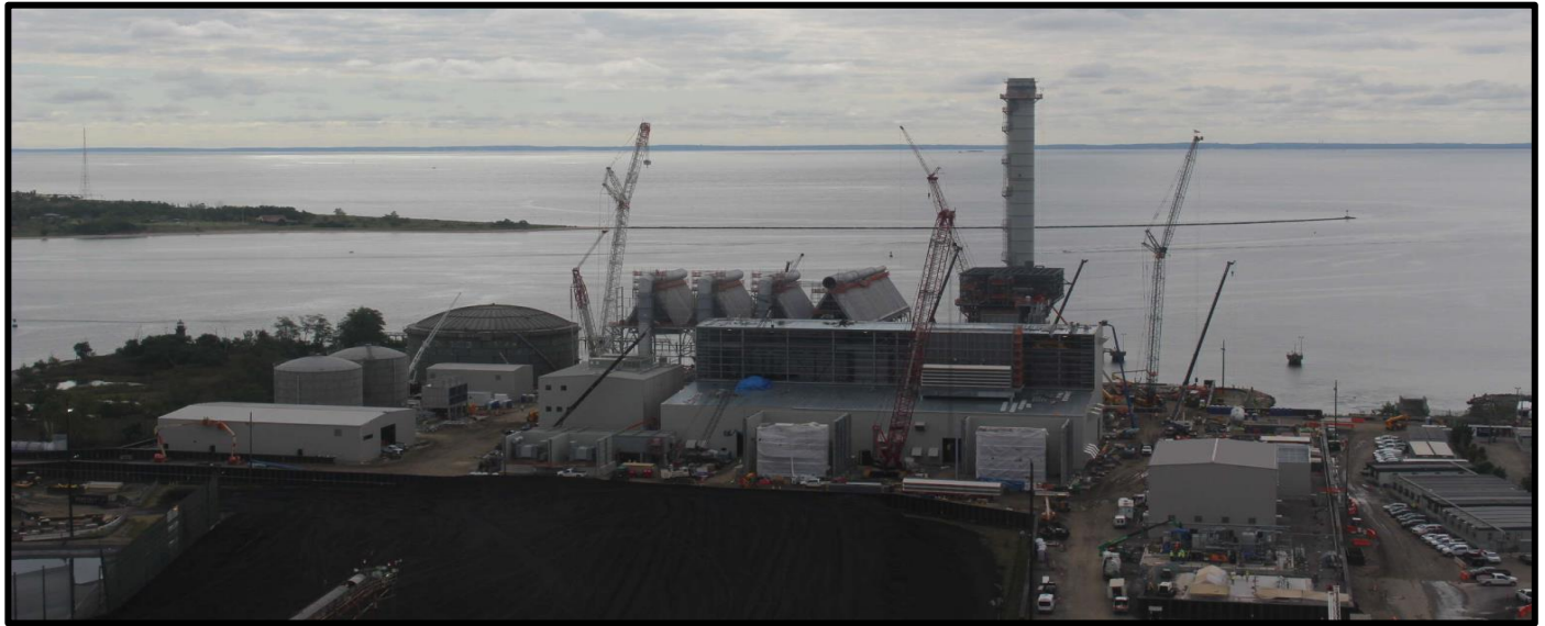
Progress Photos Site Progress Photo 9/20/2018
