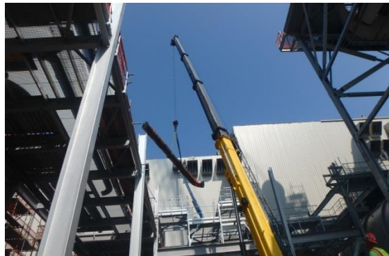
Setting Pipe Spools in Pipe Rack
