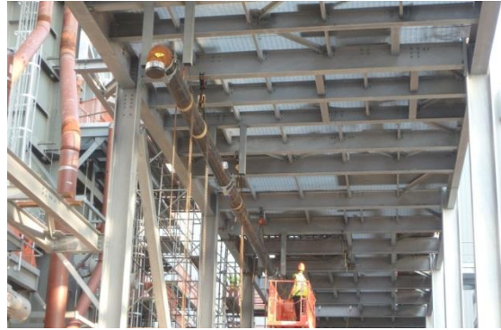
Installing Condensate Piping
