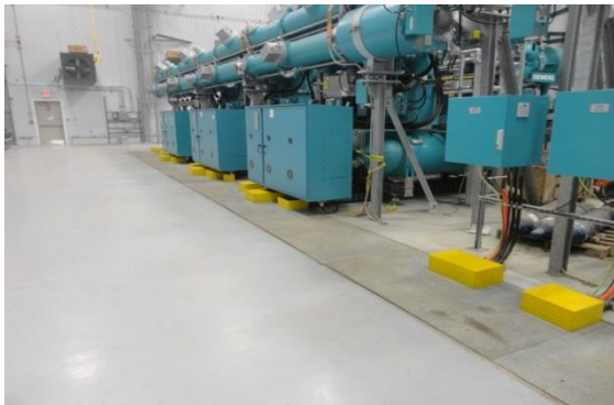
Completed Trench Covers in GIS
