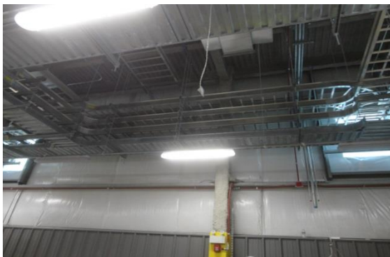
Cable Tray Installation in Admin Building
