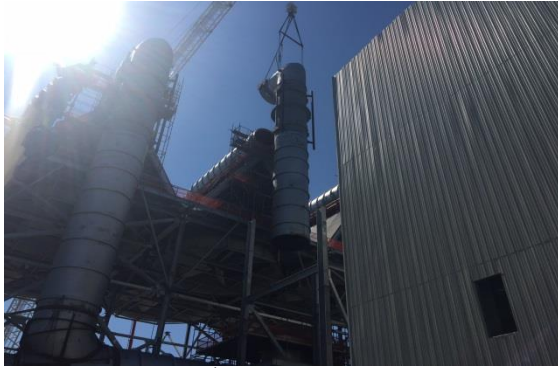
Setting 3 rd ACC Riser (Street #2)
