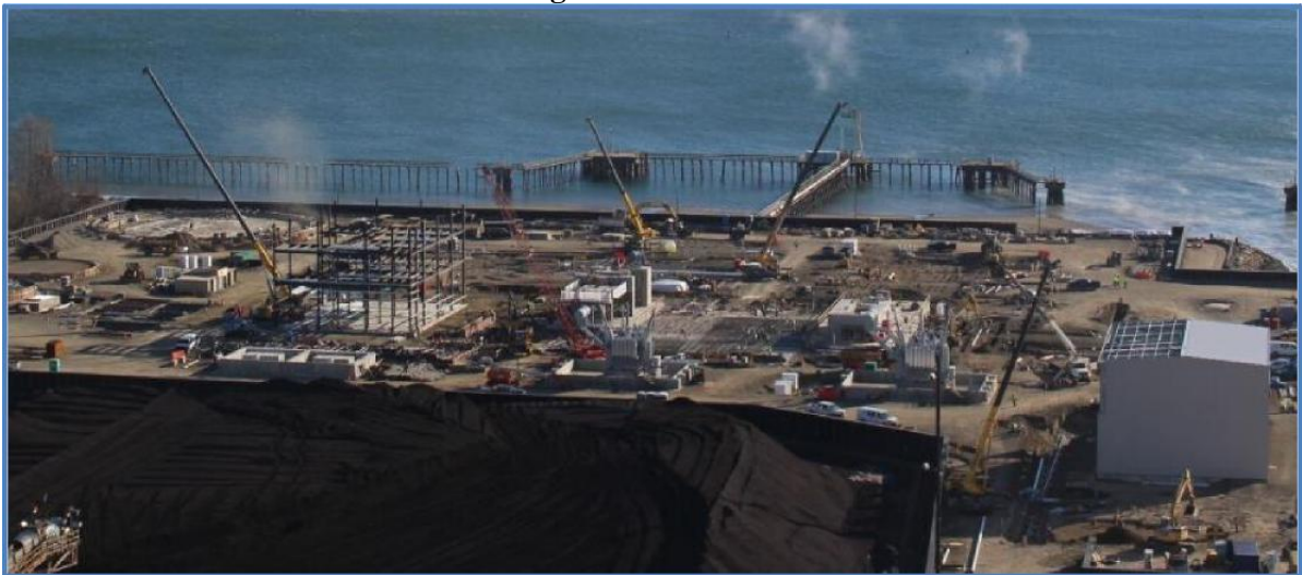
Site Progress Photo 12-28-2017
