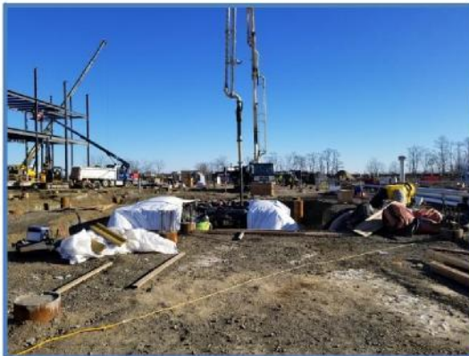
Pouring the ACC Drain Pot Sump
