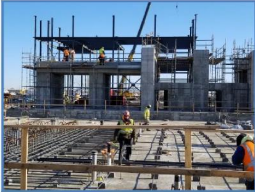
Turbine Building Foundation & ST Pedestal Work
