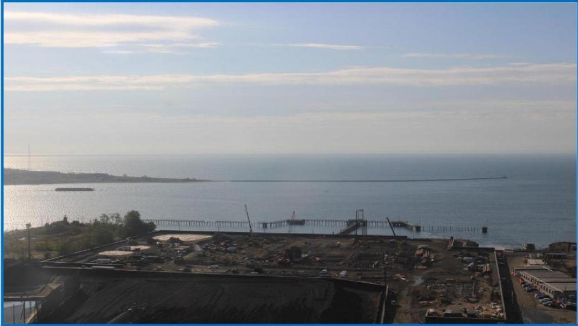
Site Progress Photo 10-05-17
