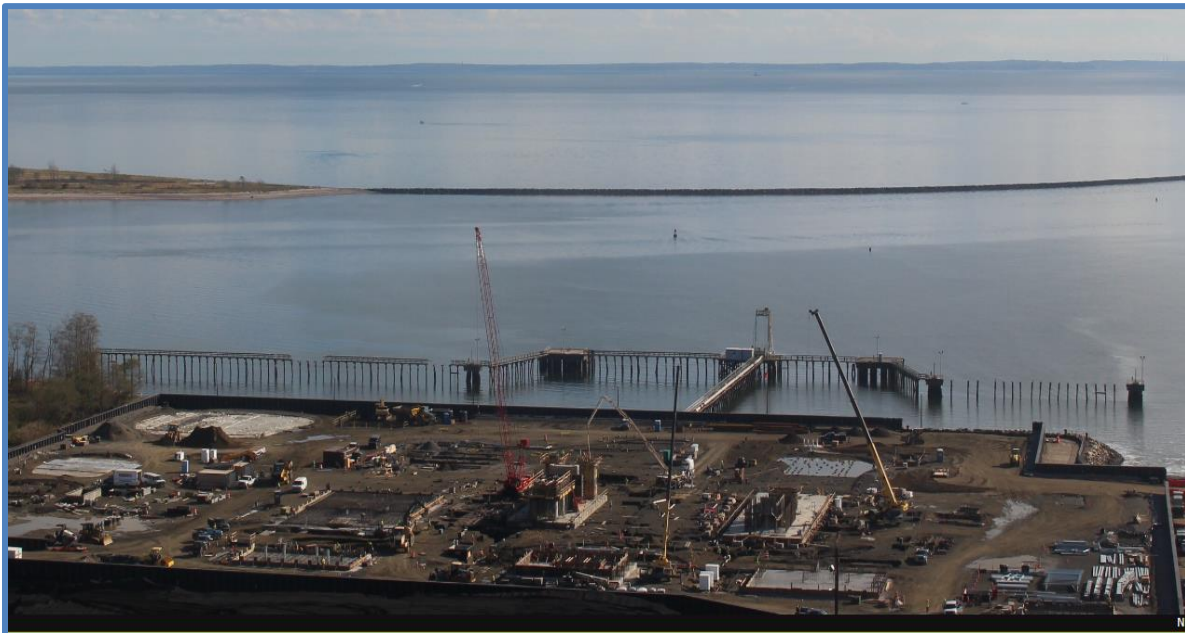
Site Progress Photo 11-02-17
