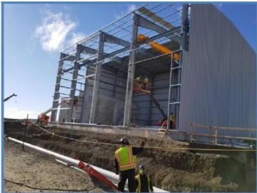
GIS Building Erection
