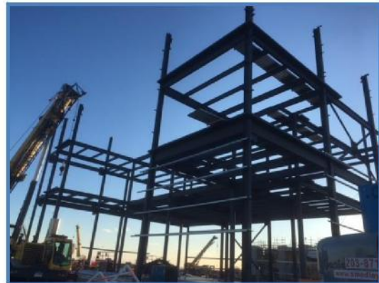
Admin Building Erection
