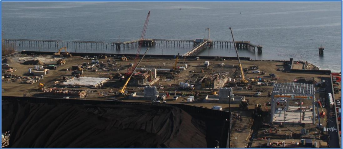
Site Progress Photo 11-30-17
