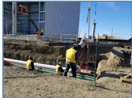
Underground Piping Next to GIS Building
