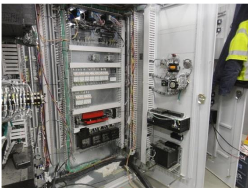
Generator Protection Panel Terminations
