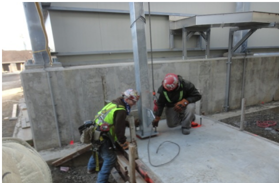
MVPDC Access Steel Erection
