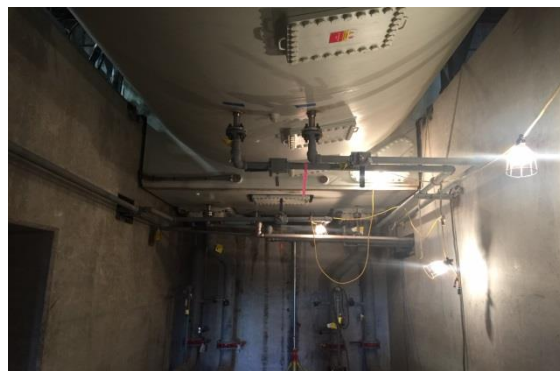
Hydrogen Piping Under CTG
