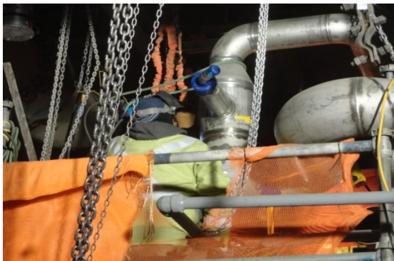
Steam Turbine Lube Oil Piping
