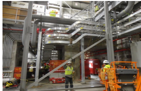
STG Iso-Phase Steel Erection
