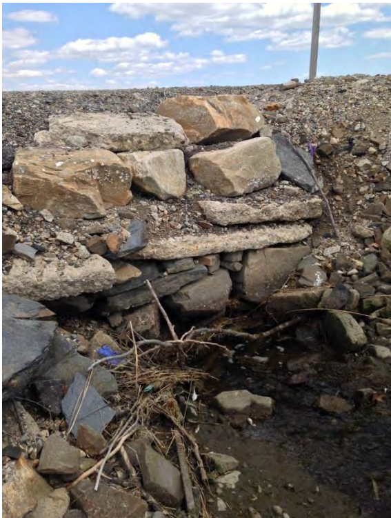
Culvert on east side connecting wetland to harbor.
