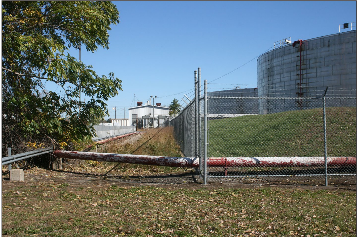
View of northwestern corner of the proposed combined cycle project site looking east. The existing aboveground storage tanks and their earthen containment berm can be seen in the photograph 1
