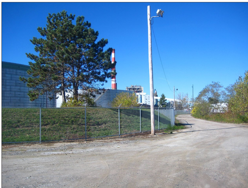
View of eastern edge of proposed combined cycle project site looking north from the site's southeastern corner 4
