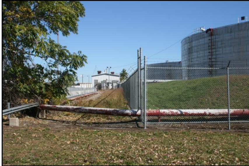
Photo 1. View of northwestern corner of the proposed combined cycle project site looking east. The existing aboveground storage tanks and their earthen containment berm can be seen in the photograph.
