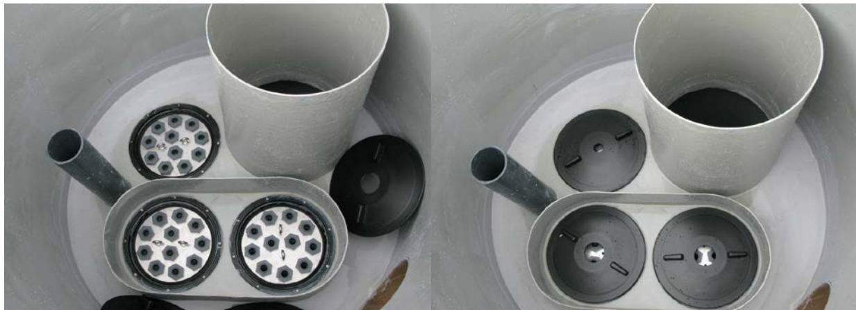
Figure 7 Top view photos of the Jellyfish ® Filter JF4-2-1 deck with two hi-flo cartridges and one draindown cartridge installed with cartridge lids off (upper left image) and cartridge lids on (upper right image). The backwash pool weir encloses the hi-flo cartridge. Also shown are the maintenance access pipe (large), pressure relief pipe (small), and the outlet opening (lower right in each image).
