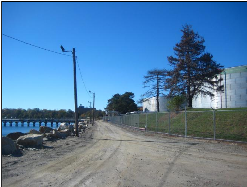
Photo 3. View of southern edge of proposed combined cycle project site looking east.
