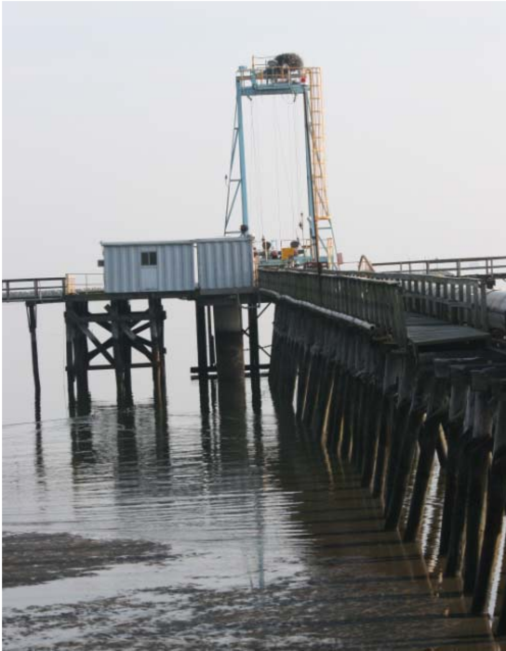
Bridgeport Harbor Station Oil Dock – Center Breasting Dolphin March 8, 2016 Looking south
