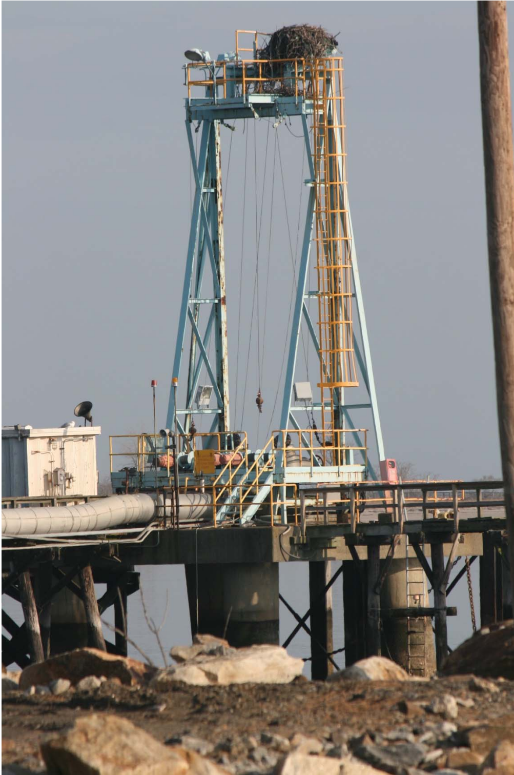
Bridgeport Harbor Station Oil Dock – Center Breasting Dolphin March 8, 2016 Looking Southeast
