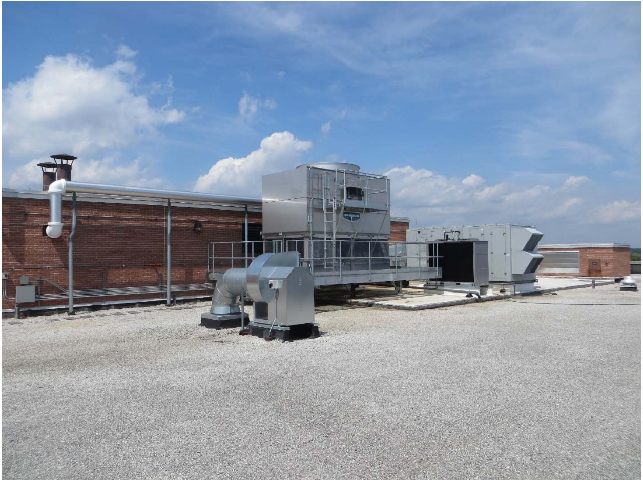
208 Harbor Drive: Existing Cooling Tower
