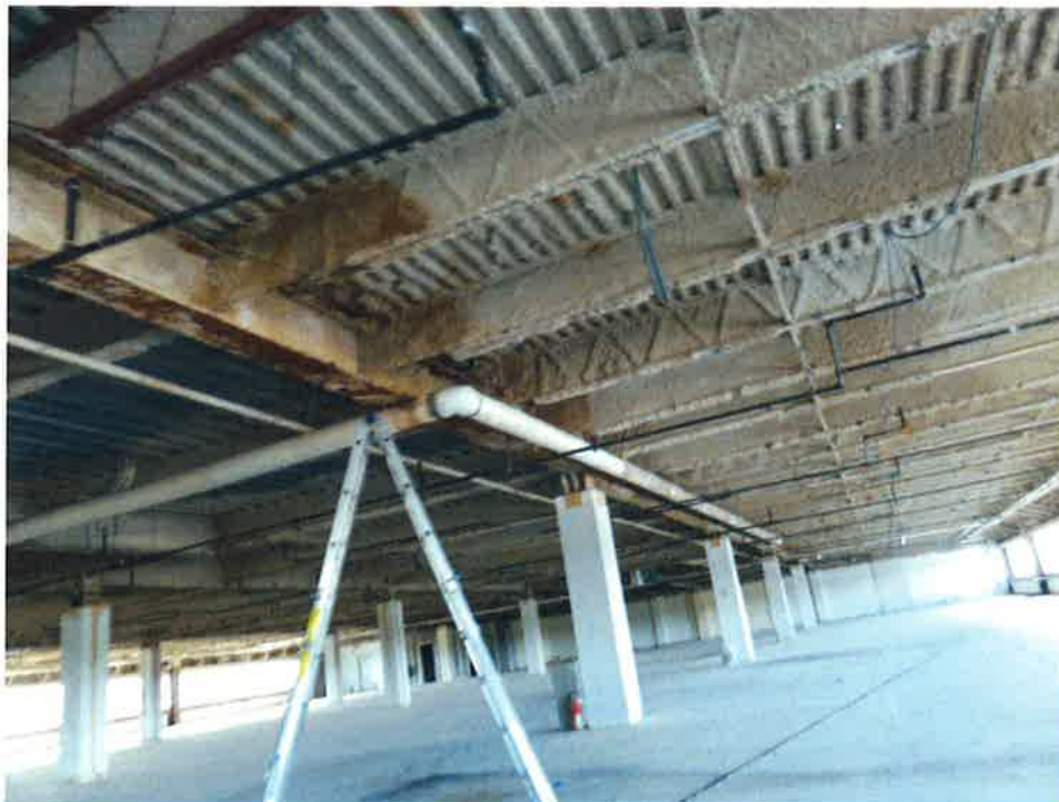
Photo 4: Sample photo illustrating the existing roof construction.
