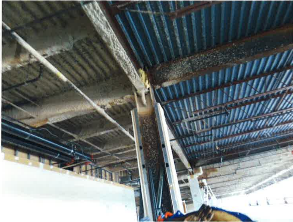
Photo 3: Sample photo illustrating the existing roof construction.
