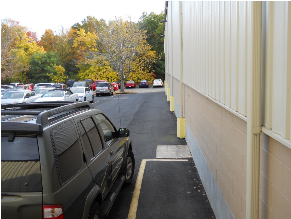
LOCATION OF PROPOSED FACILITY VIEW FROM WEST TO EAST
