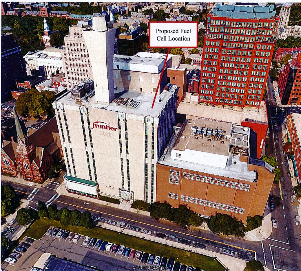
View of site, Frontier Building, 310 Orange Street, New Haven
