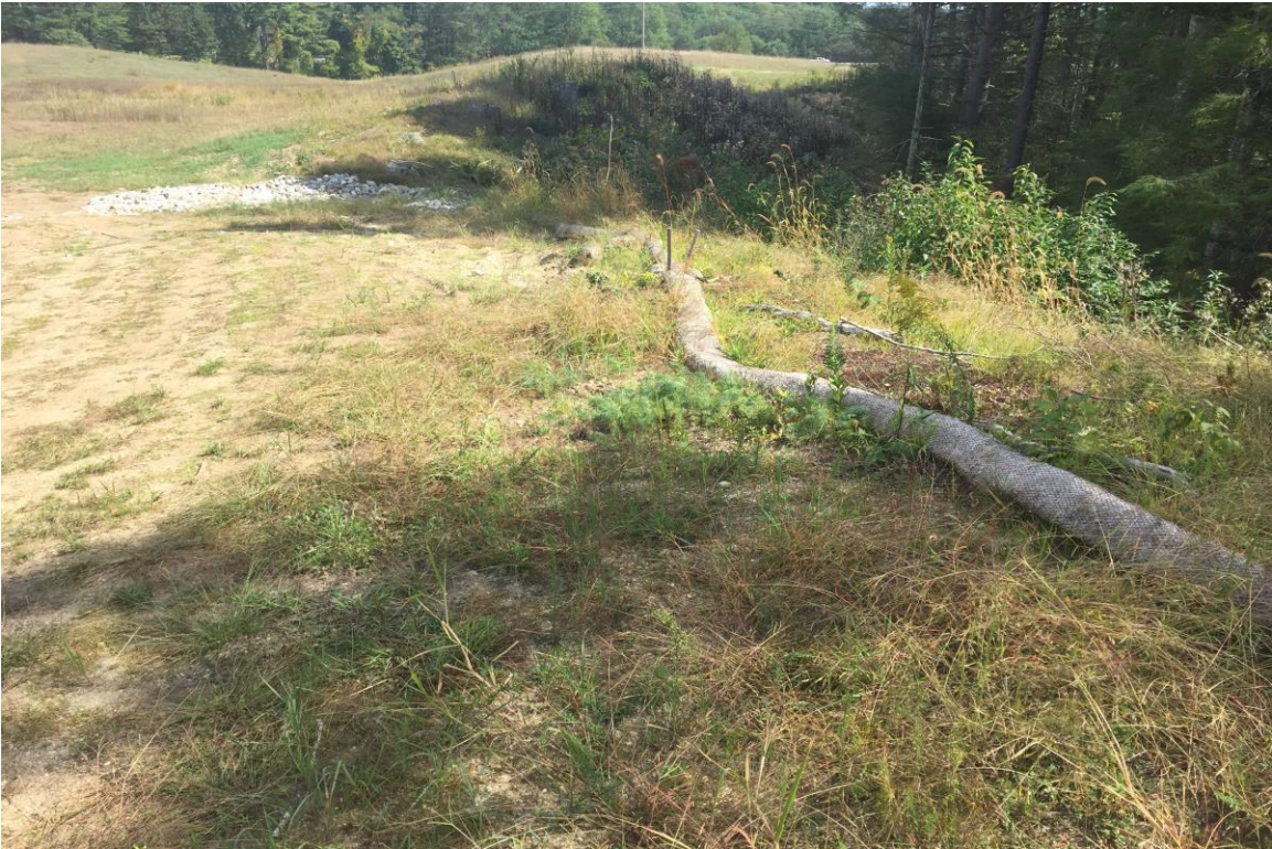
Photo 3: View of perimeter straw wattle controls looking east taken on 9/26/17.
