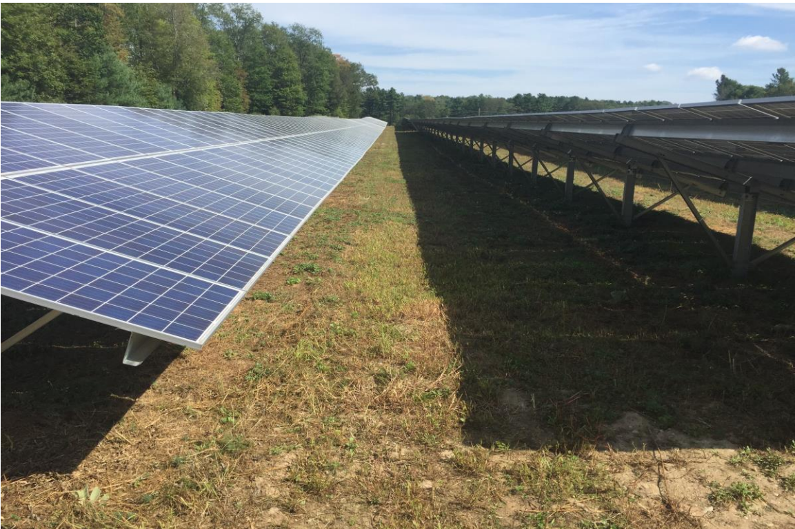
Photo 2: View of permanent vegetative stabilization in between solar arrays looking east taken on 9/26/17.
