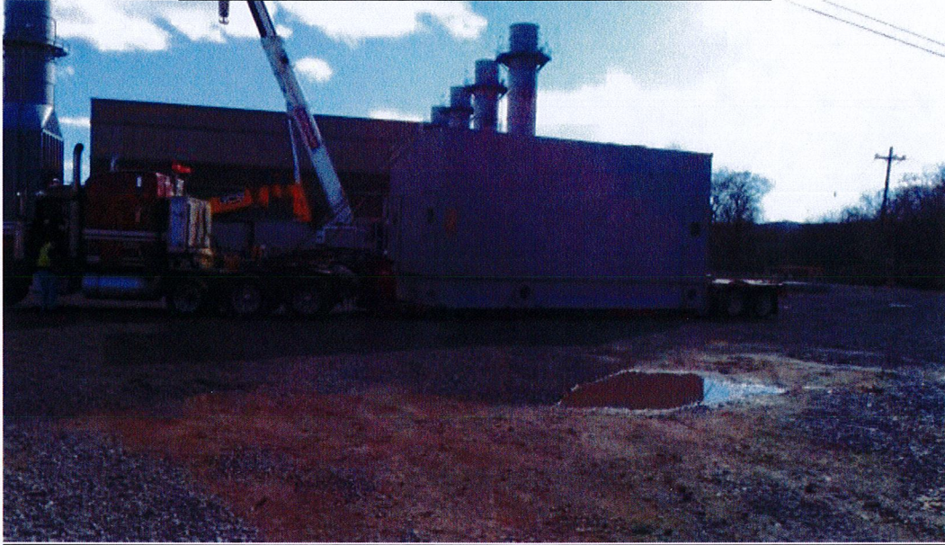
Inserting Trunnions in Generator Base for CTG # 6
