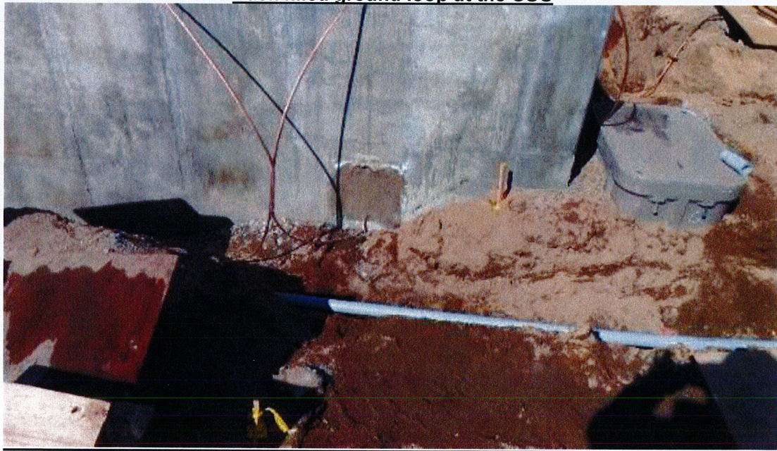
Back filled ground loop at the GSU
