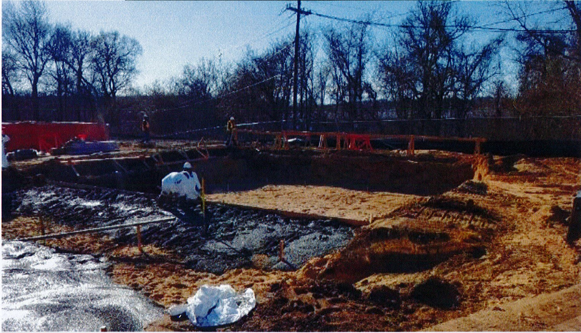
Poured flowable fill for Stack & SCR foundation # 7
