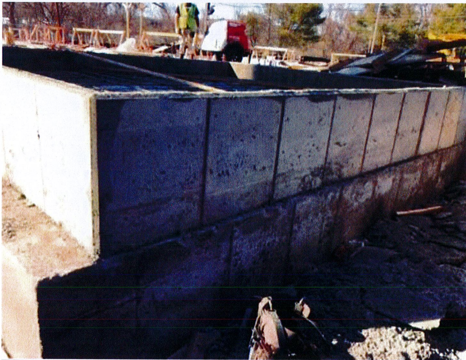
Stripped out form work for Auxiliary Skids CTG # 6
