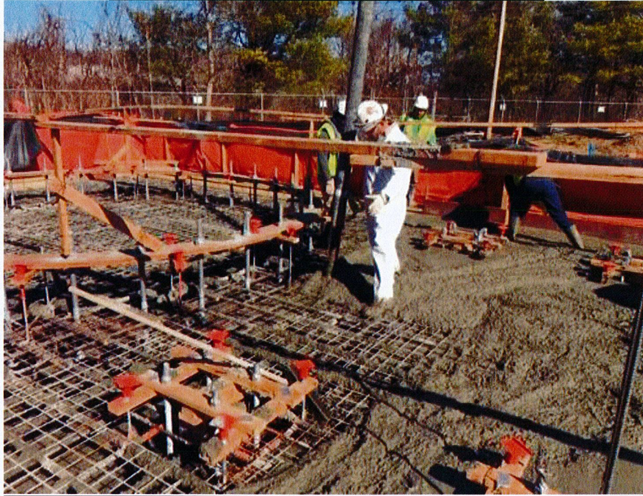
Poured concrete for Stack & SCR foundation # 7
