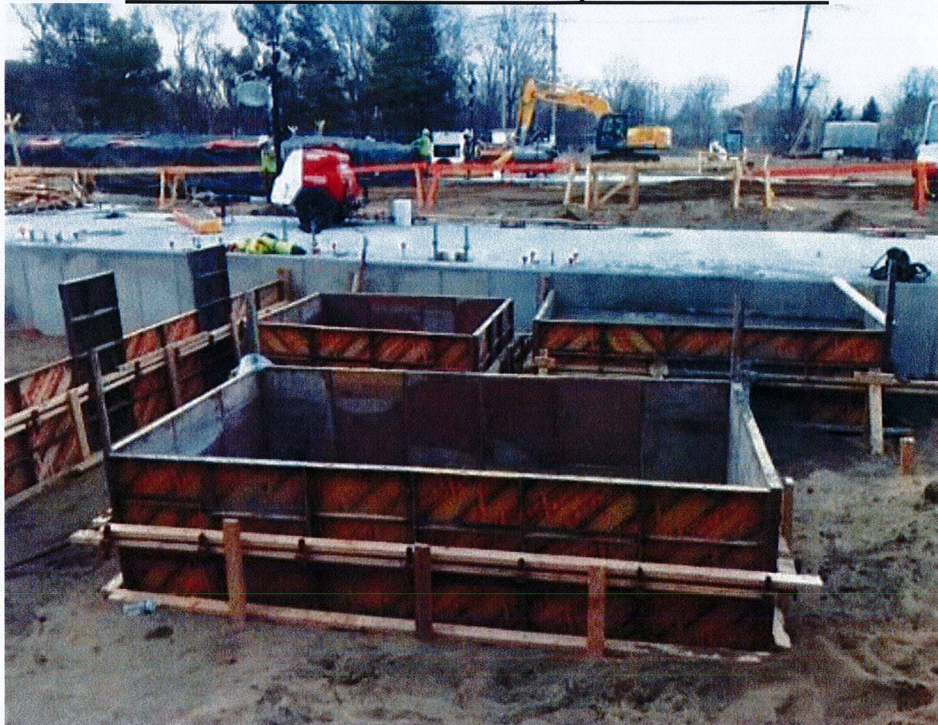
Excavated & set forms for Auxiliary Skids for CTG # 6
