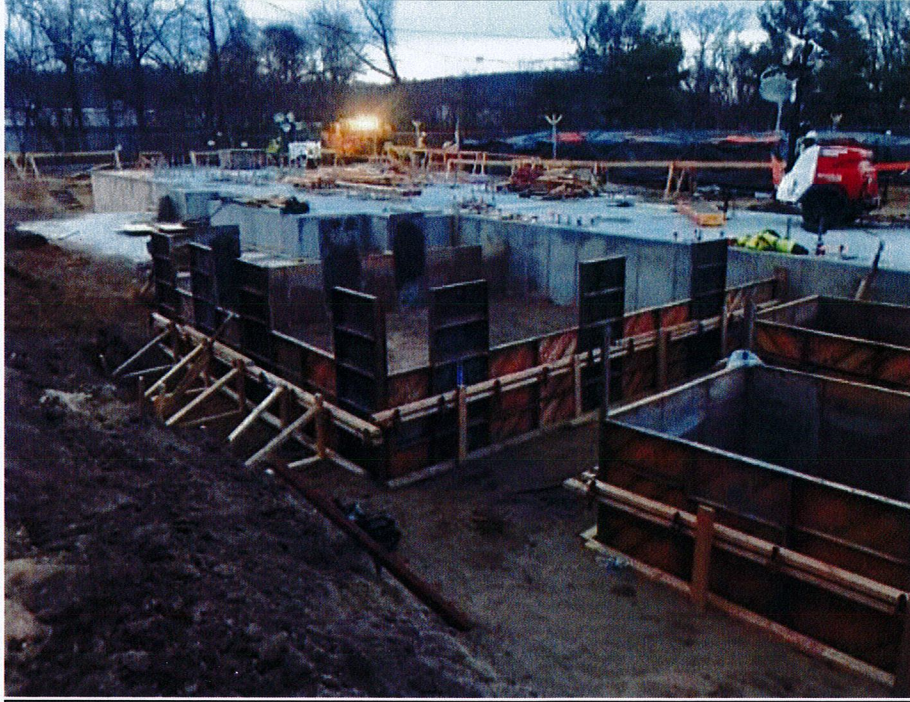
Excavated & set forms for Auxiliary Skids for CTG # 6
