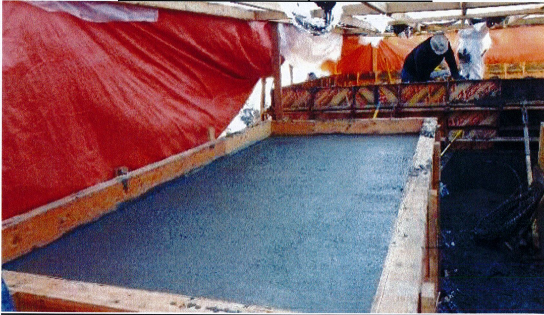
Poured concrete for Auxiliary skids for CTG # 6
