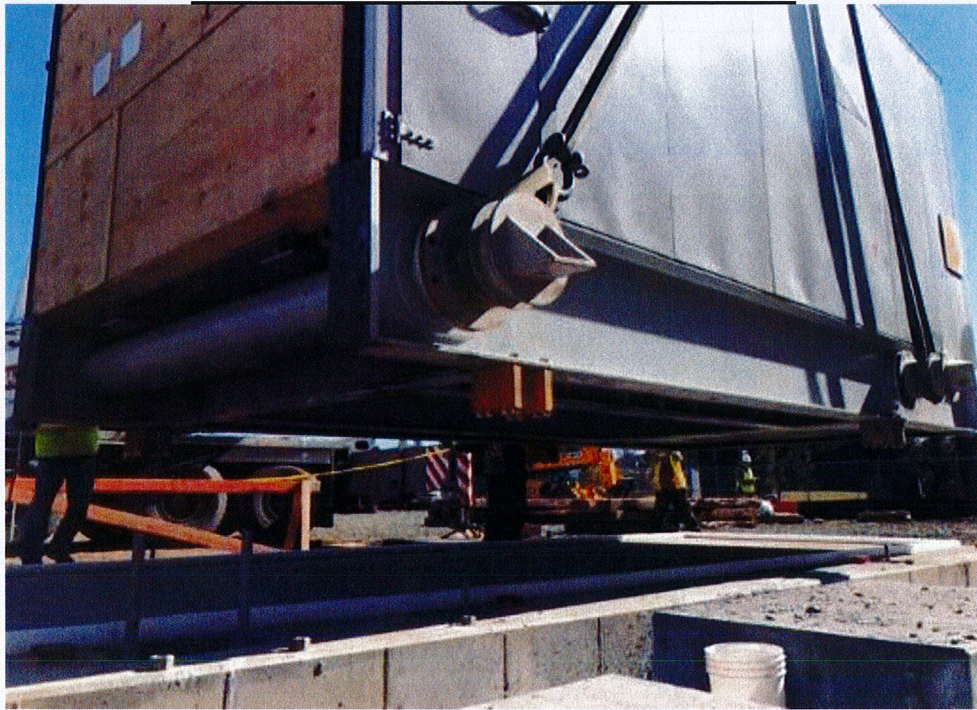
Set Generator Base on foundation for CTG # 6
