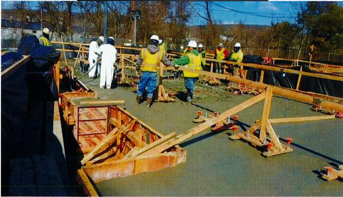
Poured concrete for Stack & SCR foundation # 6
