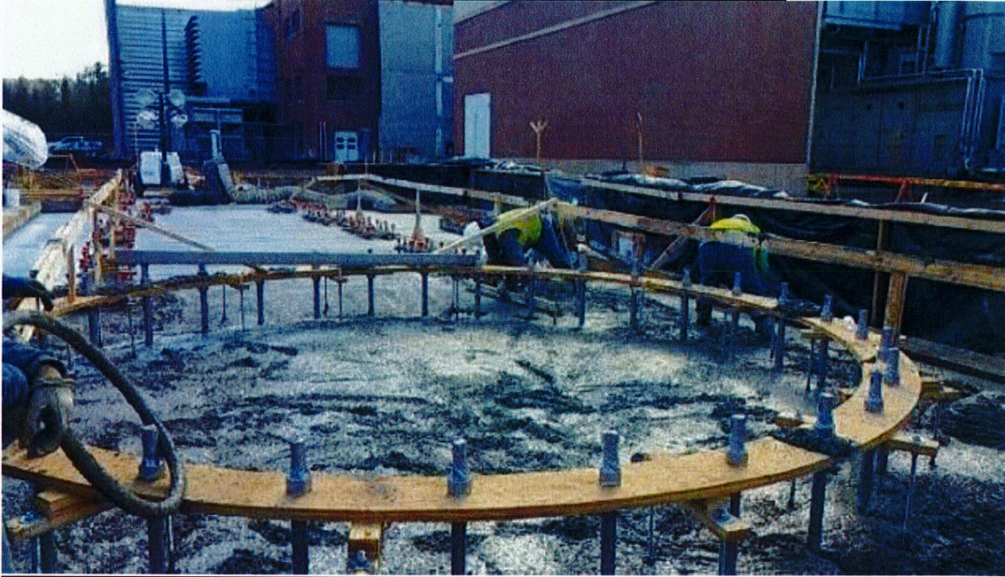
Poured concrete for Stack & SCR foundation # 6
