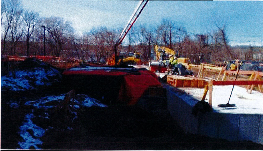
Poured flowable fill for Auxiliary skids for CTG # 6
