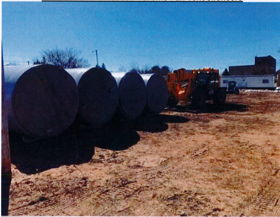
Received and unloaded Turbine Fan vent silencers
