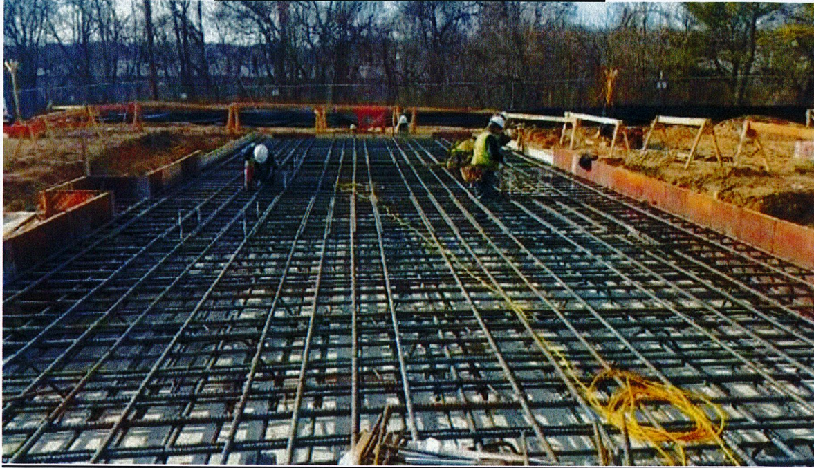
Setting anchor bolts for Stack & SCR foundation # 7
