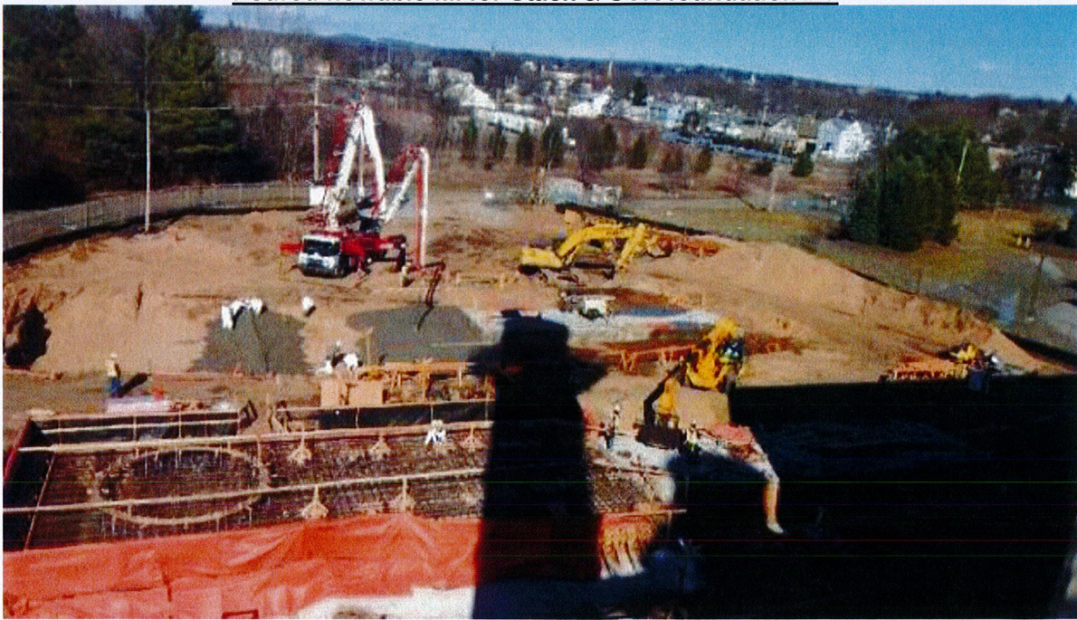
Poured flowable fill for Stack & SCR foundation # 7
