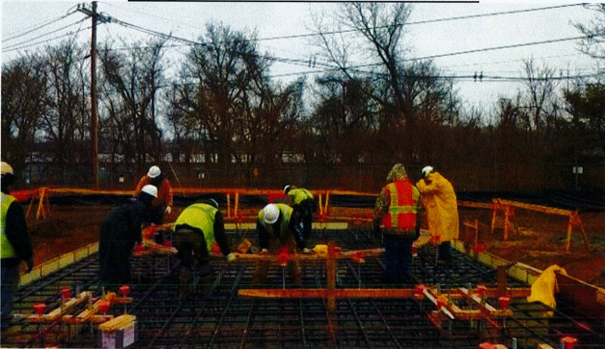
Setting anchor bolts for Stack & SCR foundation # 7
