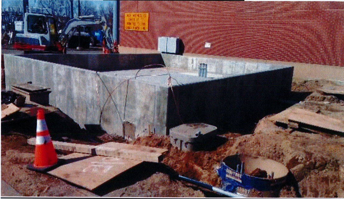
Back filled ground loop at the GSU
