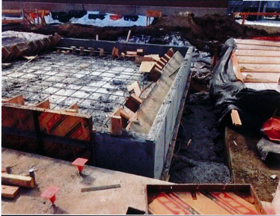
Stripped out form work for Auxiliary Skids CTG # 6
