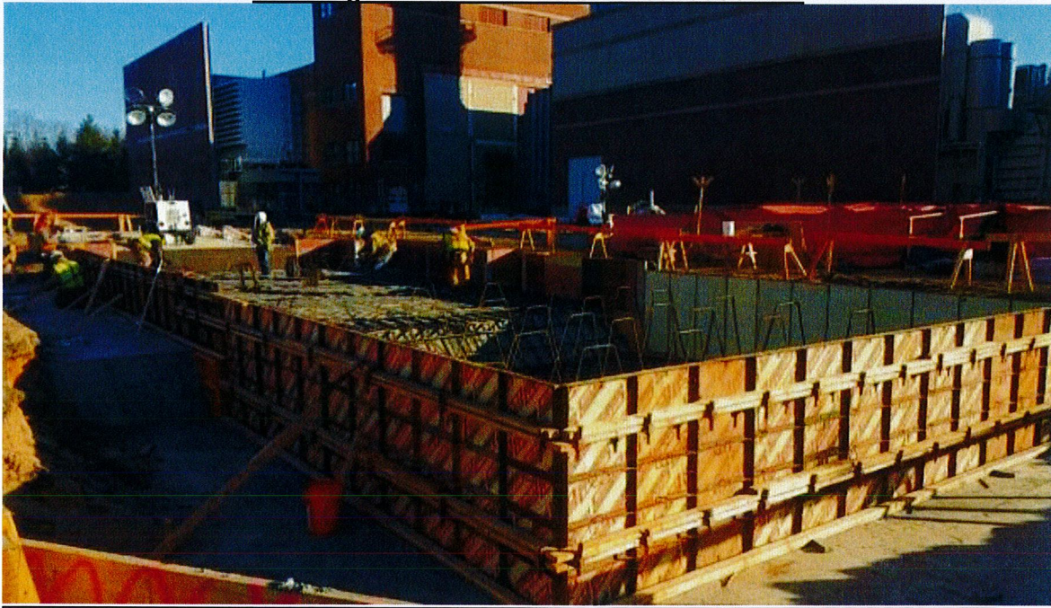
Installing rebar for Stack & SCR foundation # 7
