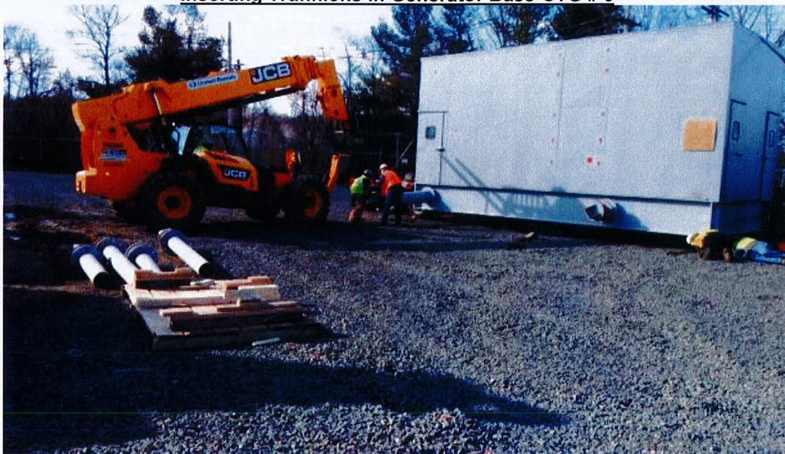
Inserting Trunnions in Generator Base CTG # 6
