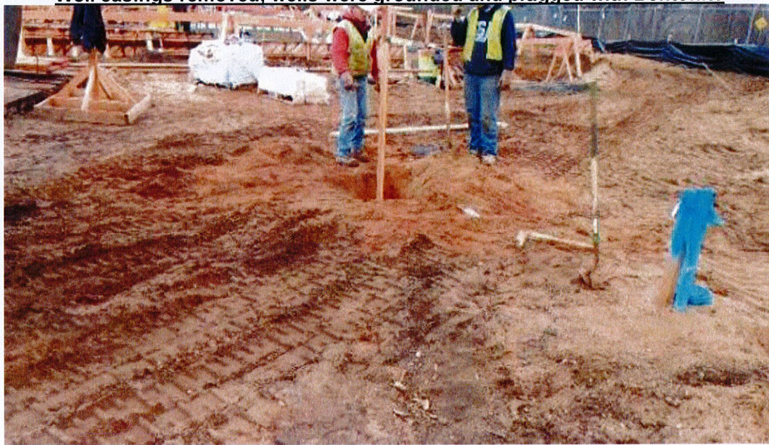
Well casings removed, wells were grouted and plugged with Bentonite
