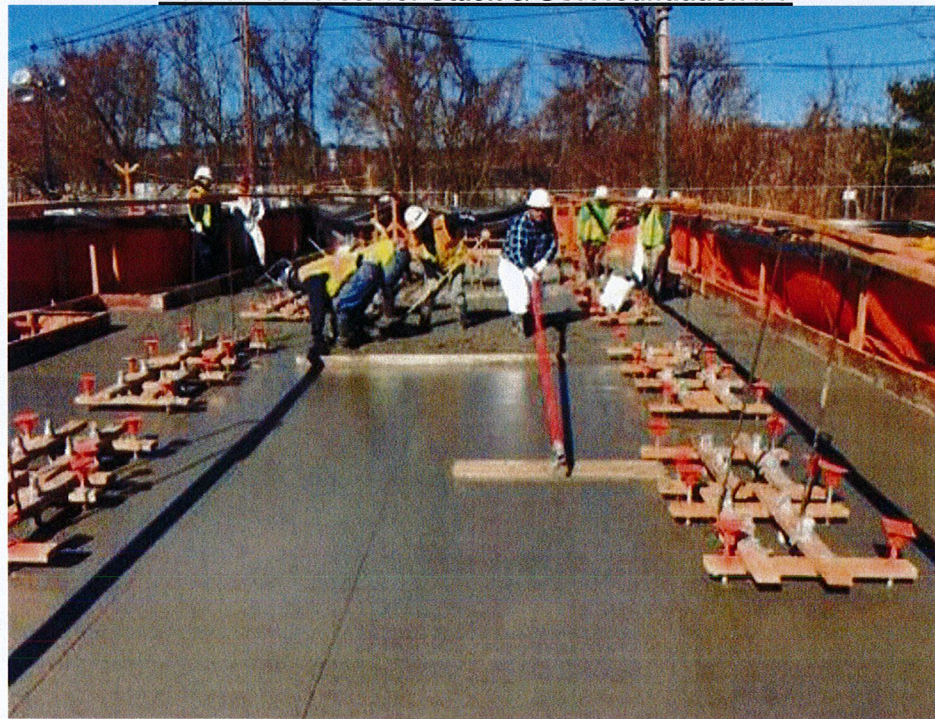
Poured concrete for Stack & SCR foundation # 7
