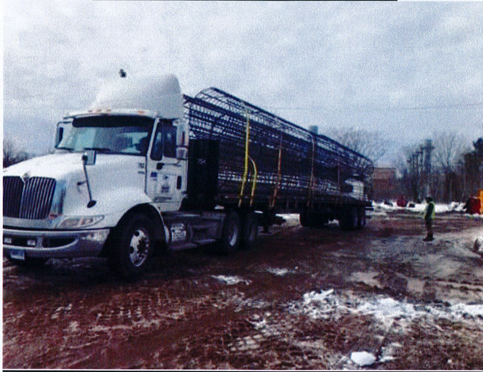
Received 18 rebar cages for Sound wall piers
