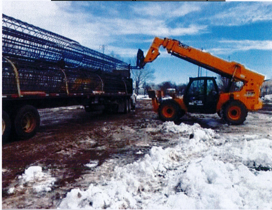
Received 18 rebar cages for Sound wall piers
