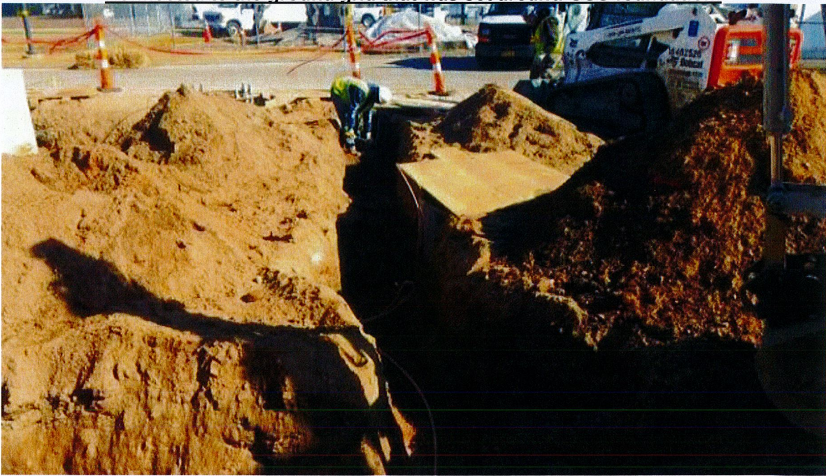
Connected to the ground grid that was set around GSU foundation.
