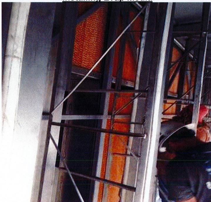
Installing Evap Media
