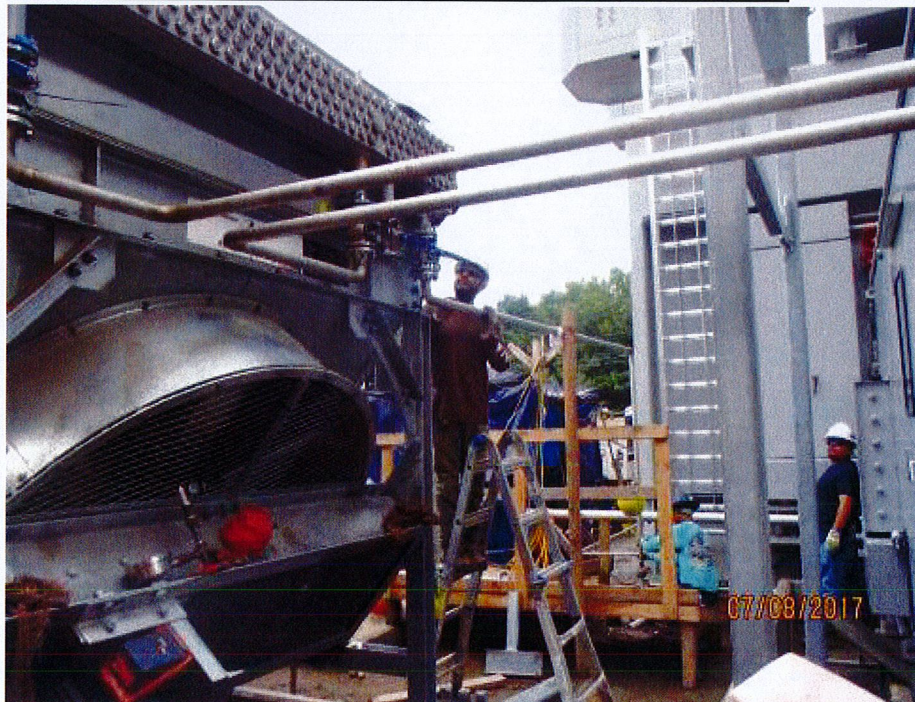
Continue working on LO cooling system piping.
