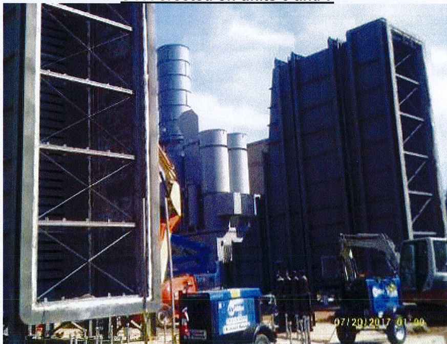
SCR erected on units 6 and 7
