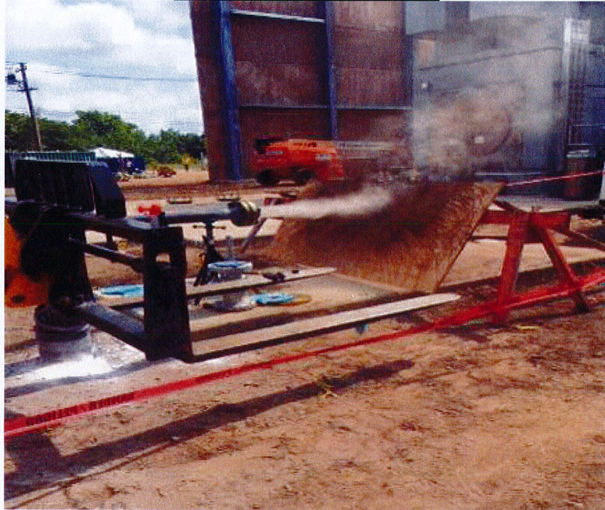
Gas Fuel Piping Air Blows
