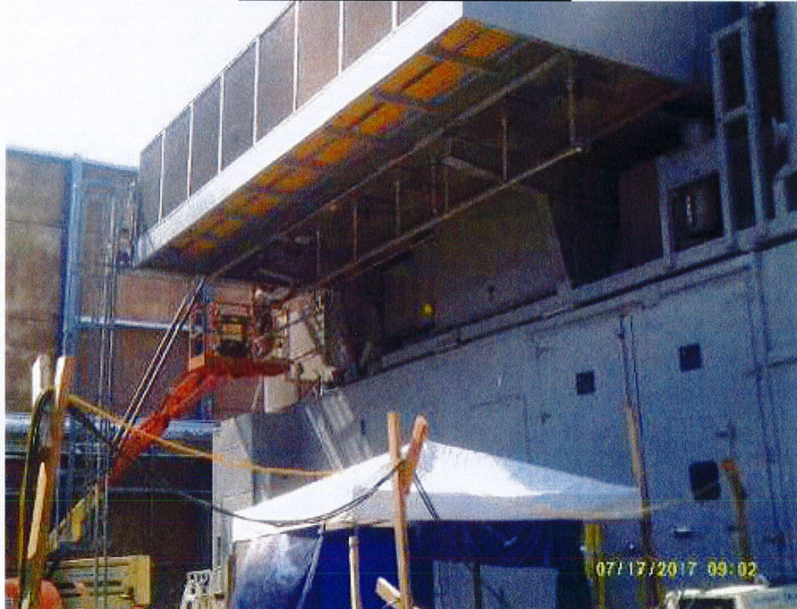
Installing header on unit 7
