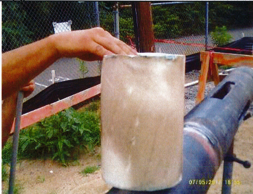
The last pig is clean from debris some soot from carbon smoke but clean
