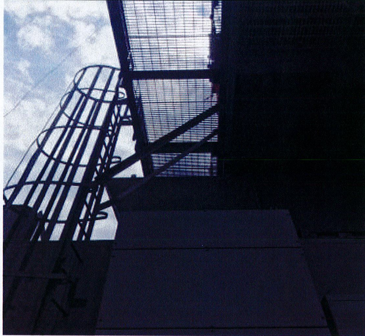
Filter house platform ladder mid supports unit # 7
