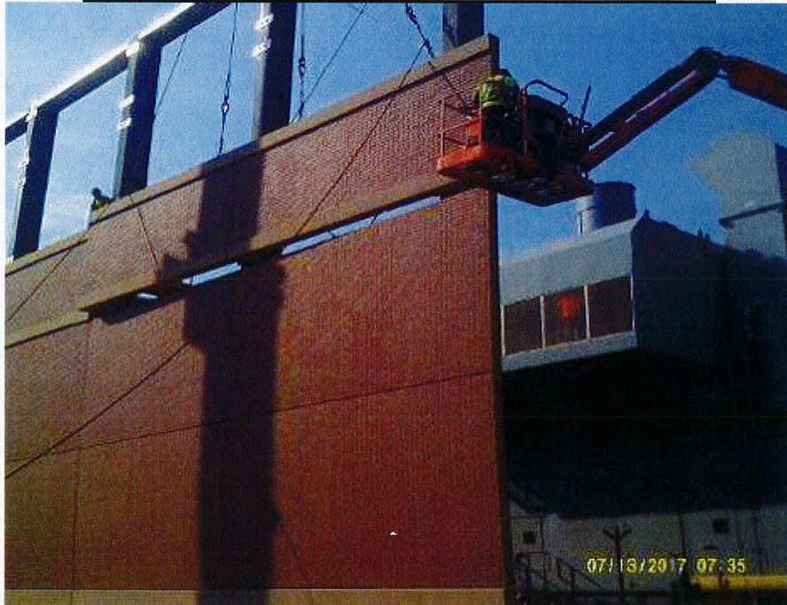
Sound wall south being erected on the South side
