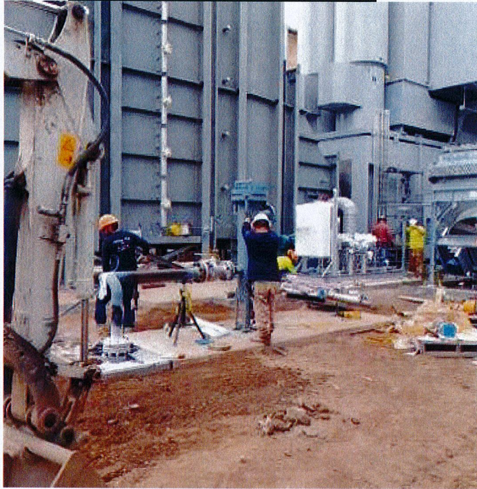
SCR view with Ammonia skid set in place.
