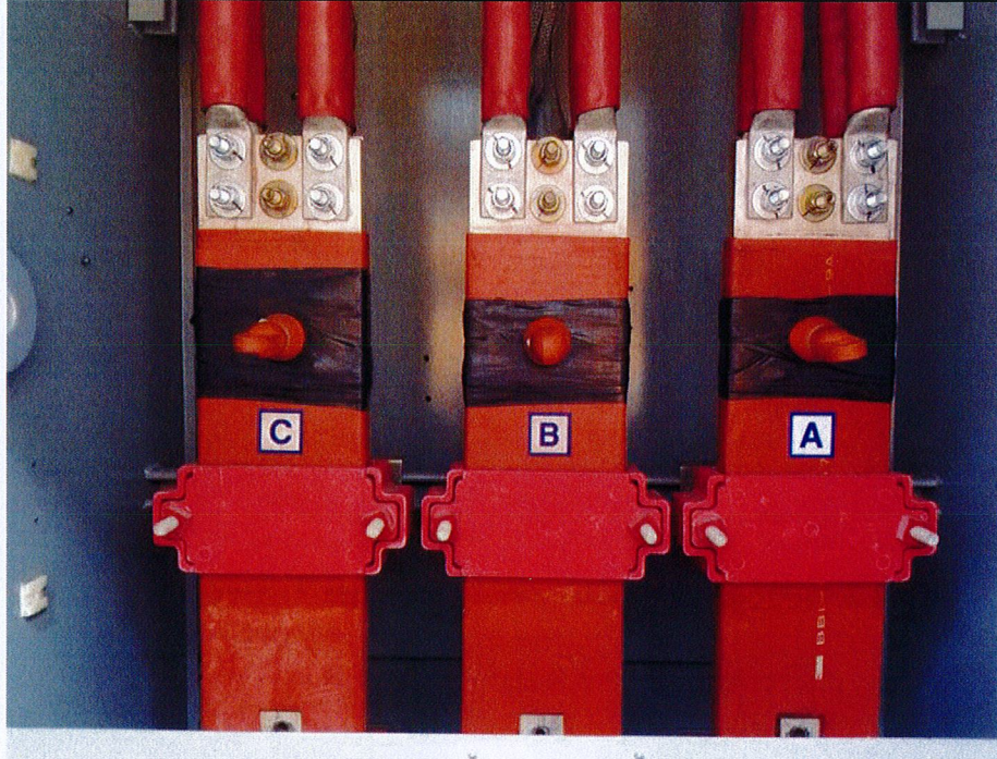
13.8 KV SWGR Top Section 3 from U-6 Generator Torqued 7/22/17 55 ft lbs
