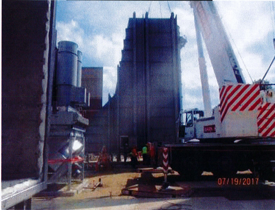
Set all 4 SCR modules on unit # 6
