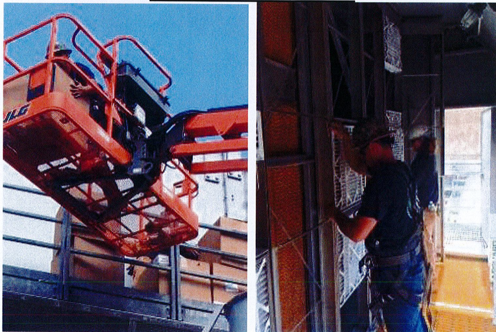
Installed Pre-filters Unit 6&7
