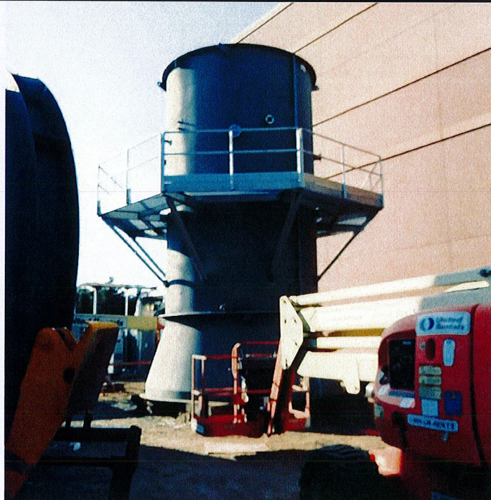
SCR installed platforms on the Transition unit on the stack
