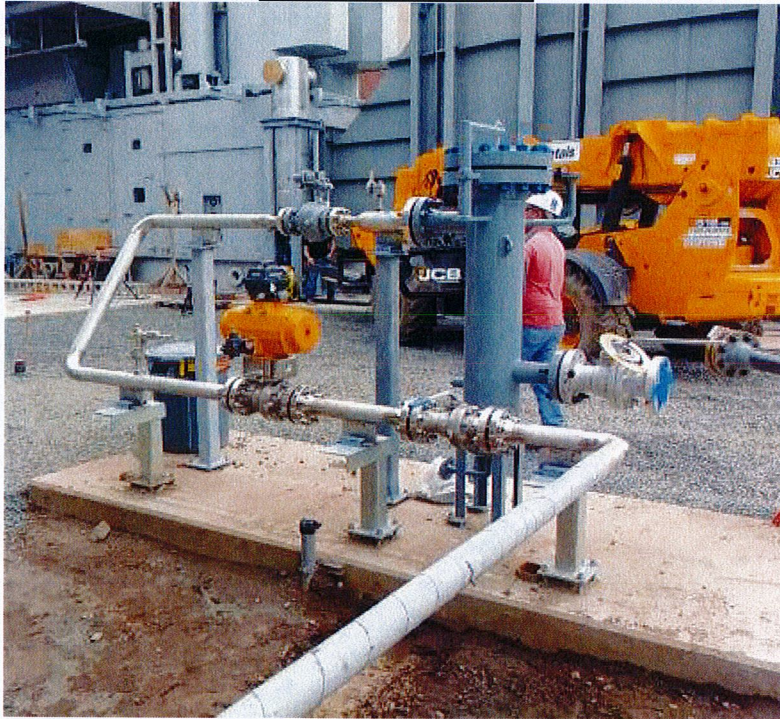
Tested lines 06FG-3-010-DC1-1 & 07FG-3-010-DC1-1 at 1200 PSI
