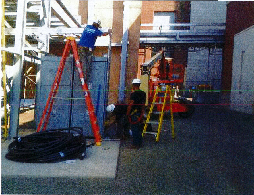
Electrical crew working on switchgear
