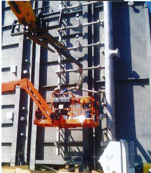
Installing lines on the SCR
