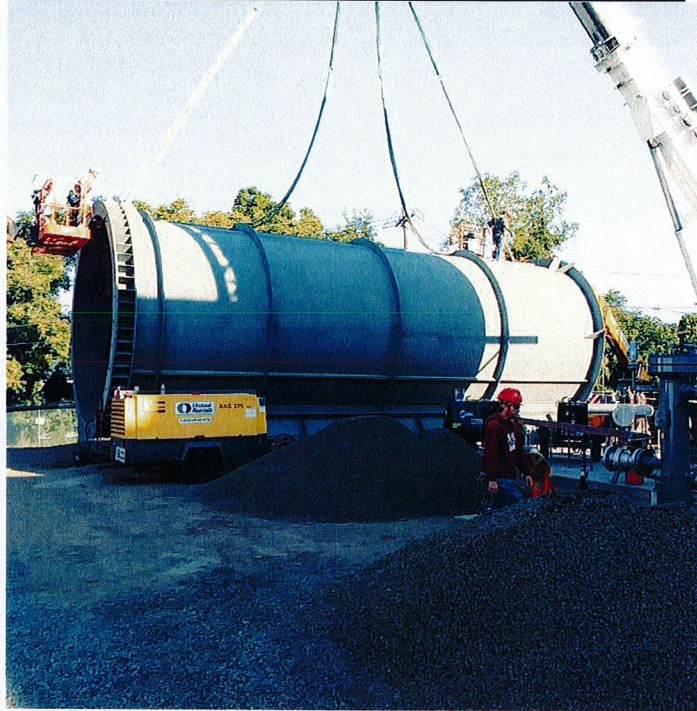
SCR installed platforms on the Transition unit on the stack
