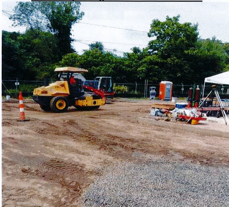
Civil compacting the North access road
