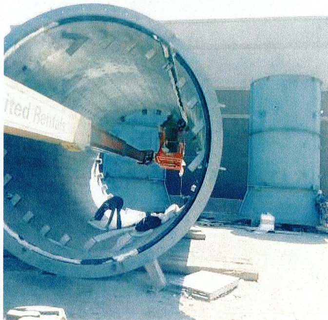
SCR welder working on Silencer
