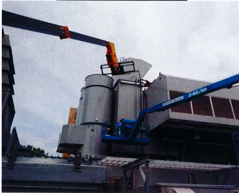
Working on fuel vent line on the side of unit #6
