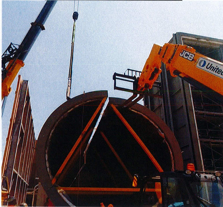
Assembled the breech for unit #2
