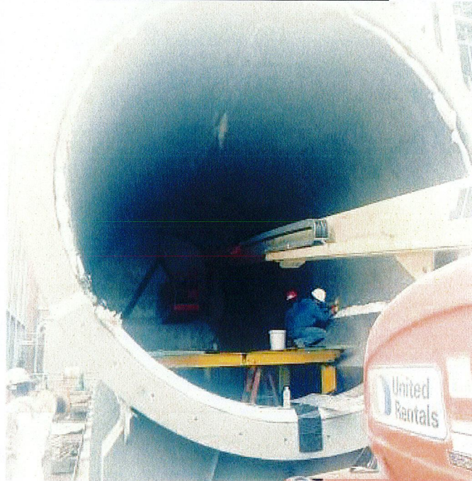
SCR welder working on Silencer
