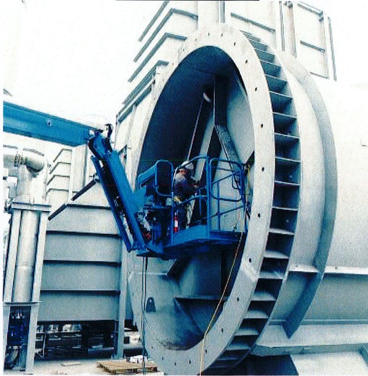
SCR crew member welding on the outside seam on silencers
