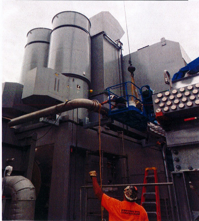
Installing inlet heating piping/duct unit 7
