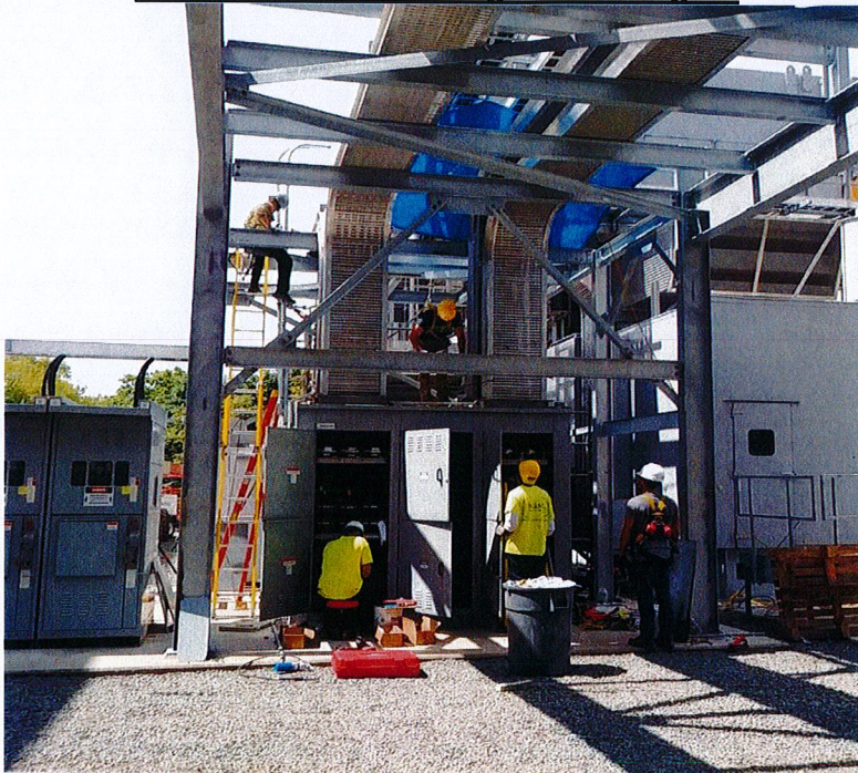
Electrical crew working on switchgear
