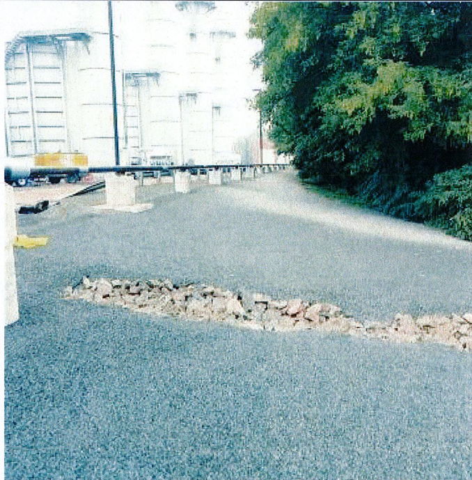
Grading and gravelling the North and South access roads
