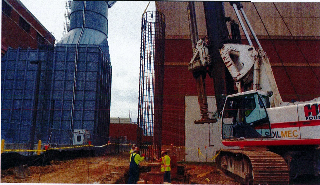
Set rebar cage on drill shaft for sound wall
