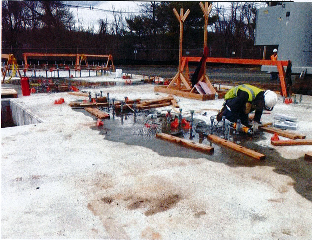
Remove all the templets and all tread from the SCR foundation # 7
