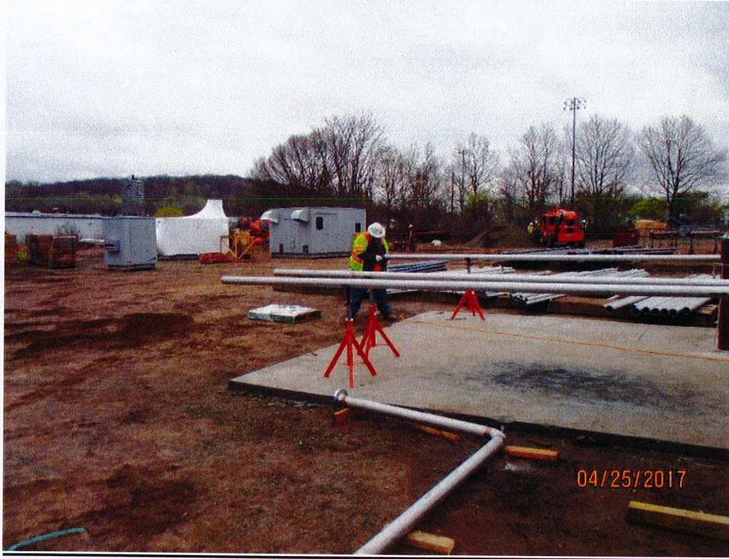
PVC fit and installed drain water
