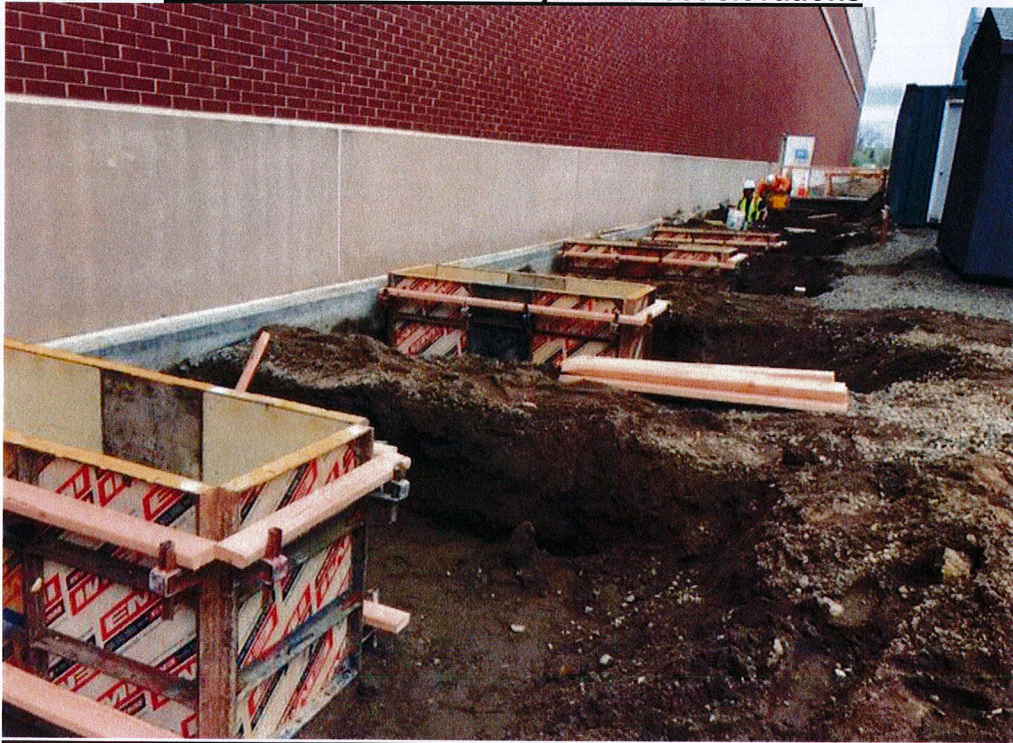
Set forms for the cable tray and shoot elevations
