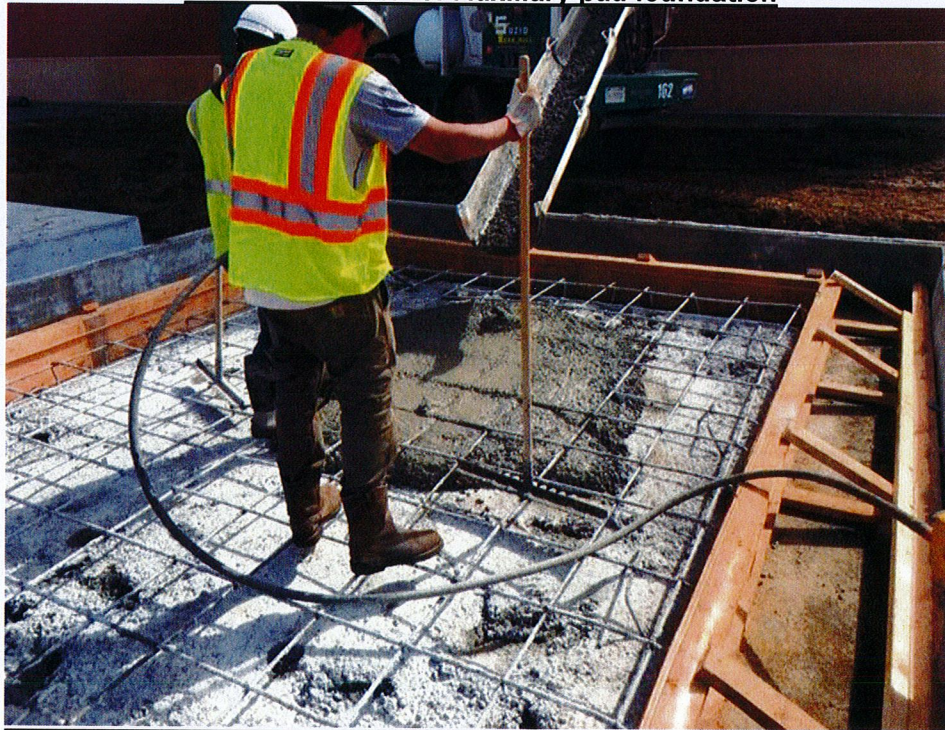
Poured concrete for Auxiliary pad foundation
