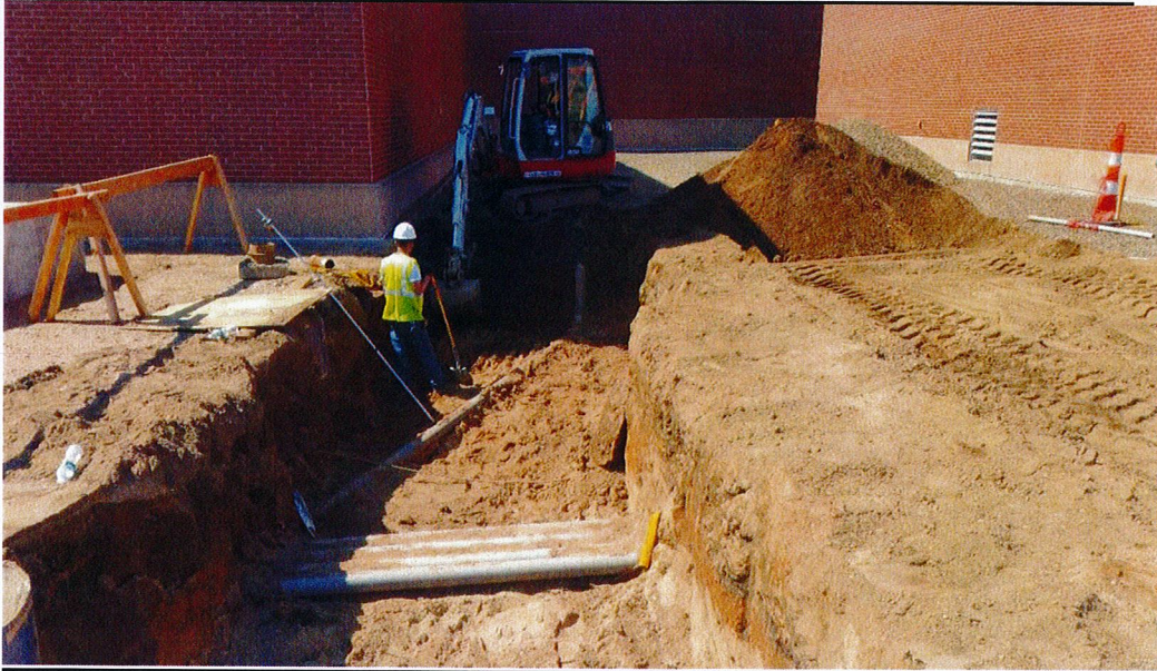
Excavated cable tray support from the GSU foundation to CTGs foundation
