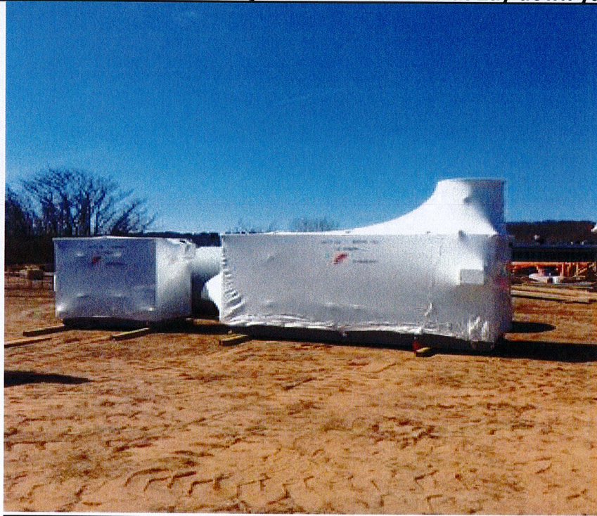
Unload Sprint, Lp water injection & Aux skids at Lay down yard
