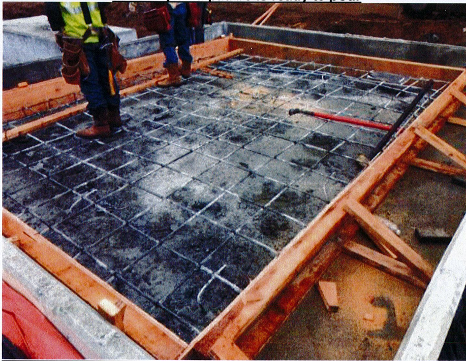
Auxiliary skid pad #6 is ready to pour
