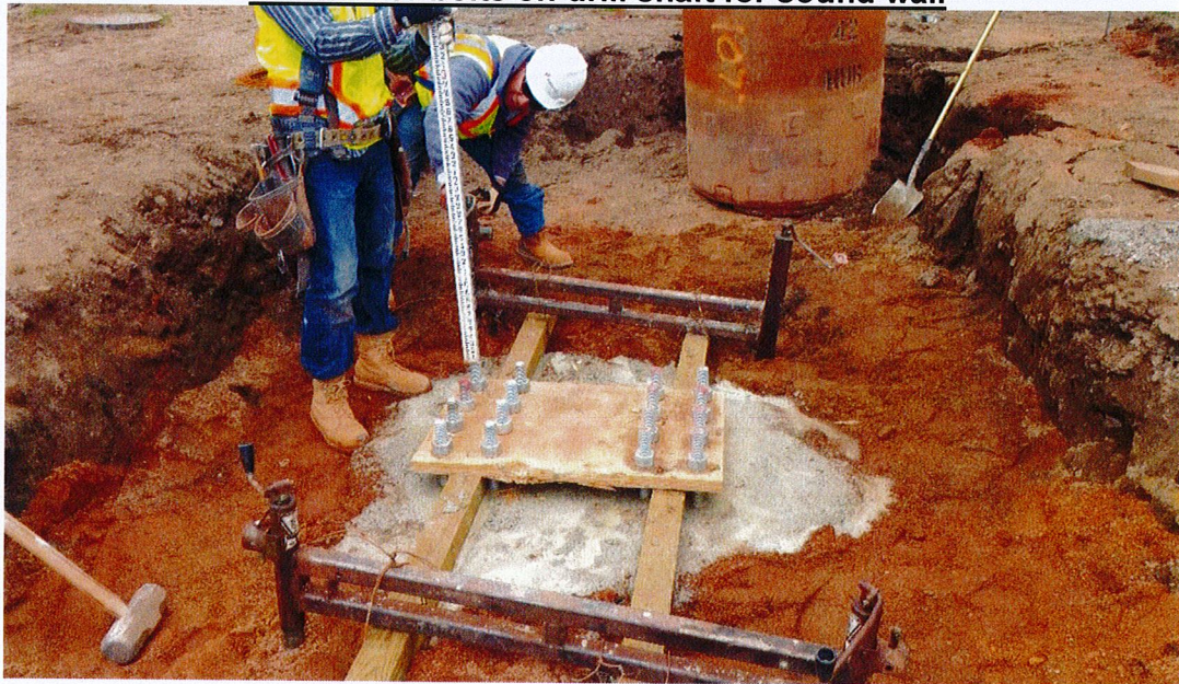
Set anchor bolts on drill shaft for sound wall
