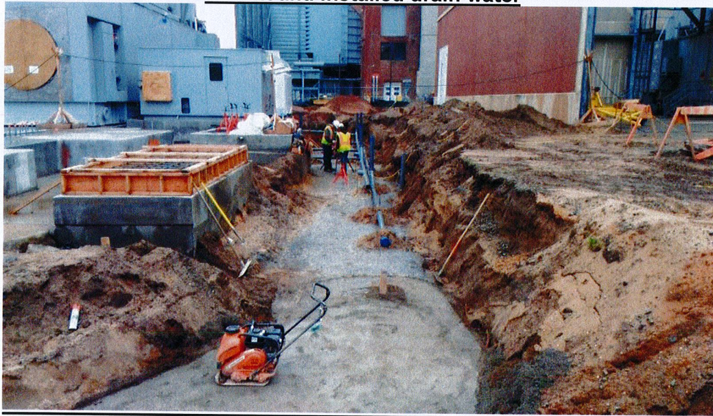
PVC fit and installed drain water
