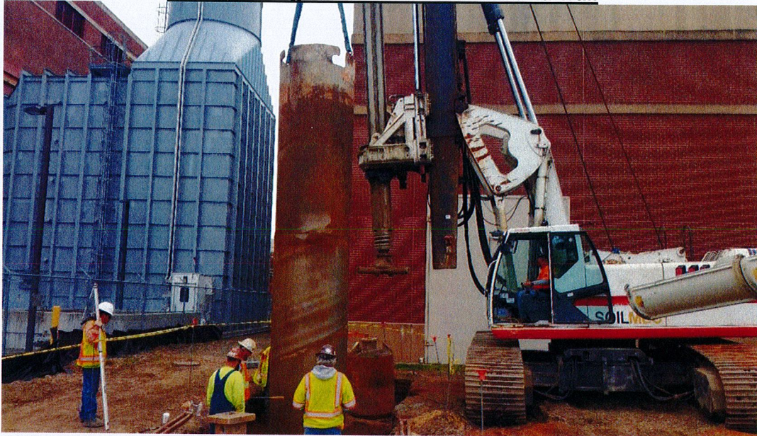
Set anchor bolts on drill shaft for sound wall
