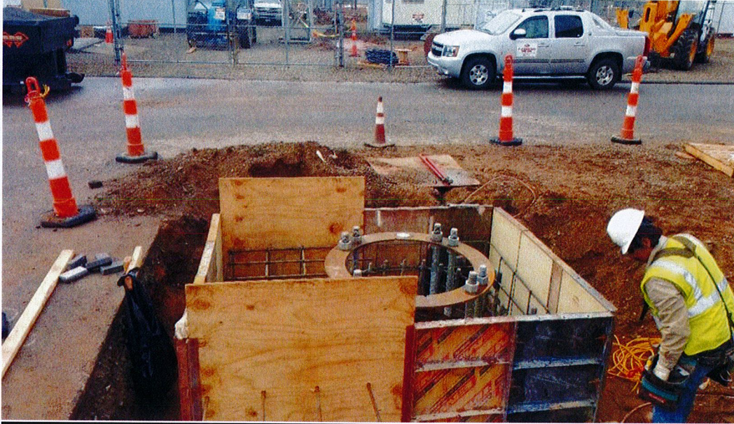
Finish setting forms on the block out for the H-frame
