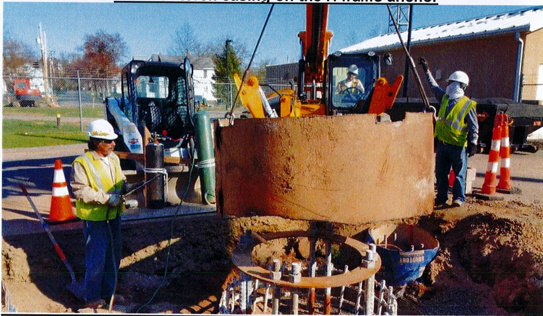
Cut with torch casing on the H frame anchor
