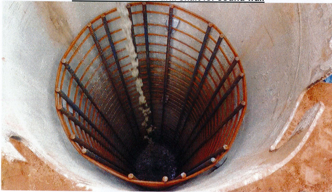
Poured concrete on drill shaft for sound wall
