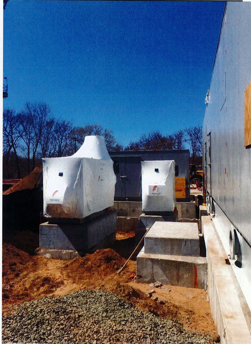
Set Sprint, Lp water injection & Aux skids for CTG # 6
