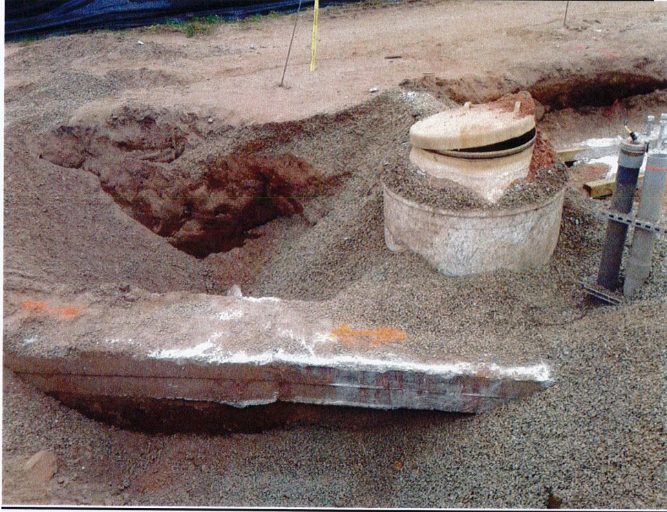
Unidentified Concrete cable vault in way of the CTG Sound Wall Piers
