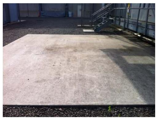
Photograph No. 12 View of change out concrete skid used when an engine or generator needs replacement.
