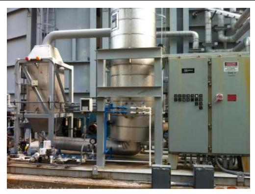
Photograph No. 17 View of ammonia vaporizer skid.
