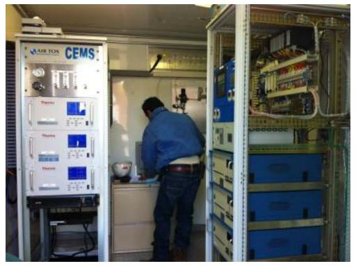
Photograph No. 20 View of air emissions monitoring equipment within the CEM enclosure.
