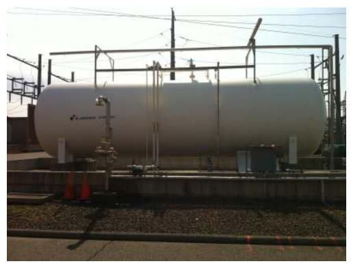
**Photograph No. 52**Northerly view of 20,000-gal 19% aqueous ammonia AST and containment area.
