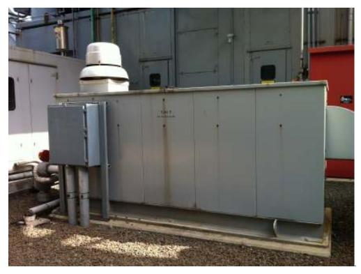
**Photograph No. 6**NOx water injection skid.
