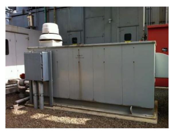
Photograph 5: NOx water injection skid
