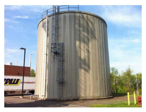
Photograph 7: 250,000 gallon demineralized water AST
