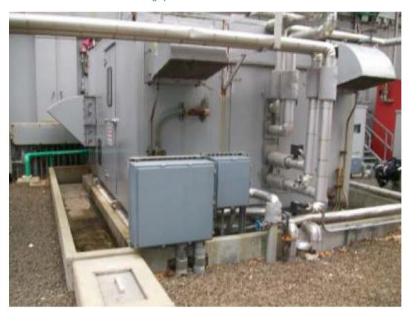
Photograph 10: Enclosure near gas combustion turbines mounted within a secondary containment structure
