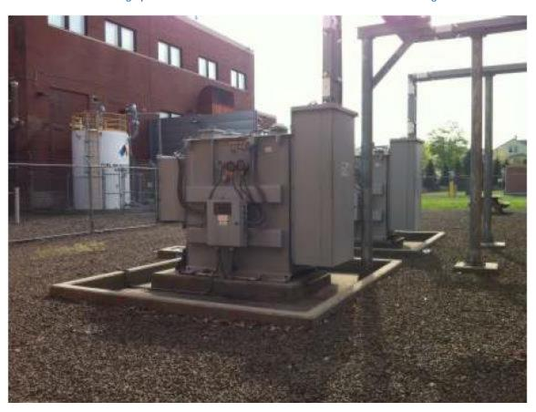
Photograph 4: View of transformers and associated secondary containment
