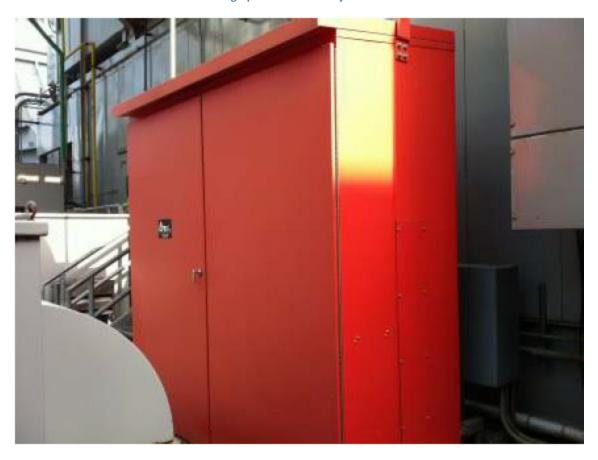
Photograph 6: Fixed CO<sub>2</sub> fire protection
