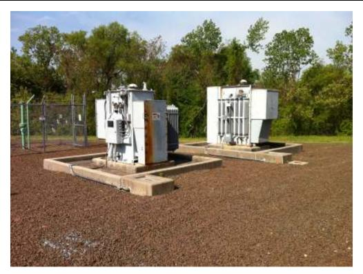
Photograph No. 39 Plant auxiliary transformers.
