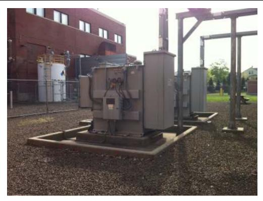
Photograph No. 5 View of transformers and associated secondary containment.
