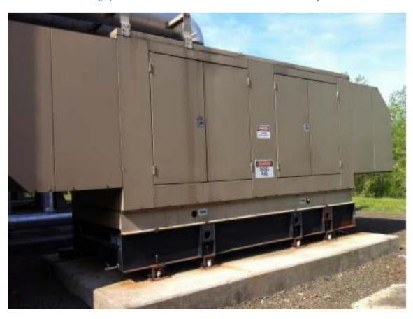
Photograph 16: Black start generator located behind the compressor building. A 500gallon diesel tank is located within the generator compartment
