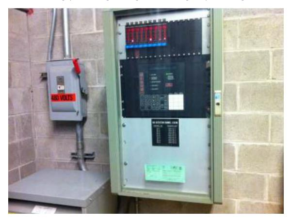
Photograph 20: Natural gas detection system located inside anti-icing boiler room
