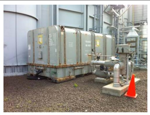
Photograph No. 21 Spare engine located on site within secondary containment.
