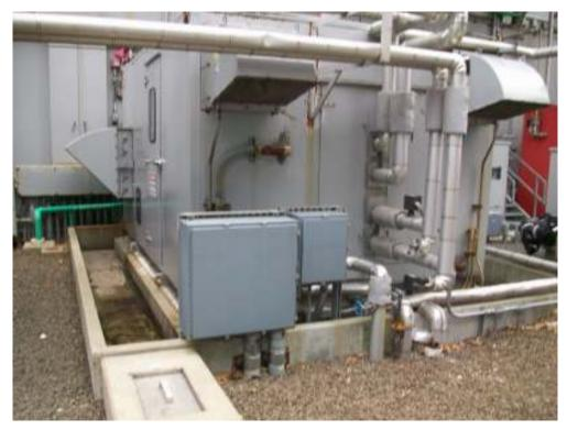
Photograph No. 11 Enclosure near gas combustion turbines mounted within a secondary containment structure.
