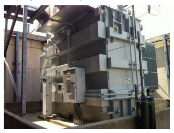
Photograph 26: One of three step-up transformers
