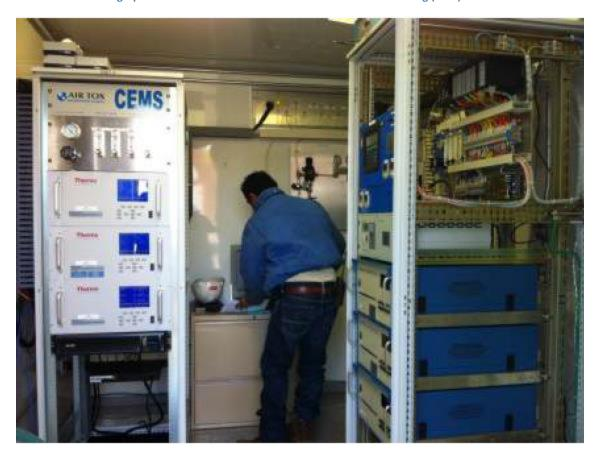
Photograph 12: View of air emissions monitoring equipment within the CEM enclosure
