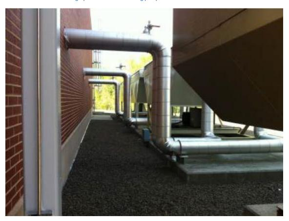
Photograph 18: Coolers located on the exterior of the natural gas compressors building
