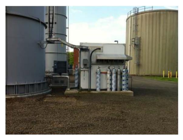
Photograph 11: View of exterior of continuous emissions monitoring (CEM) enclosure
