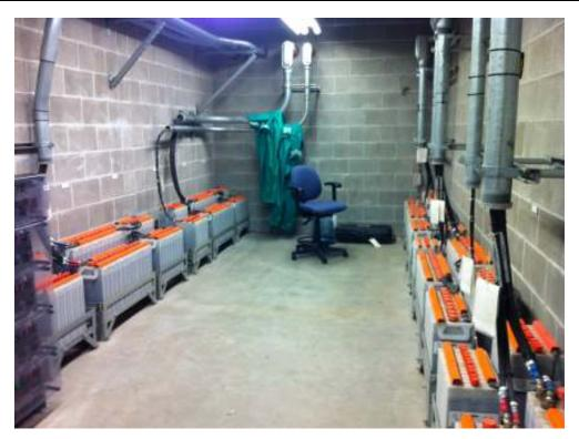
Photograph No. 51 View of battery cell blocks inside the battery room.
