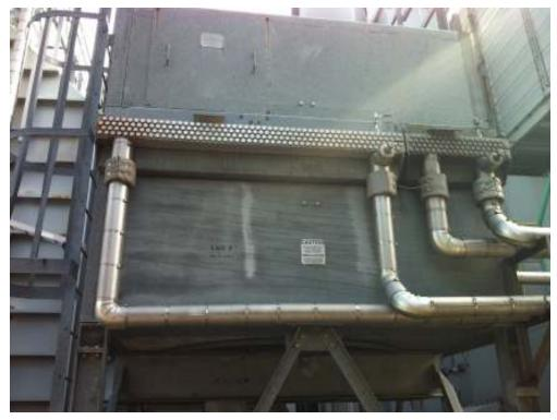
Photograph No. 16 View of lube oil cooler.
