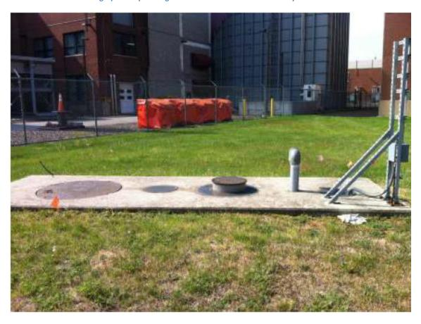
Photograph 14: View of the 4,000-gal process wastewater UST
