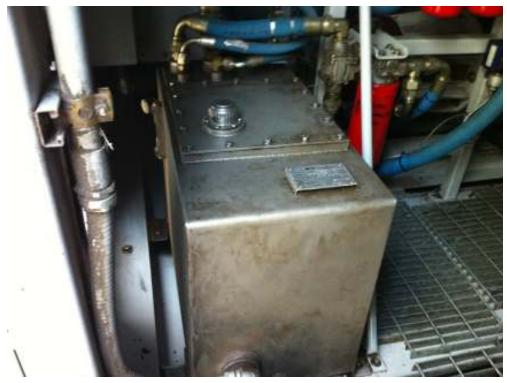
Photograph No. 14 Hydraulic starter tank which contains hydro oil.
