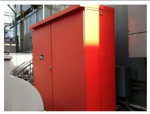
**Photograph No. 7** Fixed CO<sub>2</sub> fire protection.
