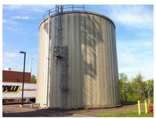
**Photograph No. 24** 250,000 gallon demineralized water AST.
