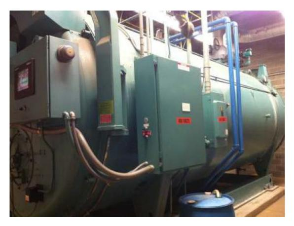
Photograph 19: Anti-icing hot water generator inside the gas compressor building
