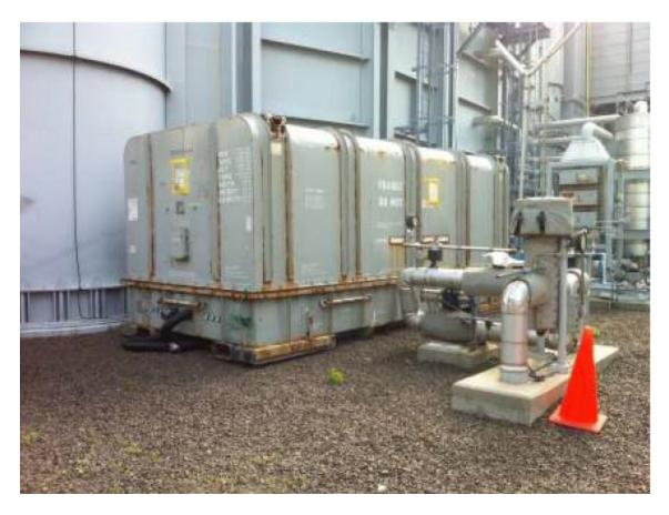
Photograph 13: Spare engine located on site within secondary containment
