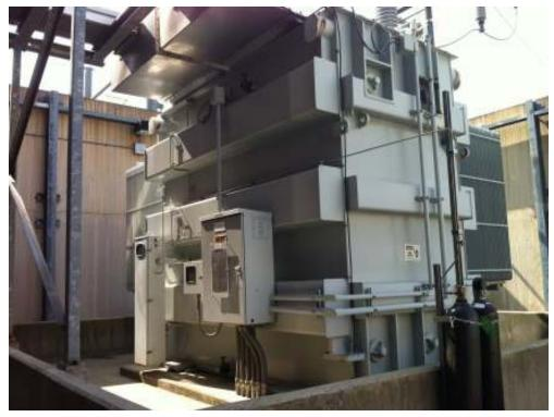
**Photograph No. 44** One of three step-up transformers.
