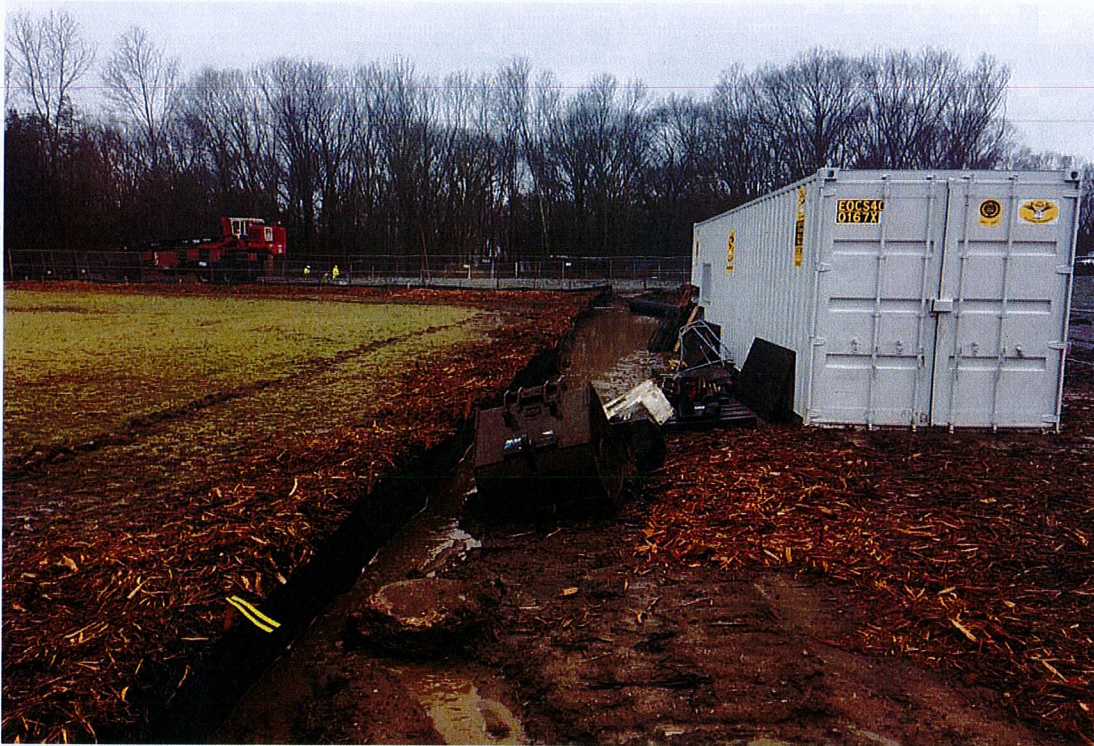
Photo 1: View of perimeter controls south of laydown yard looking west.
