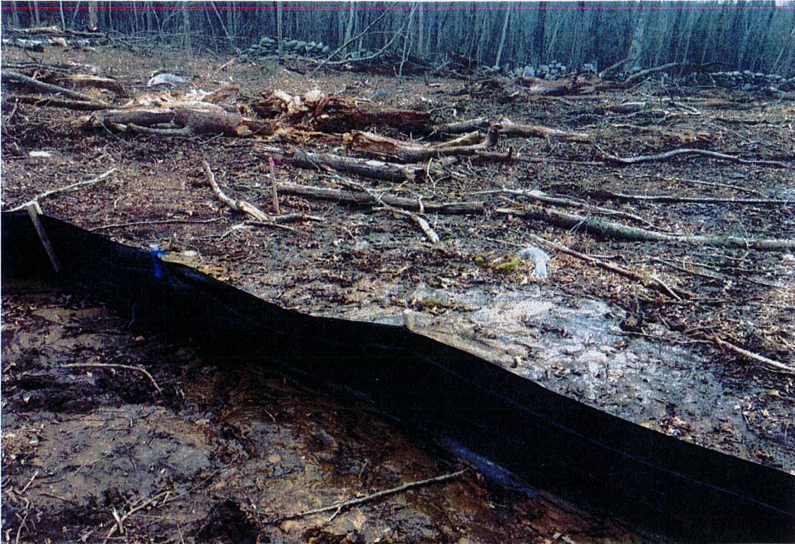
Photo 5: View of CA #8 sediment release within uplands on site.
