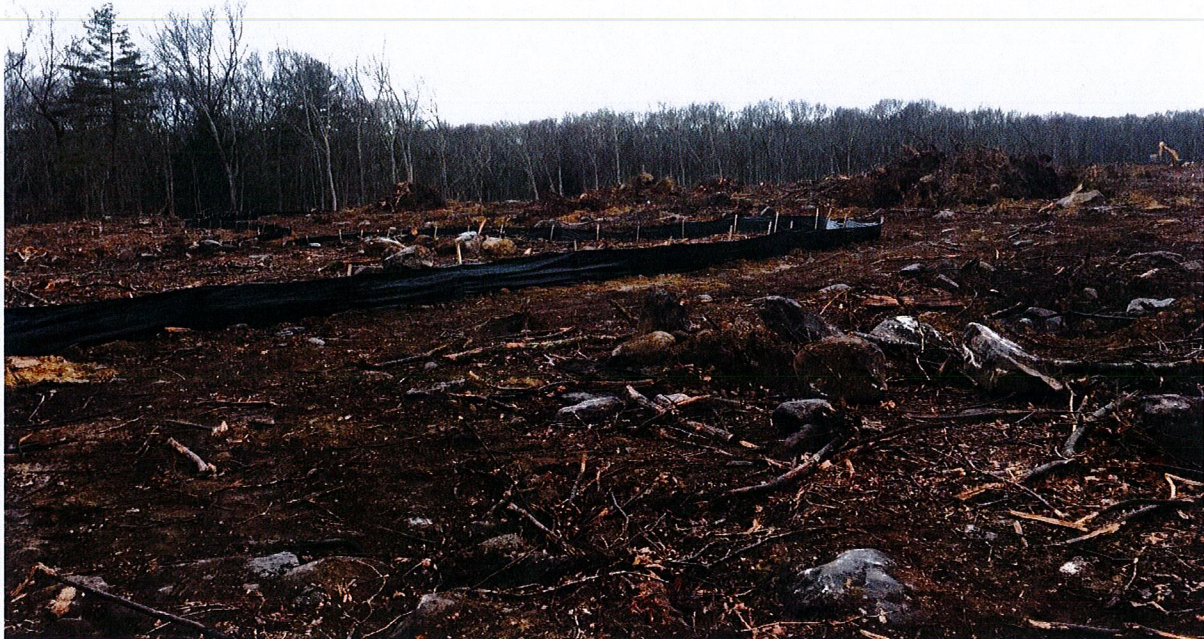
Photo 3: View of western silt fence line looking north.
