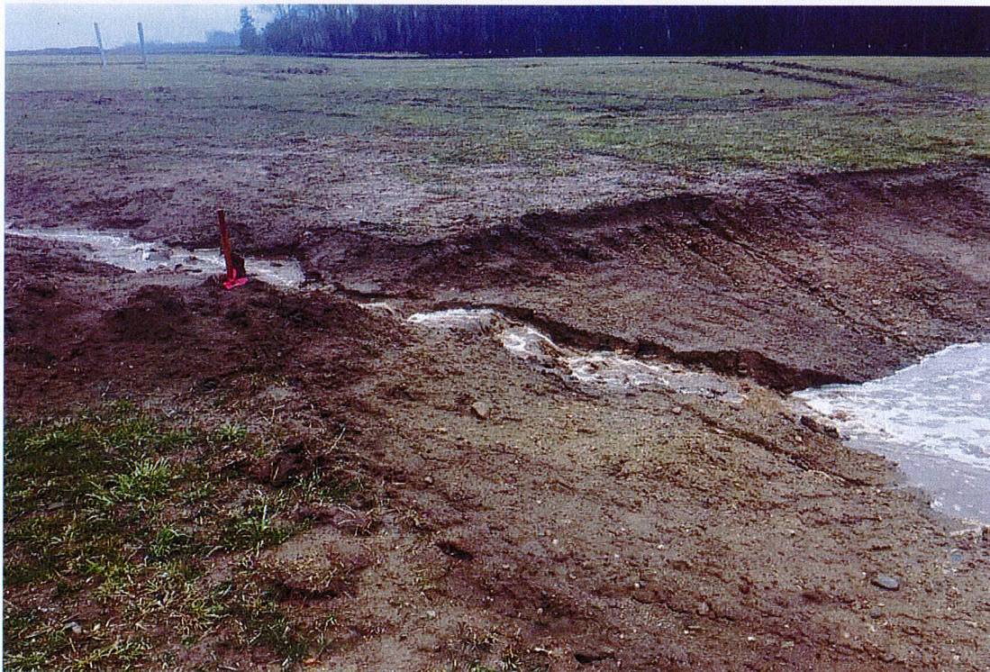
Photo 2: View of inlet to sediment trap ST-12 looking east.
