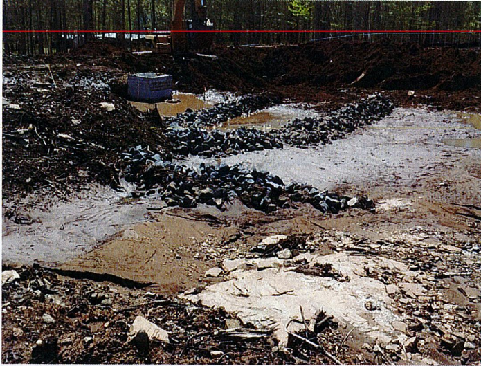
Re-work to SB-3 to double its current capacity.
