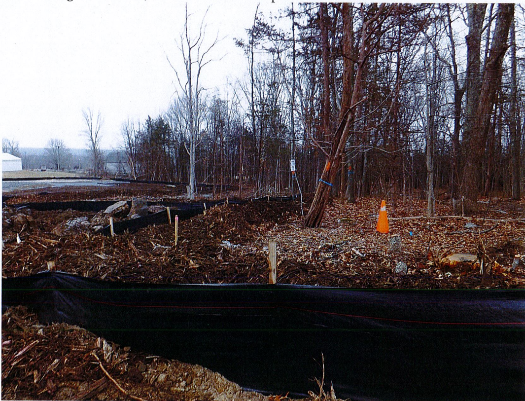
View of Silt Fence (on subject property) and Cone Depicting Mr. Bates' Property – View facing south
