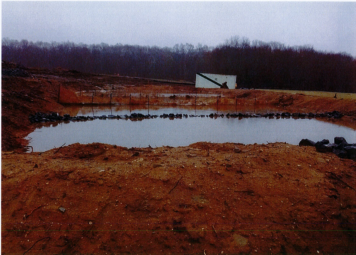
Sediment Basin SB-3
