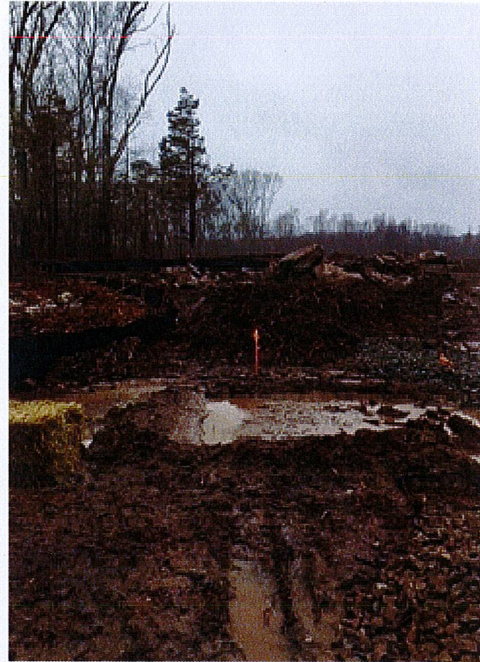
Excavated water detention "pit" below check dam
