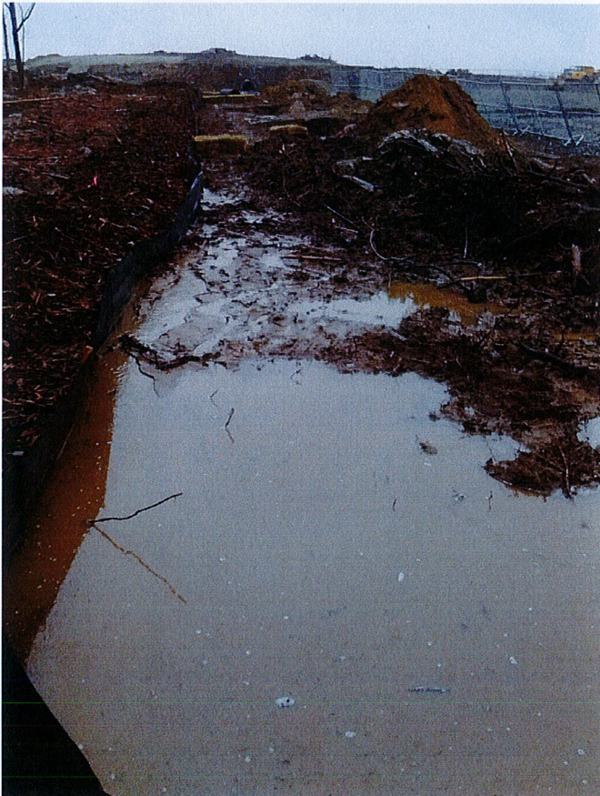
Ponded water, southwest corner, below SB-3
