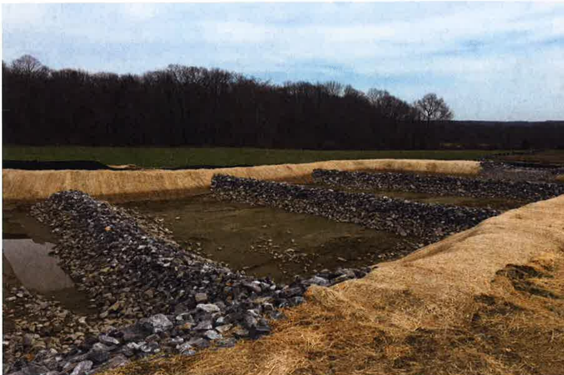
Photo 2: View of a typical sediment basin.
