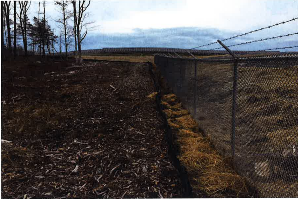
Photo 7: View of typical silt fence perimeter.
