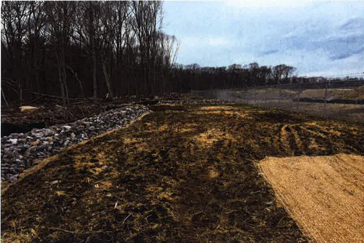
Photo 5: View of northwest project corner.
