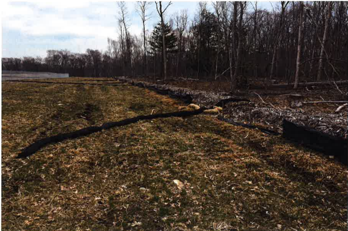
Photo 6: View of typical silt fence opening.
