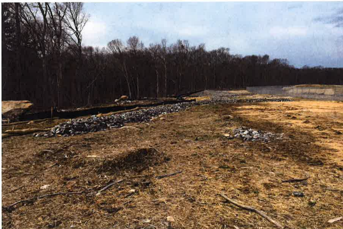
Photo 4: View of northwest project corner.
