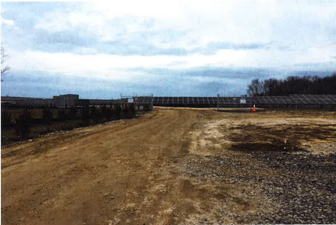
Photo 1: View of access road entrance looking north.
