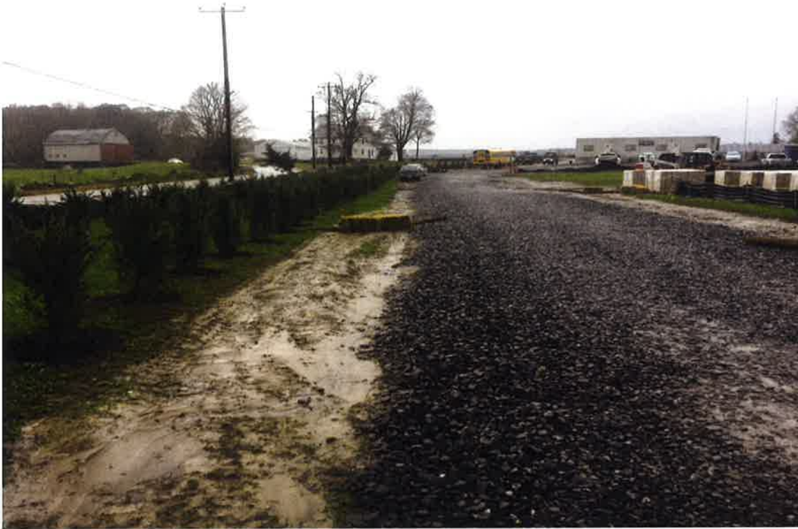
Photo 1: View of access road looking north.
