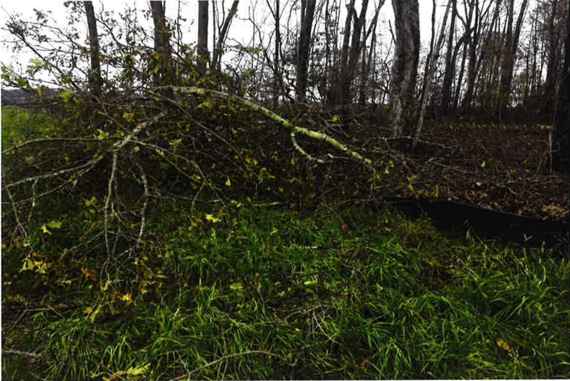
Photo 5: View of silt fence break needing repair.
