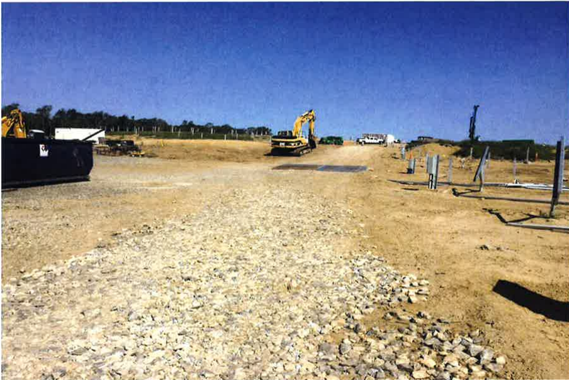
Photo 1: View of access road looking north.
