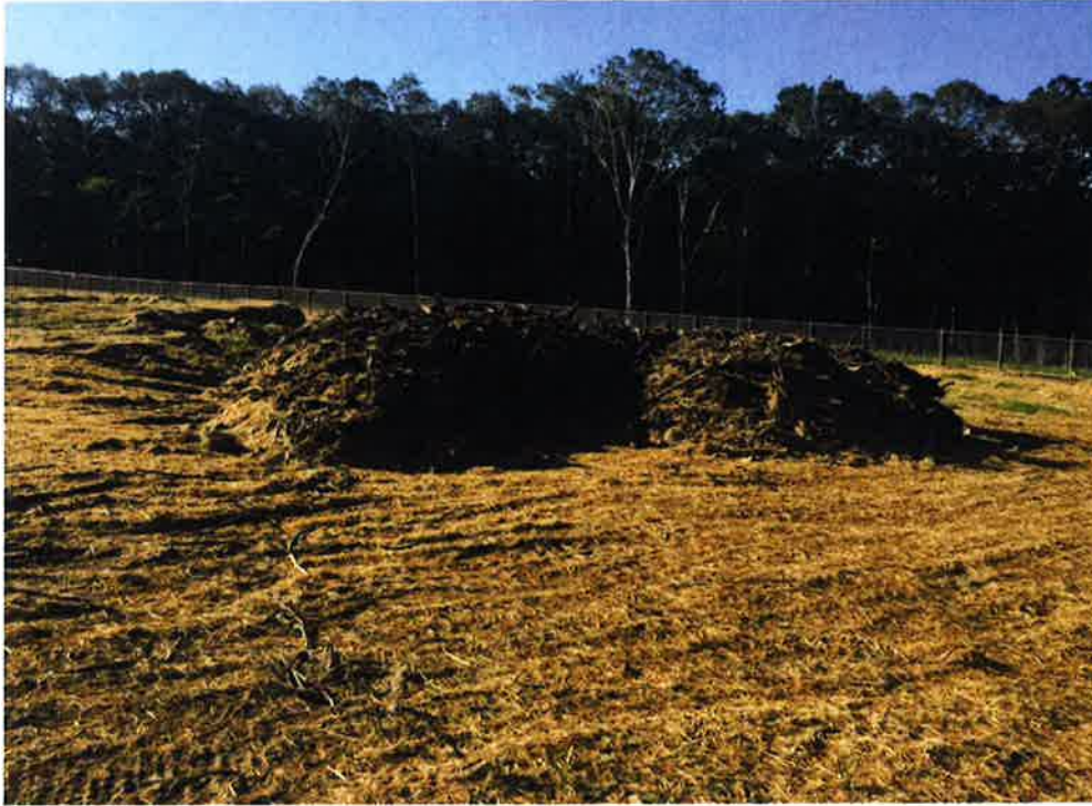
Photo 11: View of stockpile unprotected.
