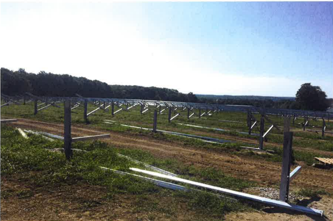
Photo 6: View of typical racking activities looking south.
