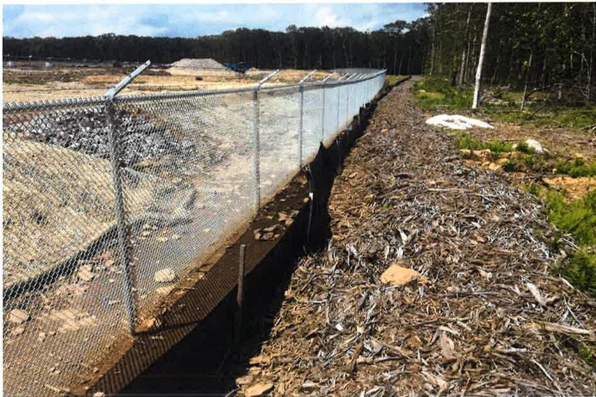
Photo 4: View of silt fence line repaired, looking north.
