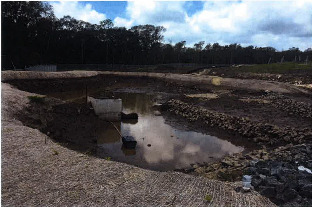
Photo 2: View of SB-3, looking west.
