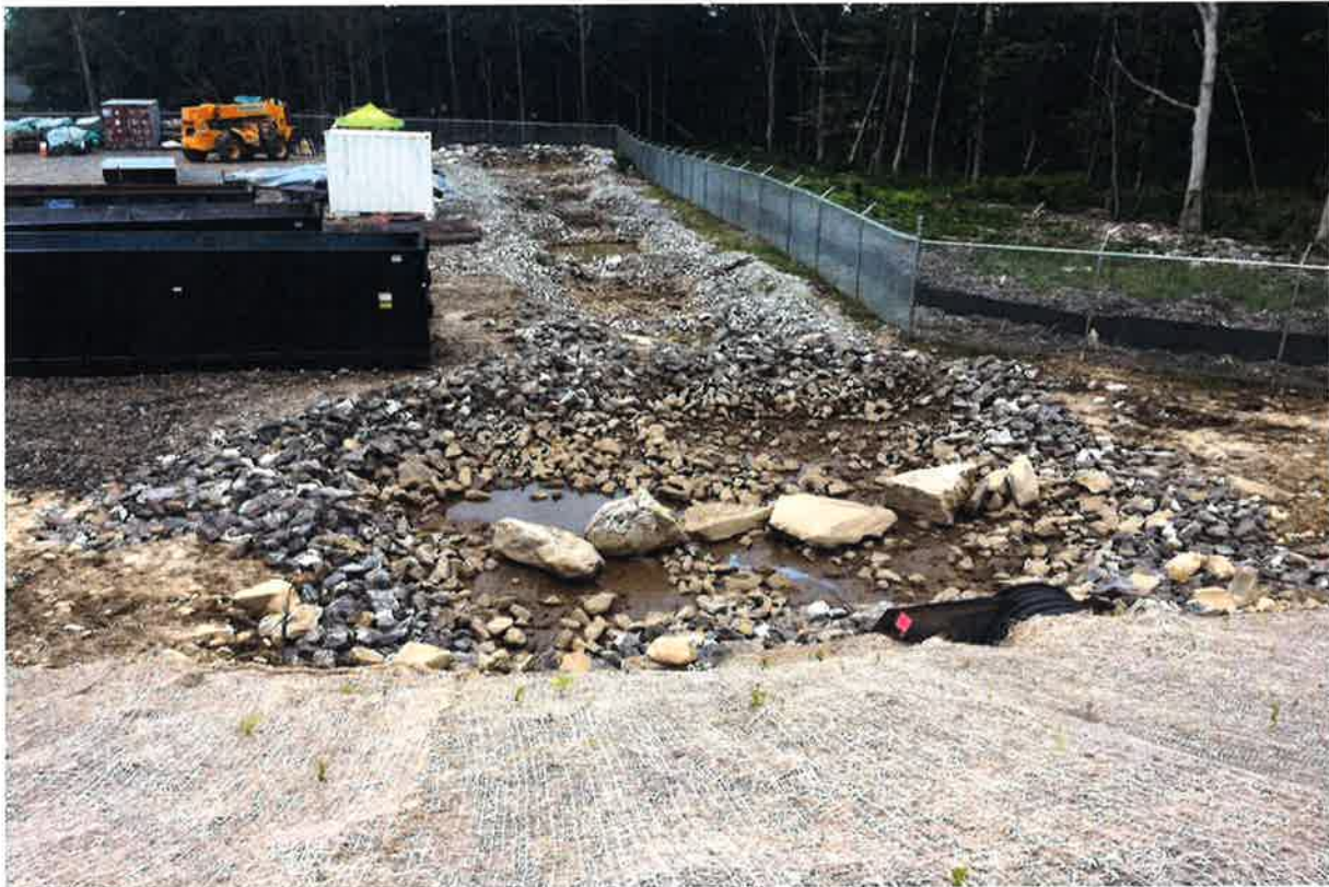
Photo 3: View of outlet from SB-3, looking south.
