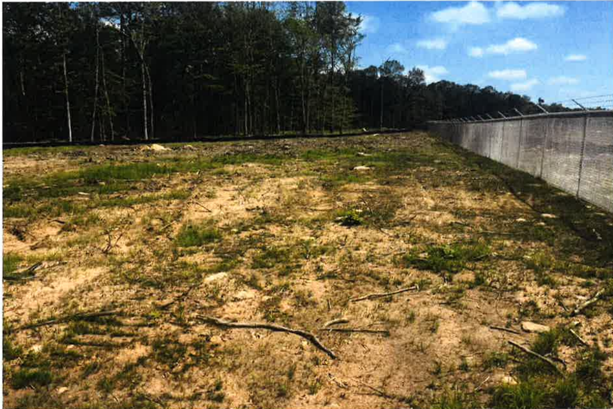
Photo 1: View of typical project perimeter looking north.
