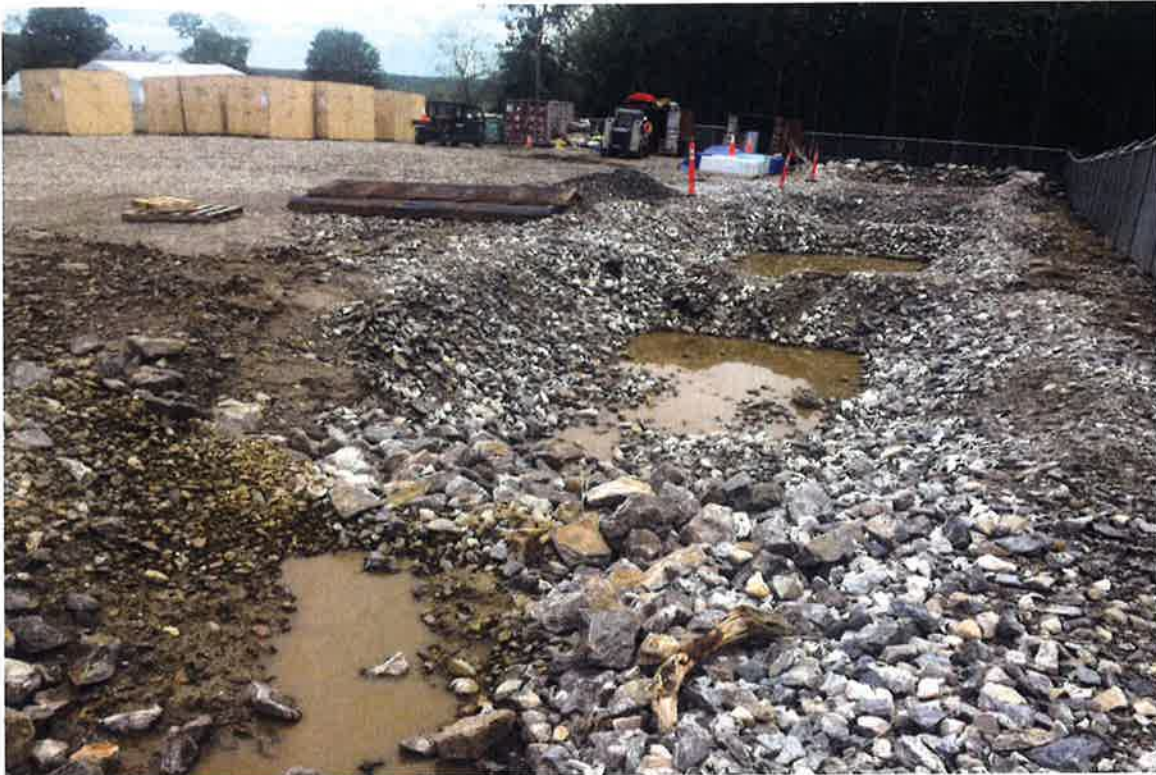
Photo 5: View of SB-3 outfall looking south.
