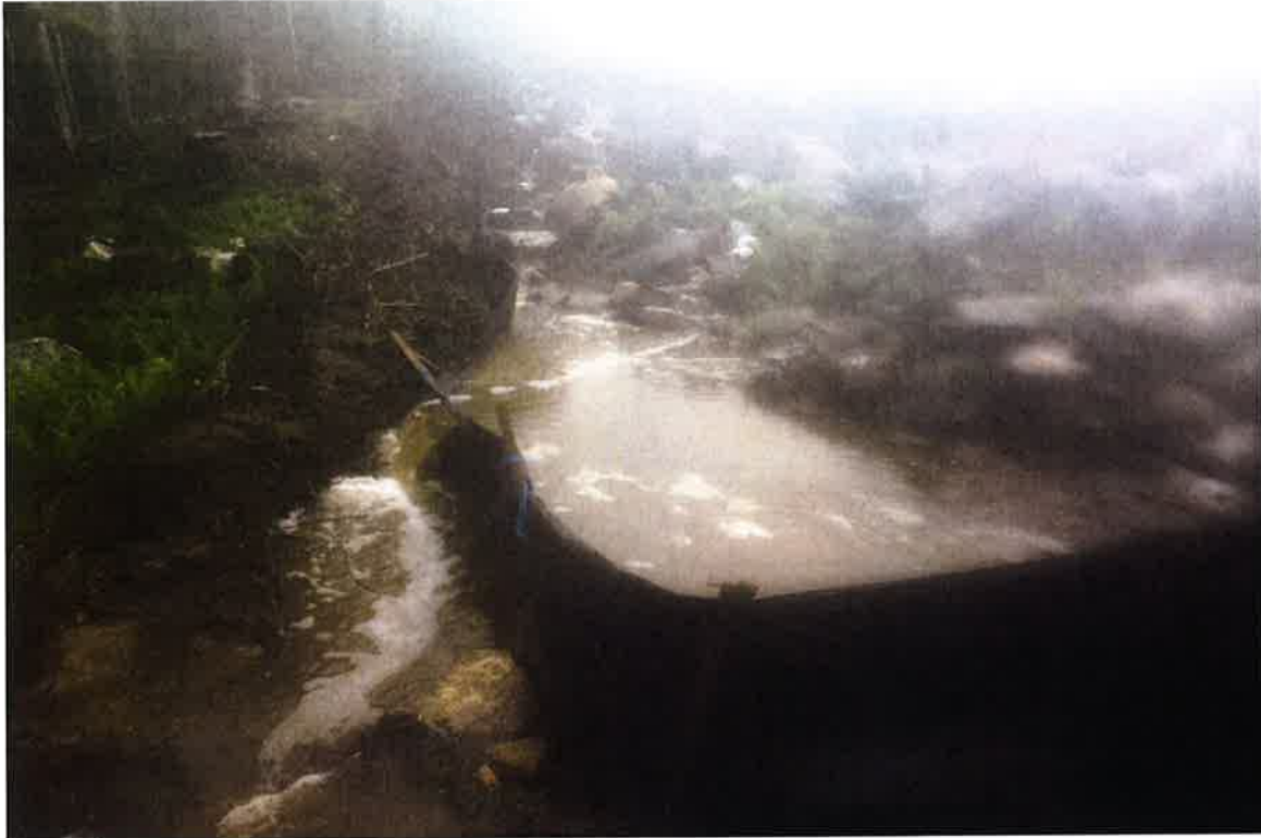
Photo 5: View of CA #8 with overtopping stormwater looking north.
