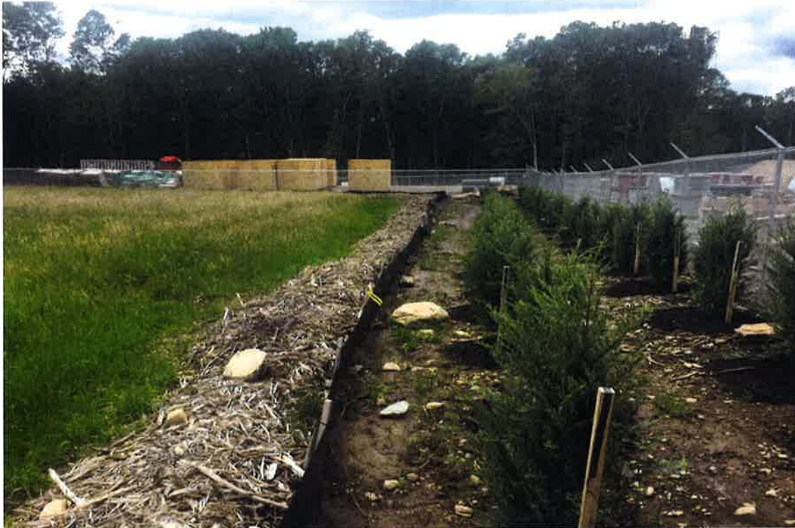
Photo 1: View of perimeter area south of laydown yard looking west.
