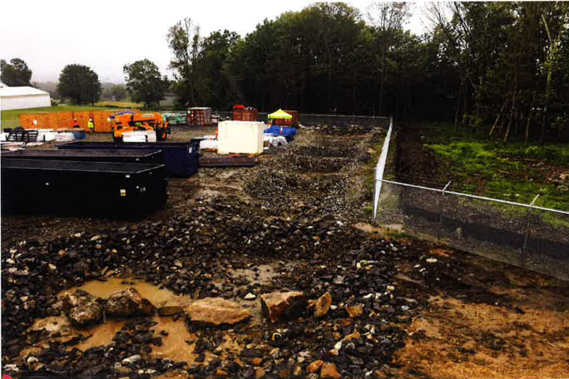
Photo 4: View of SB-3 outfall looking south.
