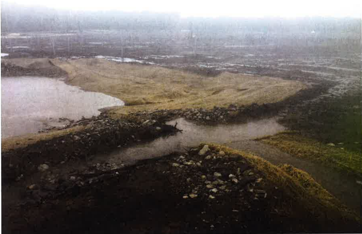
Photo 1: View of ST-7 (description of activity found in Report Notes) looking north.
