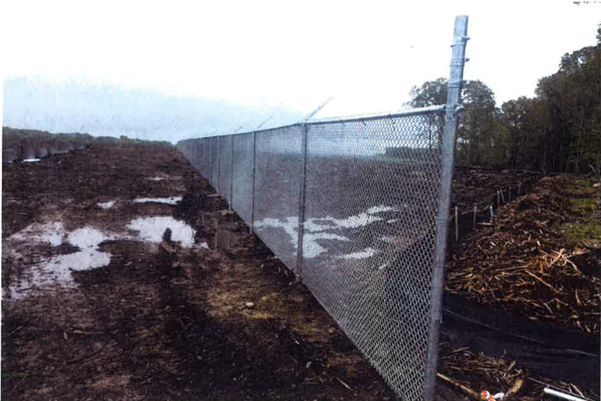
Photo 9: View of permanent fence installed looking south.
