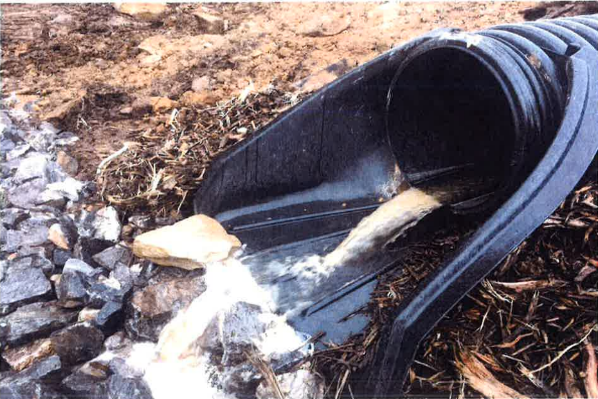
Photo 8: View of outlet from SB-3.
