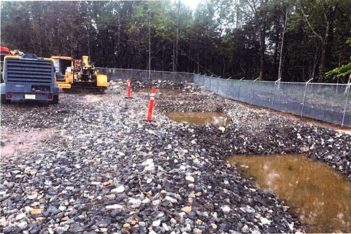
Photo 7: View of drainage swale from SB-3 looking south.
