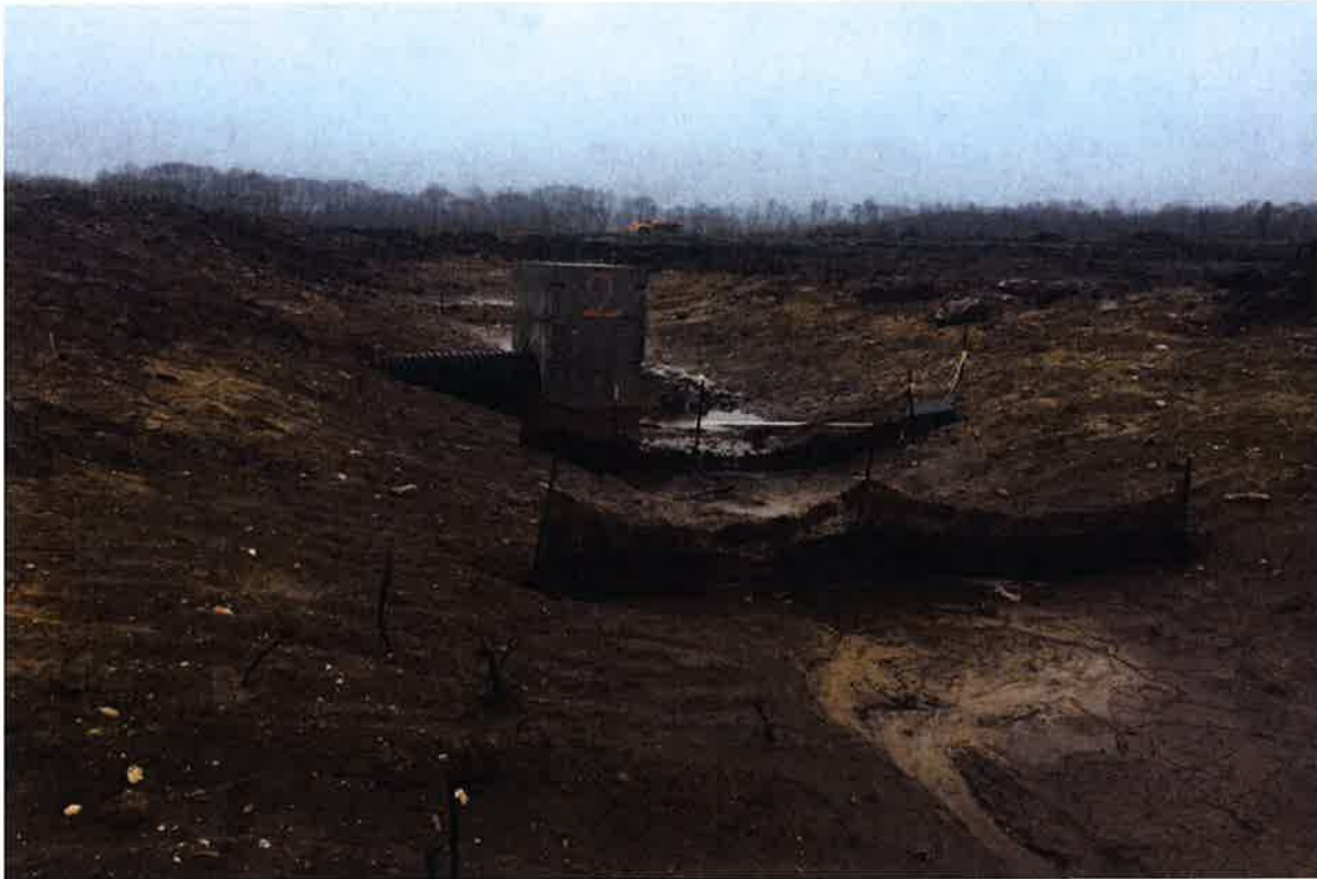
Photo 3: View of SB-2 functioning properly, looking west.
