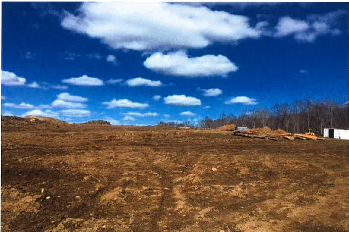
Photo 2: View of southeast project area looking north.
