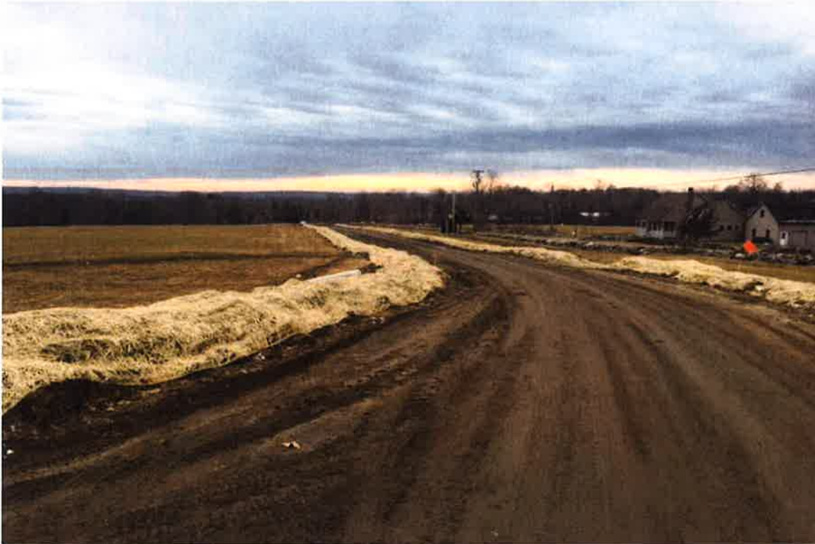
Photo 1: View of construction access looking south.
