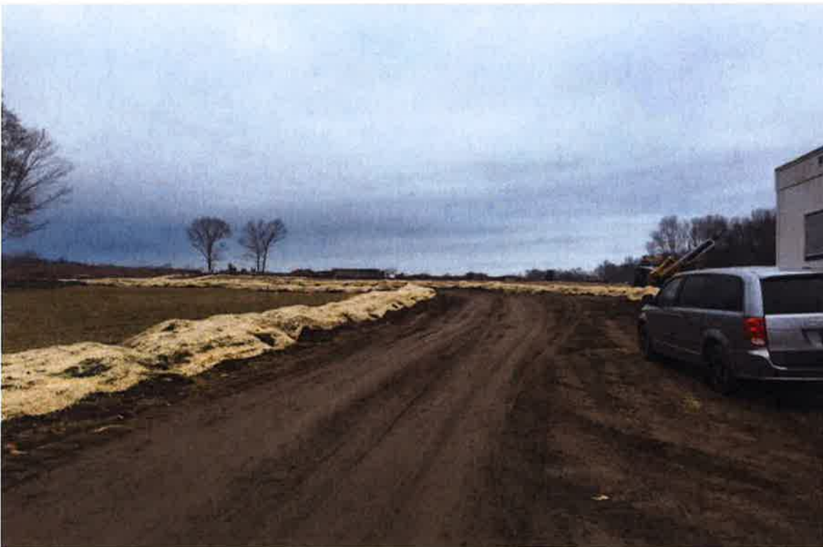
Photo 2: View north from construction trailer.
