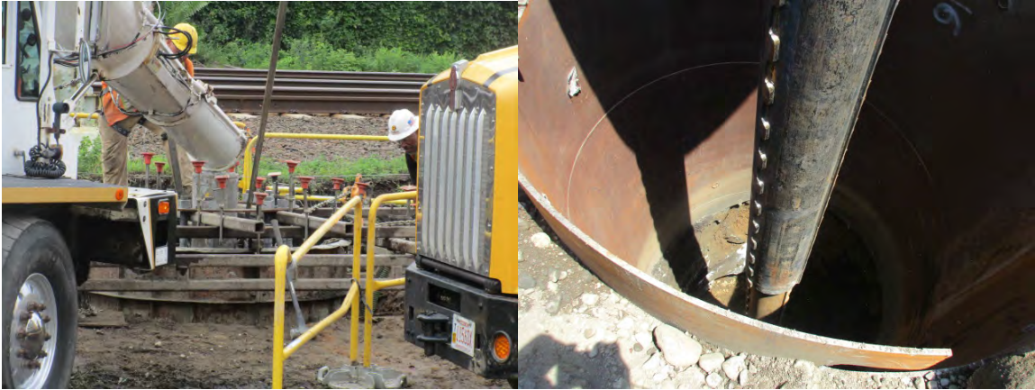
Pouring foundation 819N and drilling 788N
