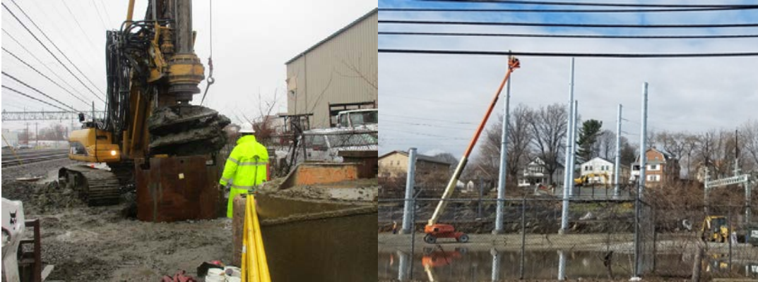
Drilling at 807N and structures 825AS through 825BS being set
