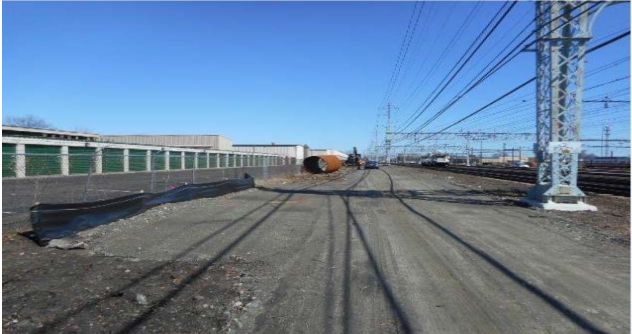
Access road and work area for Structure(s) 806N, 807N & 808N
