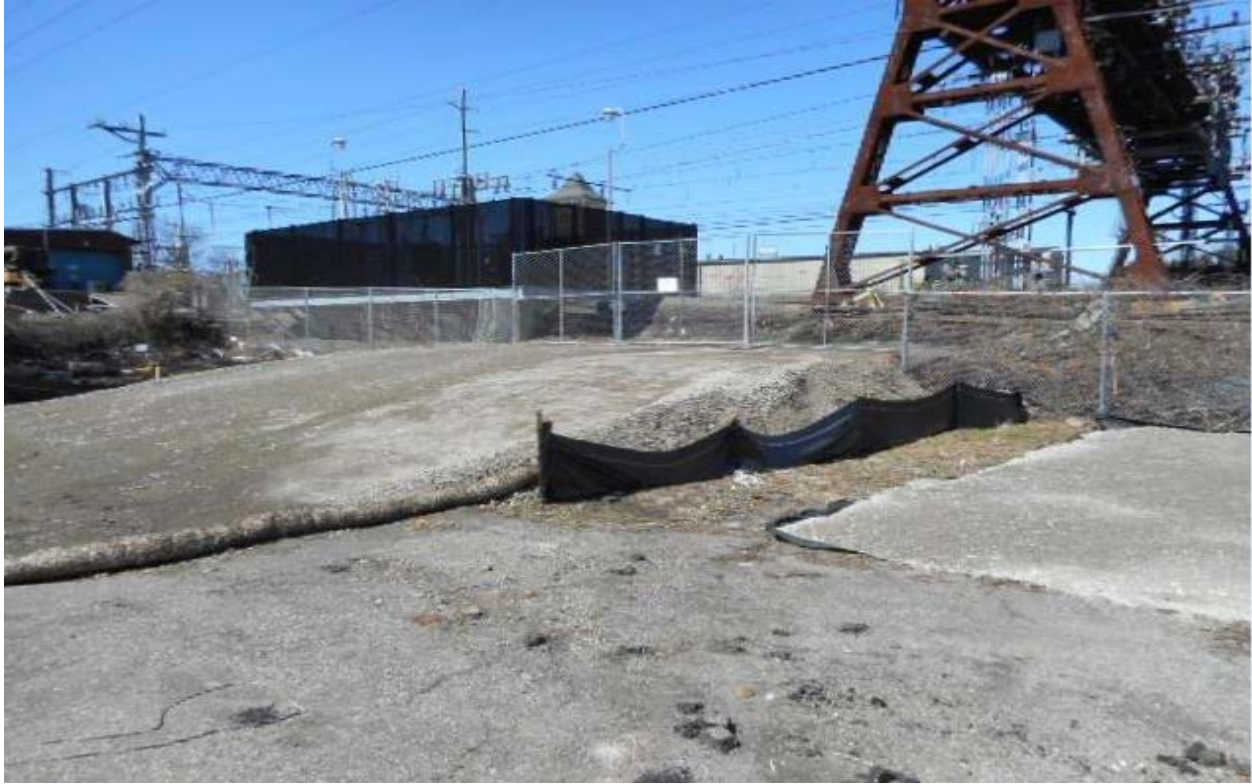
Access road and work pad for Structure 814S
