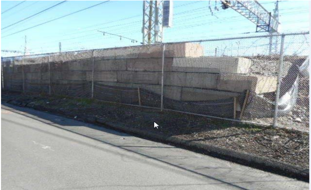
Retaining wall Structure 817N
