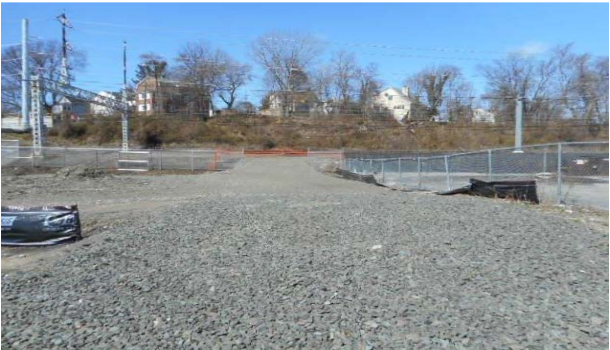
Access road for Structure(s) 823S, 824S & 825S
