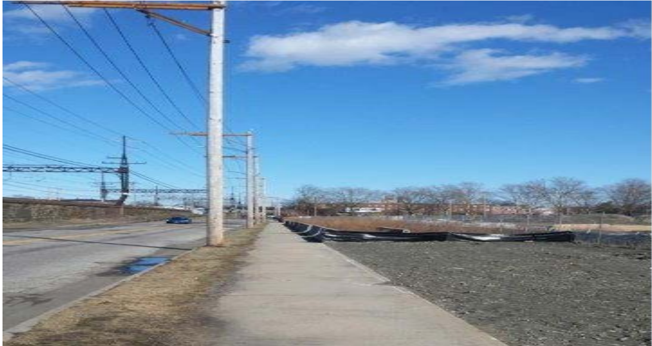
Work pad for Structure 797S
