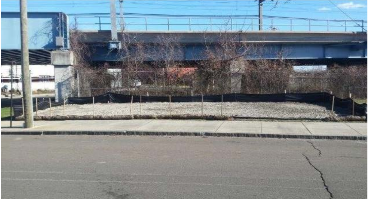
Work pad for Structure 786N
