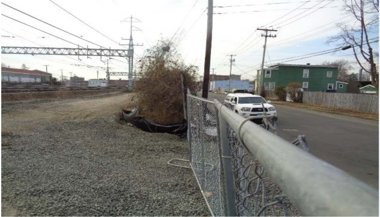
Construction entrance along with E&S controls for Structure(s) 816N, 817N & 818N
