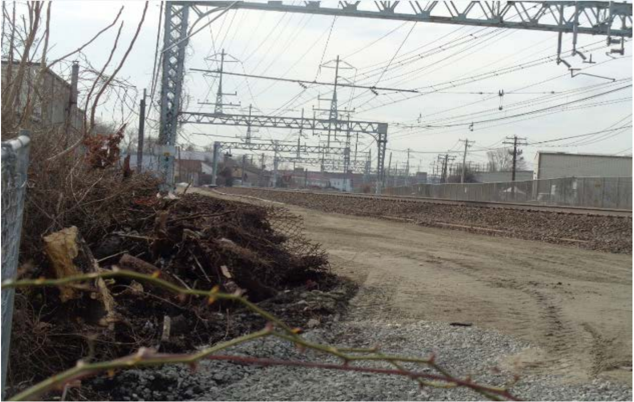
Access Road for Structure(s) 821S, 822S and 823S
