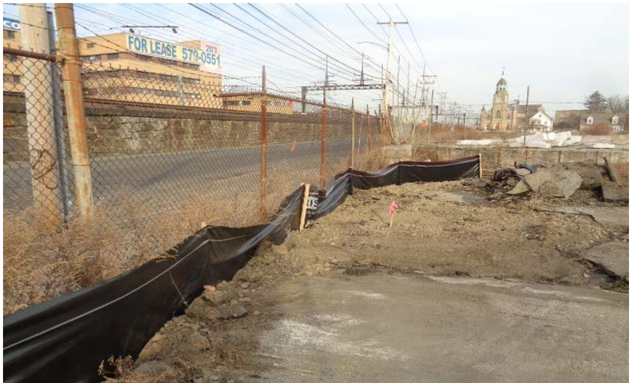
Work area at Structure 792S
