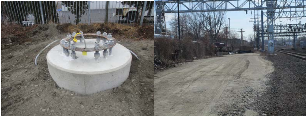
Finished foundation at 803S and access road from 809S to 811S
