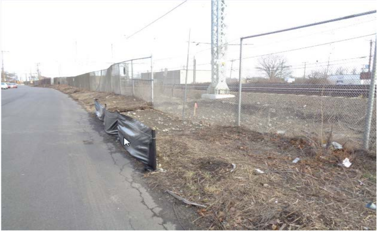
Silt fence for Structure 821N
