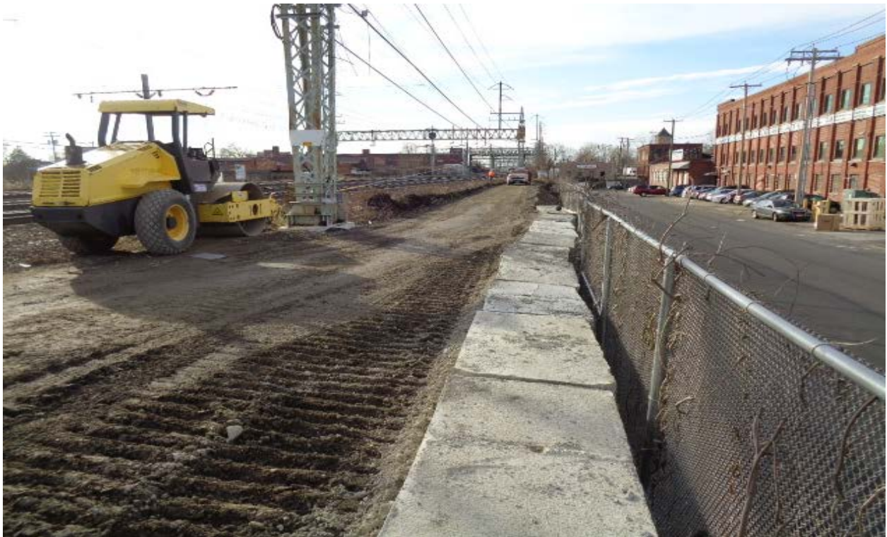
Access road to Structure(s) 216N, 817N and 818N
