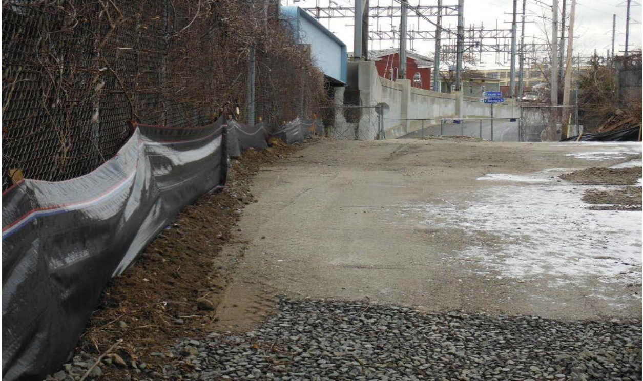
Tracking pad and access road to Structure 786S
