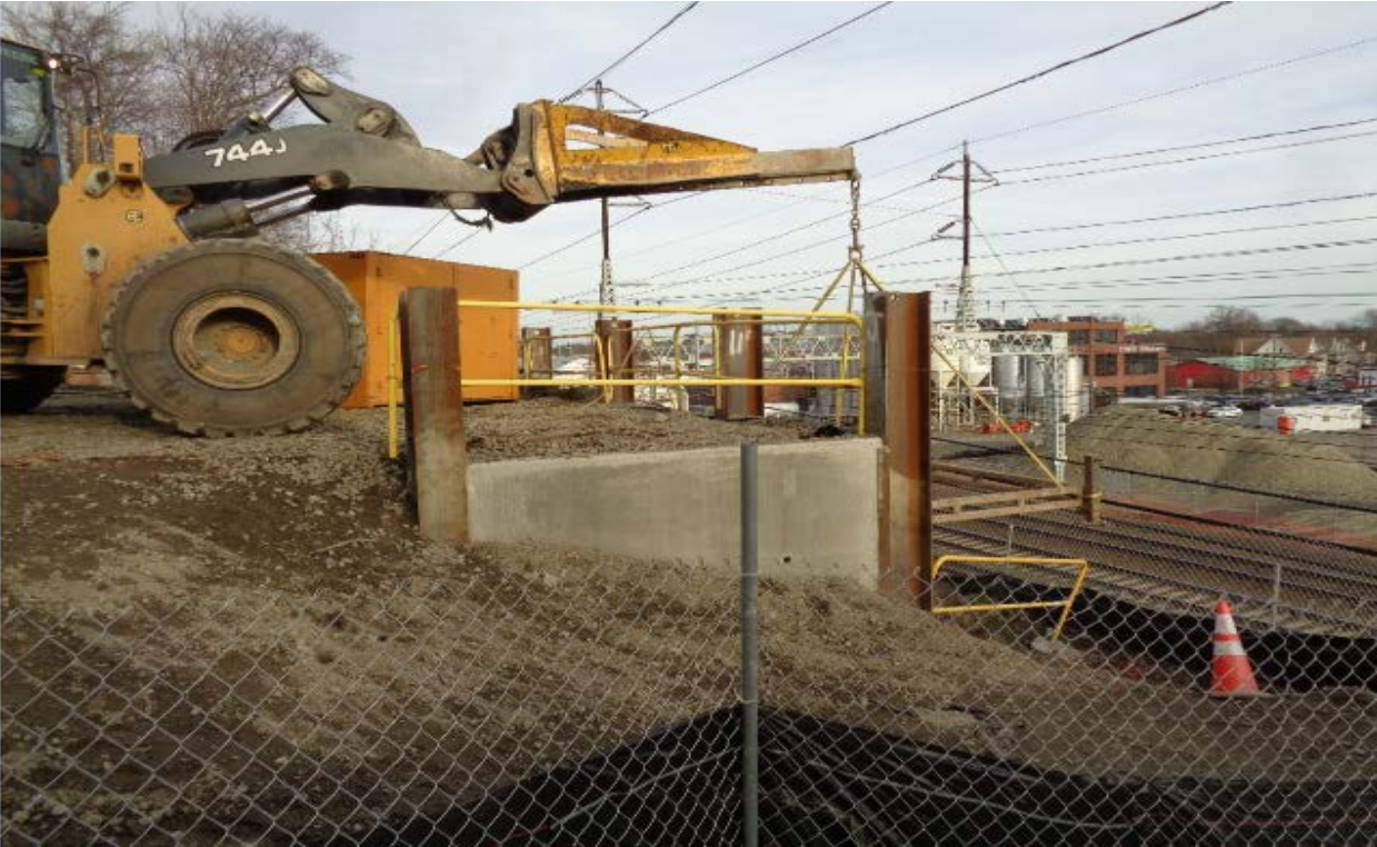
Building of work area for Structure 825N
