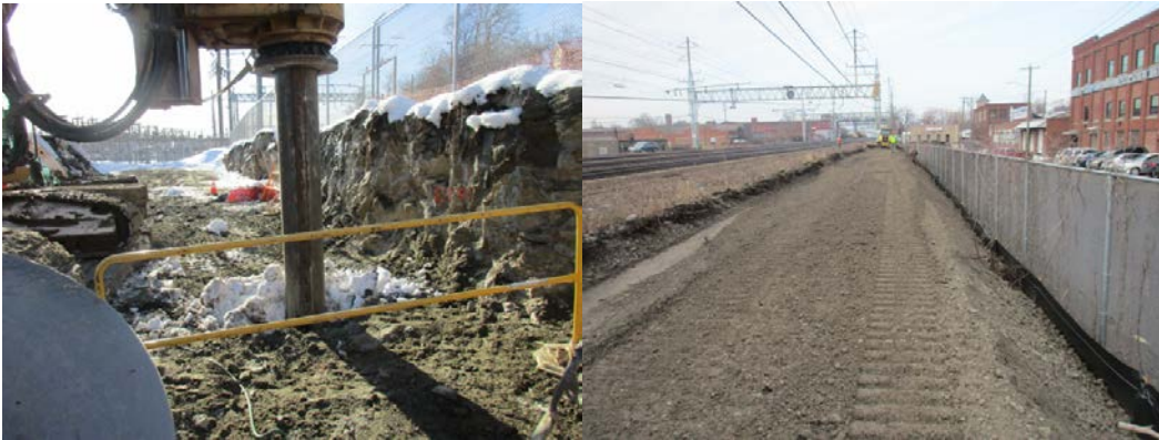
Drilling at 825BS and access road at 814N
