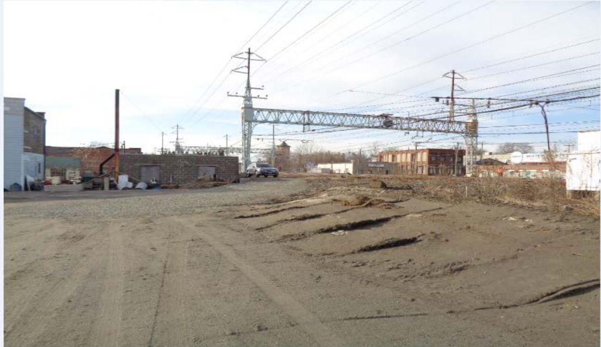
Grading and access road development at Structure(s) 816S, 817S and 818S
