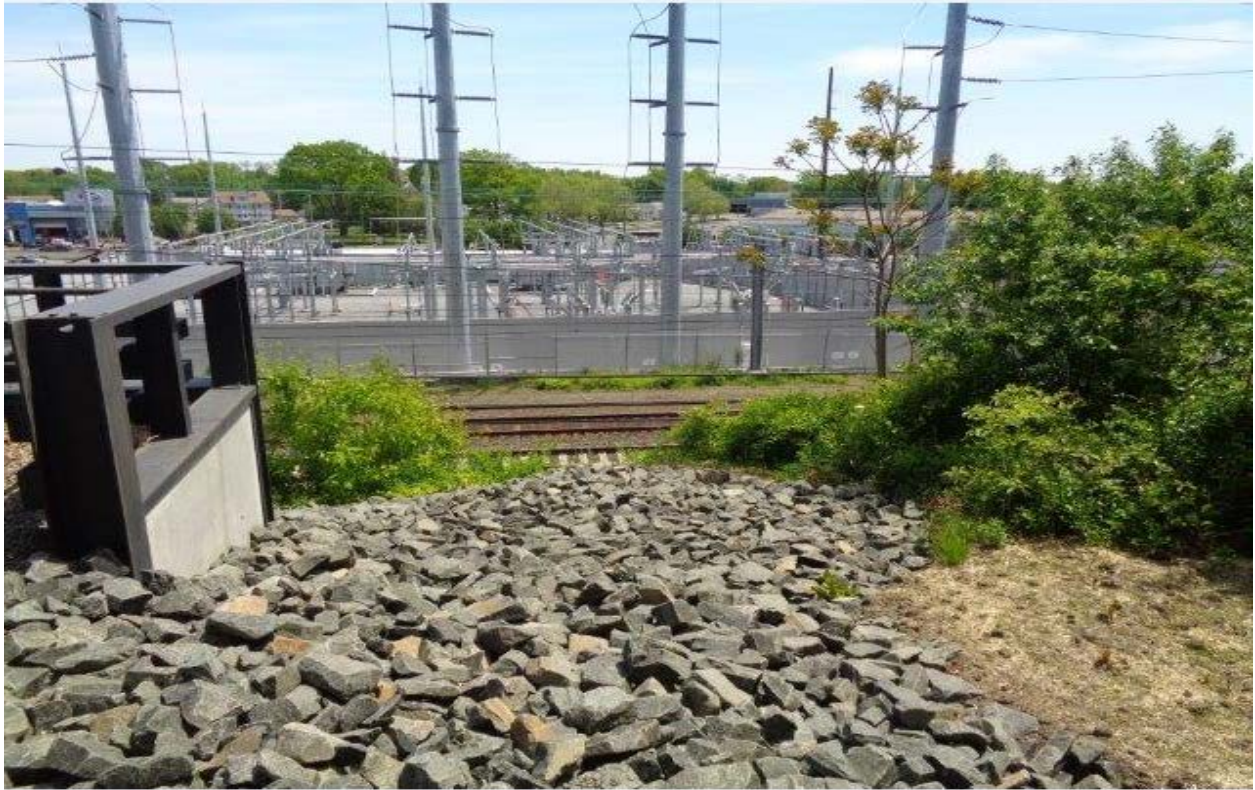
Swale north of New Baird Substation
