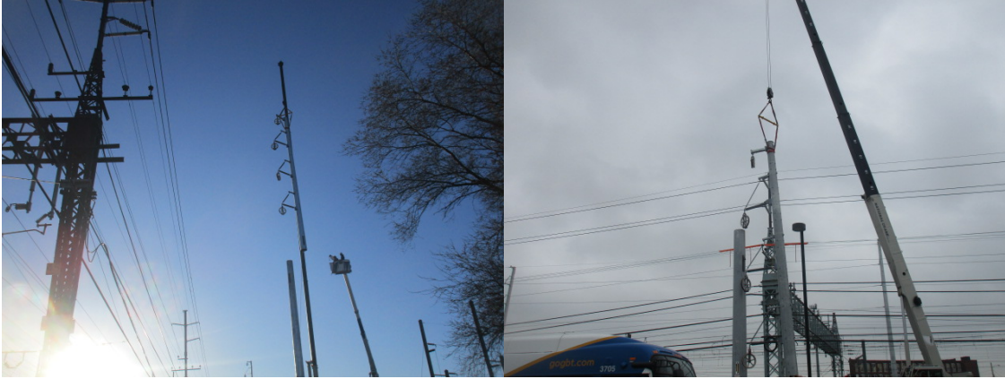
Setting structure 801N and structure 811N
