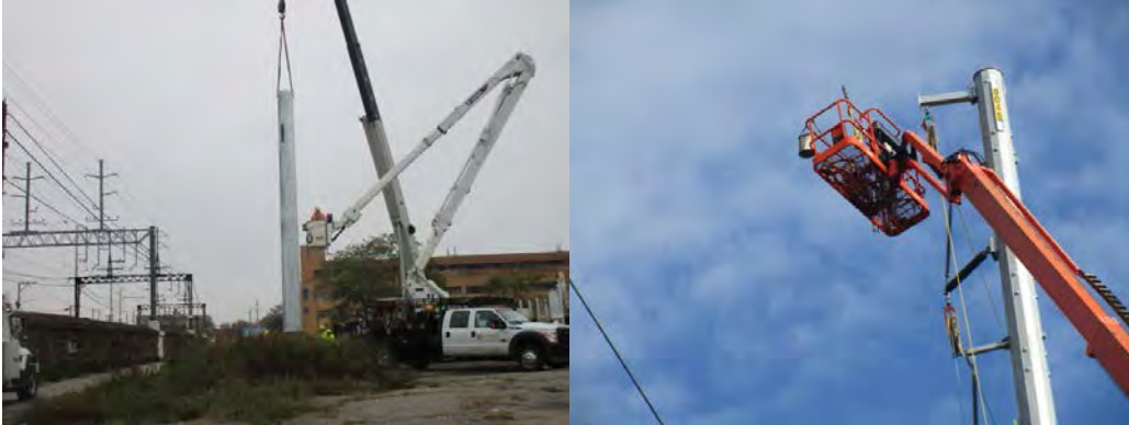
Setting structure 794N and installing ropes at structure 805S
